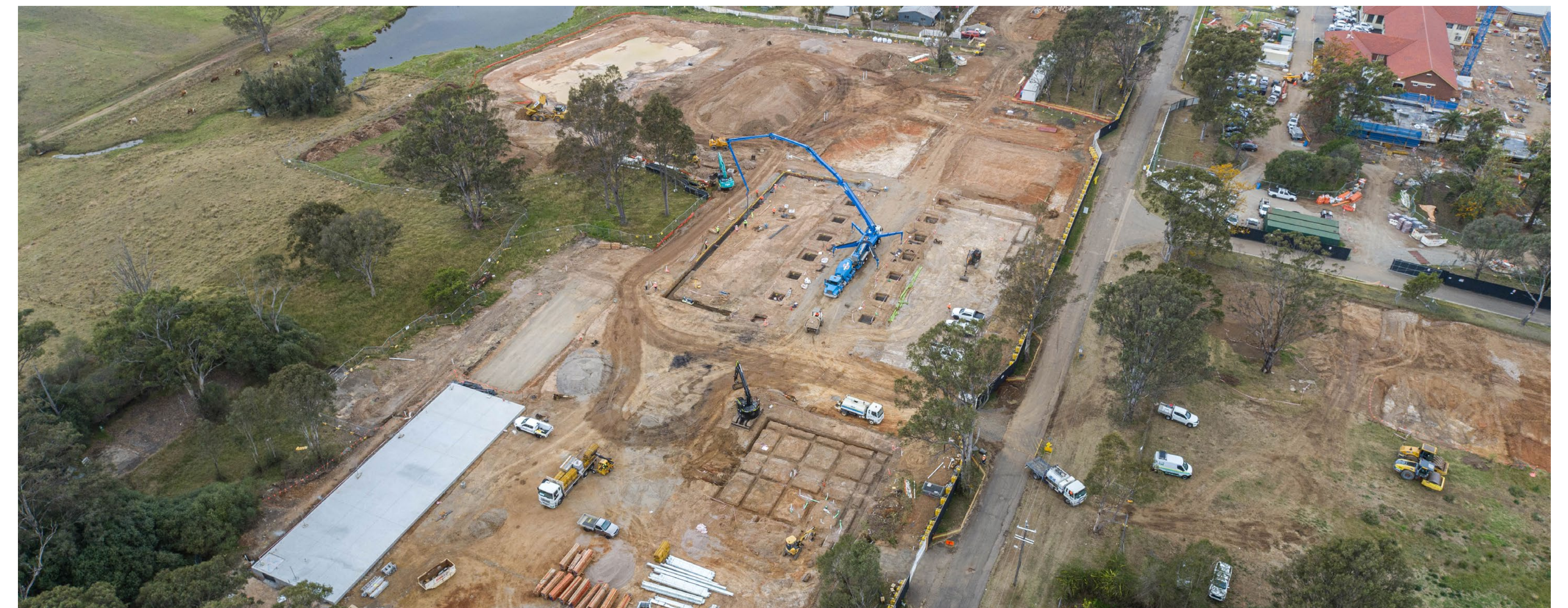
Construction of new farm buildings (Oct '23)
