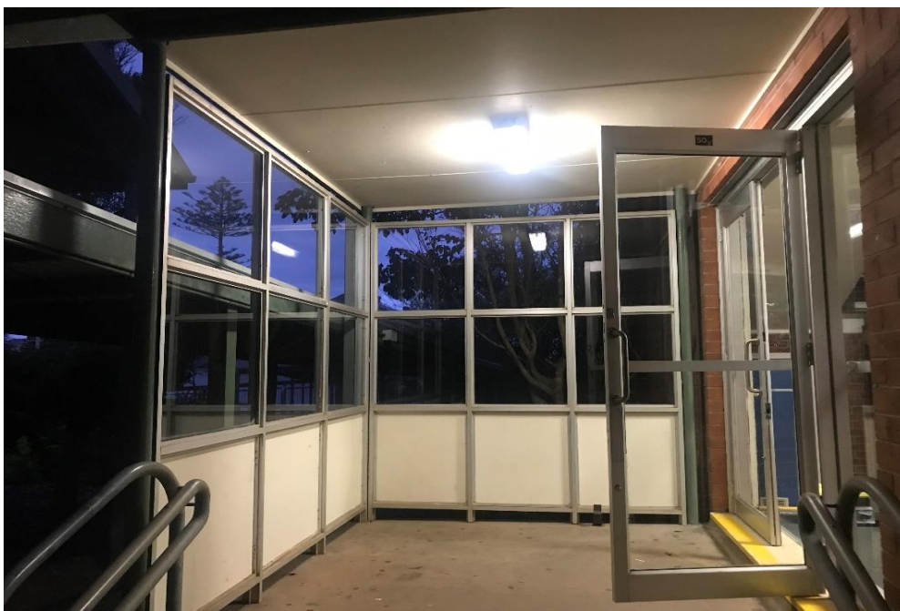
Photograph 1: B00B, BR0019, ceiling, fibre cement sheet, asbestos detected by analysis.
