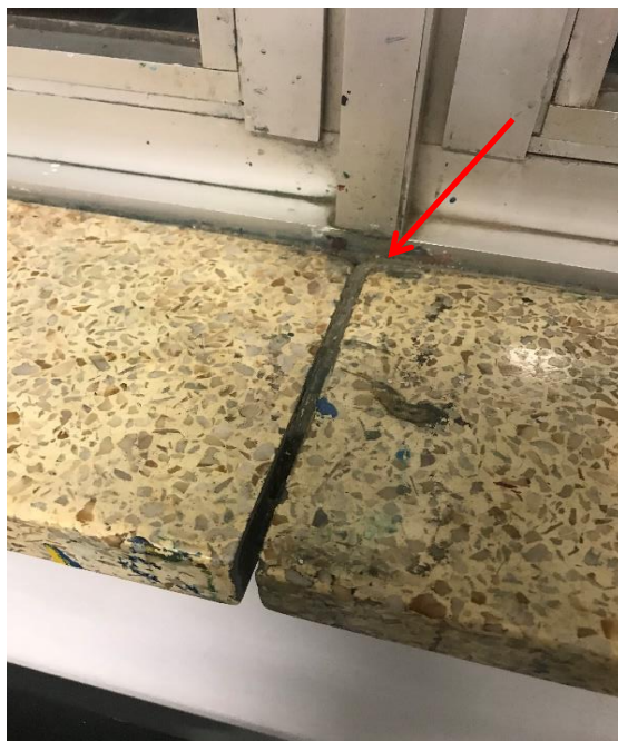
Photograph 5: Photograph shown is similar to B00B, BR0002, between window frame and terrazzo sill, putty, asbestos detected by analysis.
