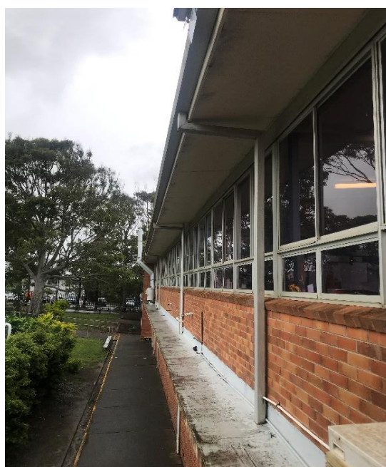
Photograph 4: B00B, exterior, eave linings generally, fibre cement sheeting, asbestos detected by analysis.
