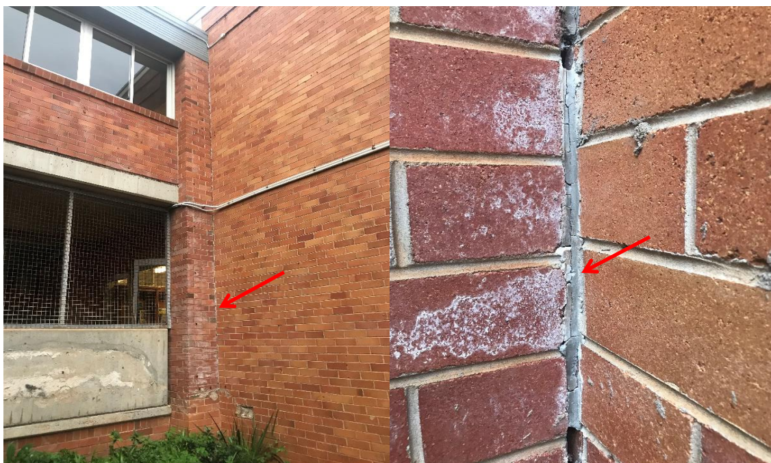
Photograph 11: B00B, BR0020 / BR1023, exterior brick wall, expansion gap, grey putty, asbestos detected by analysis.
