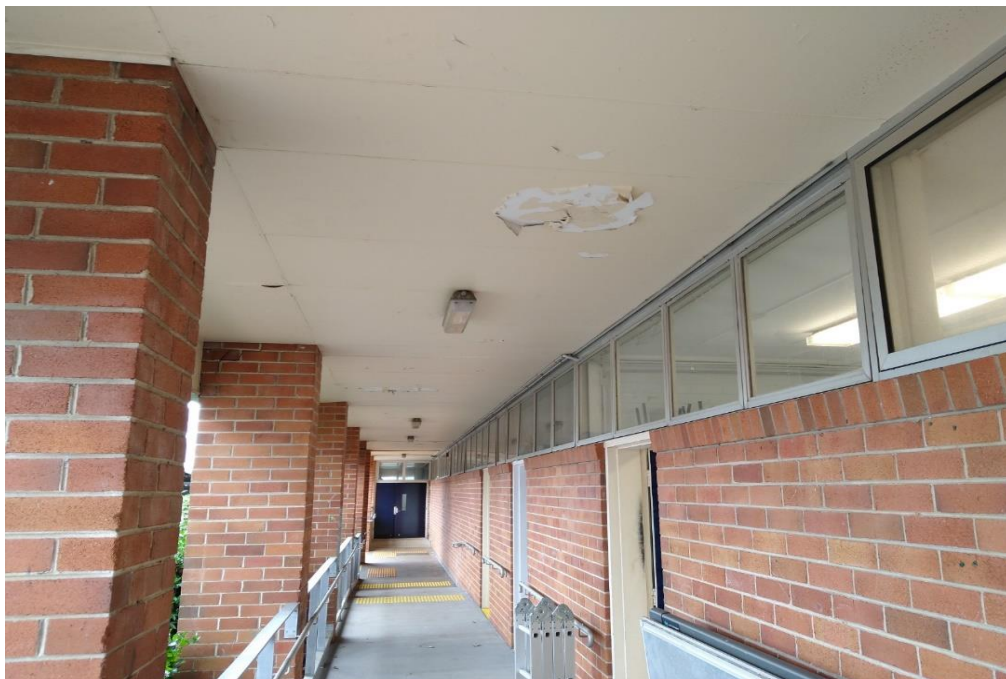
Photograph 2: B00T, R0016, ceiling, fibre cement, asbestos detected by analysis.
