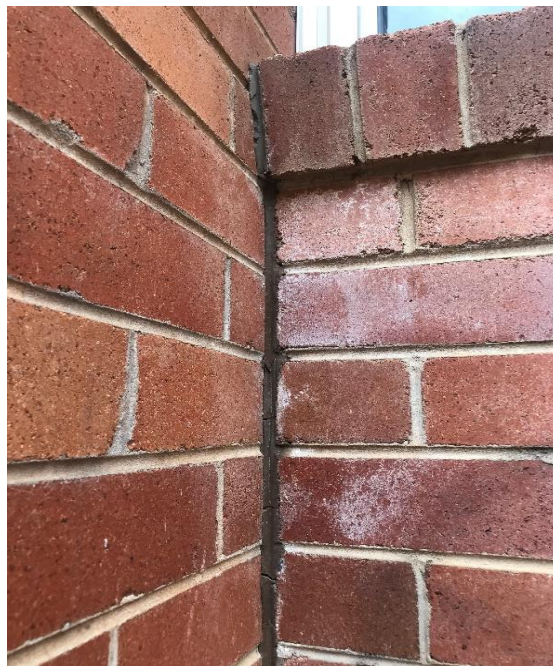
Photograph 2: B00L, exterior, western façade, between brick columns and walls, mastic, asbestos detected by analysis.
