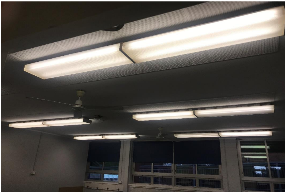
Photograph 22: B00L, rooms and areas in general, fluorescent light fittings in general, capacitors, insulating oil, PCB (assumed).
