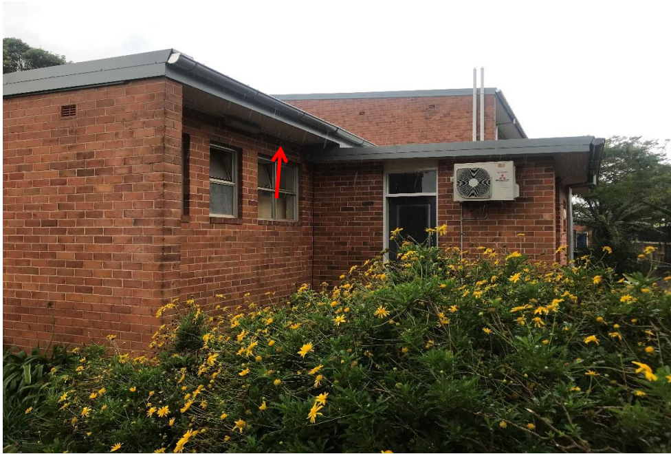
Photograph 17: B00A, exterior, fibre cement sheeting, upper eave south west corner, fibre cement, asbestos detected by analysis.
