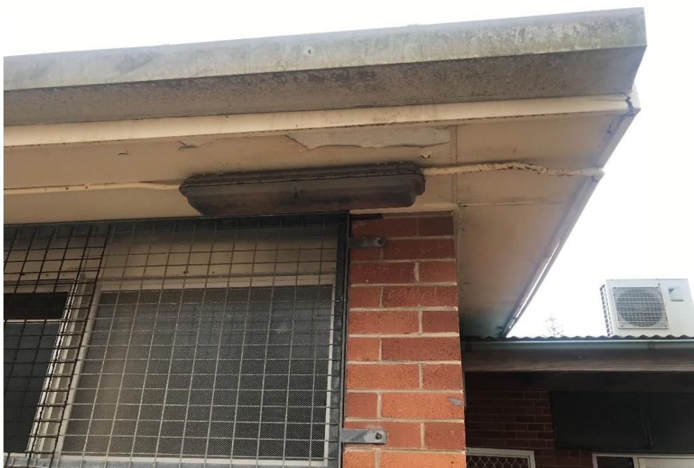
Photograph 12: B00C, rooms and areas in general, fluorescent light fittings in general, capacitors, insulating oil, PCB (assumed).
