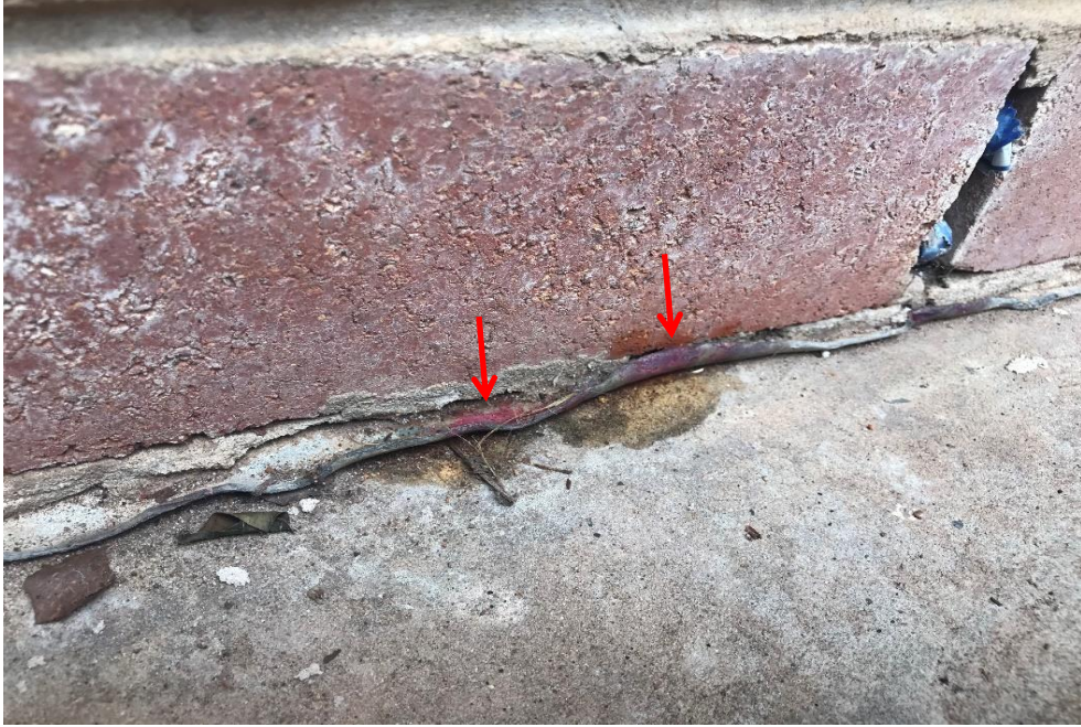
Photograph 23: B00L, exterior, western façade, northern end, typical flashing, positive for lead.
