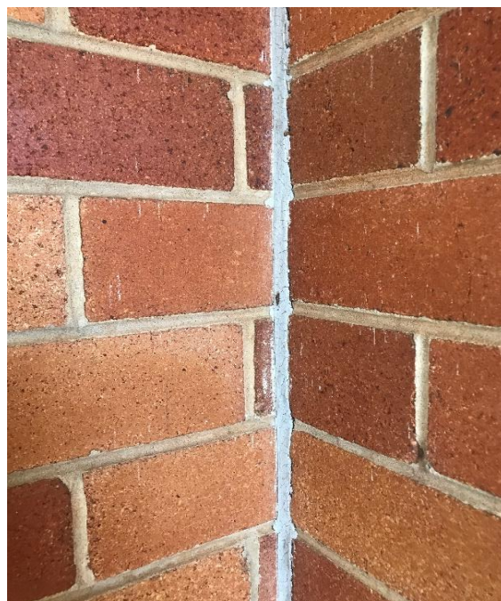
Photograph 9: B00A, AR0042, southeast corner, brick wall, expansion gap, joint mastic, asbestos detected by analysis.
