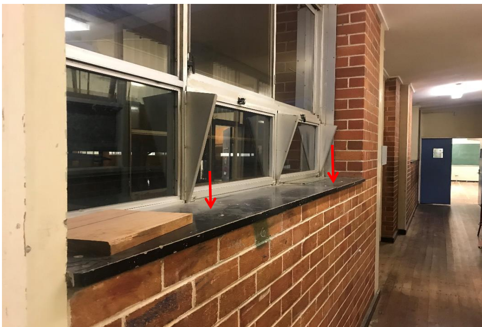
Photograph 1: BTAS, typical window sill lining(s), fibre cement, asbestos detected by analysis.
