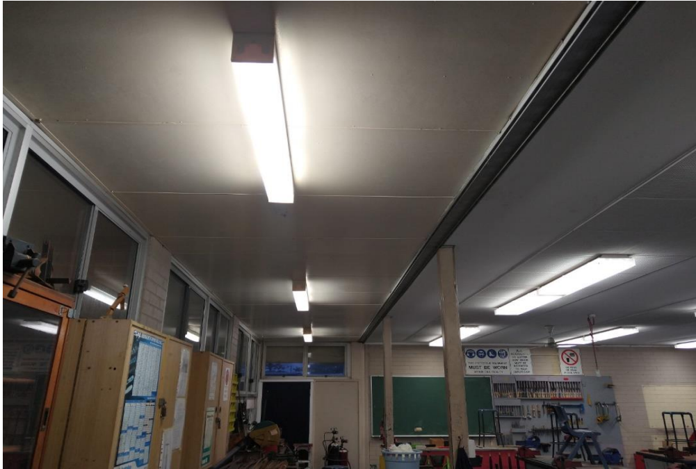
Photograph 7: B00T, R0014, ceiling panels along western side of room , fibre cement , asbestos detected by analysis.
