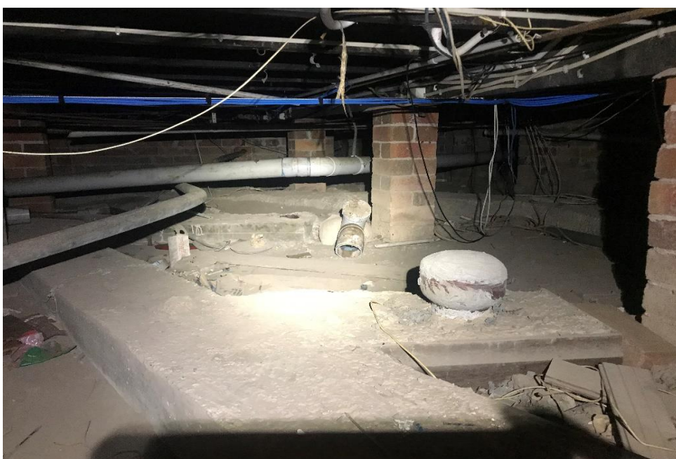
Photograph 3: B00A, AR0015, ceiling, vermiculite, no asbestos detected by analysis, SMF detected.
