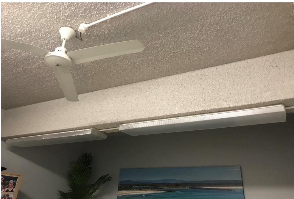
Photograph 1: B00A, rooms and areas in general, fluorescent light fittings in general, capacitors, insulating oil, PCB (assumed).
