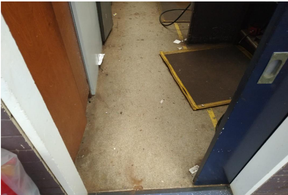
Photograph 10: B00T, R0006, flooring, vinyl flooring, asbestos detected by analysis.
