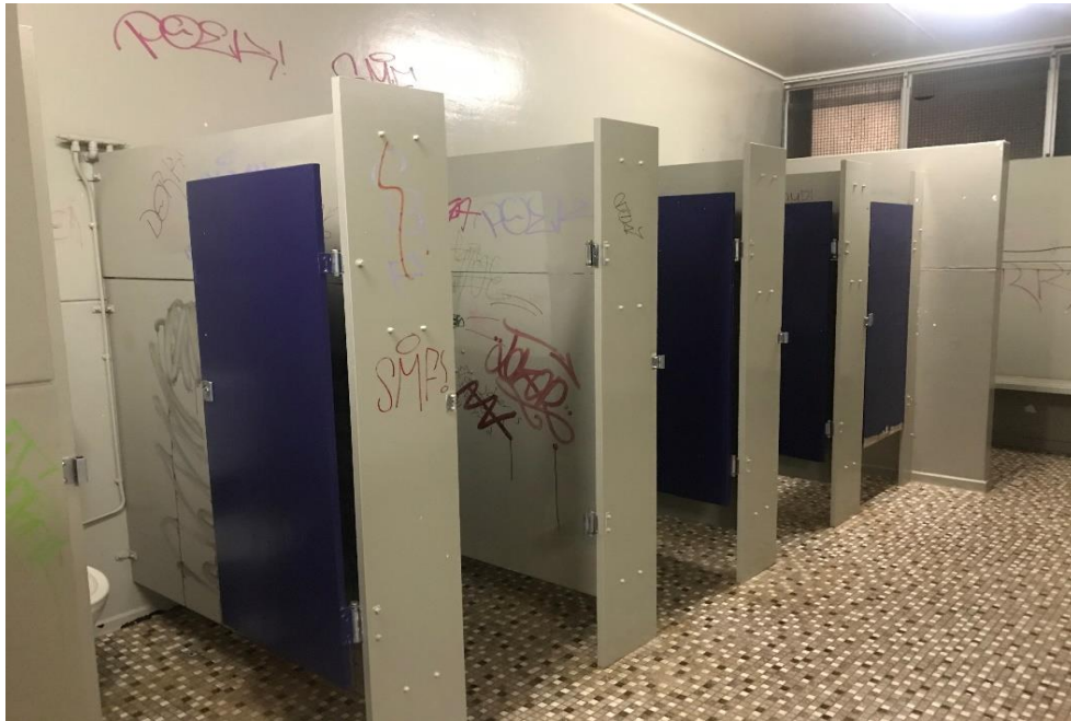
Photograph 7: B00C, CR0005, cubicles, partition walls, fibre cement board, asbestos detected by analysis.
