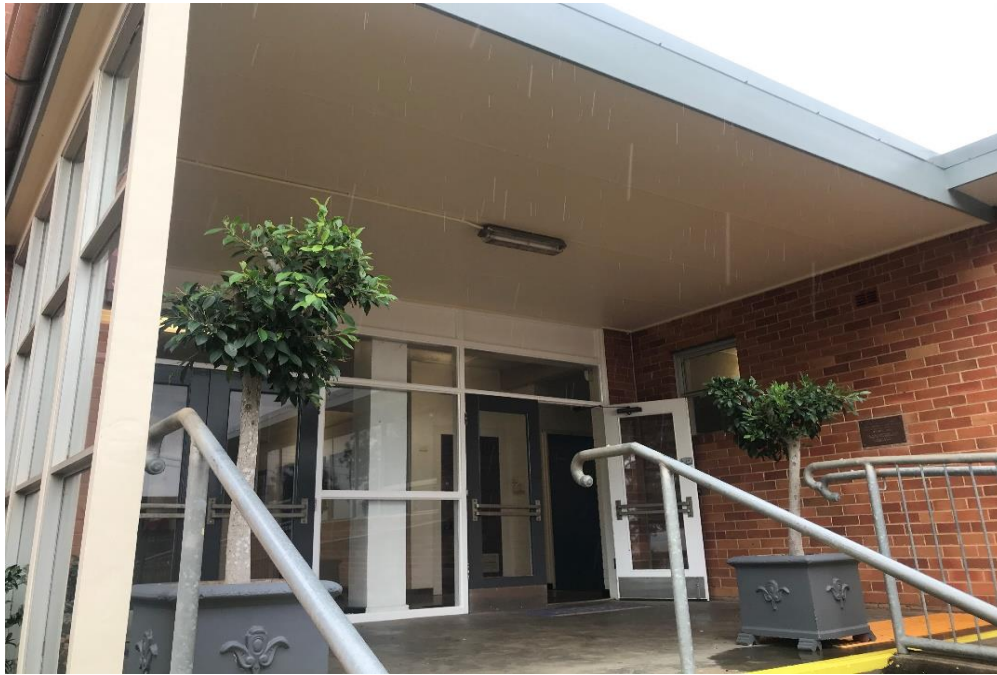
Photograph 7: B00A, AR0042, ceiling, fibre cement sheeting, asbestos detected by analysis.
