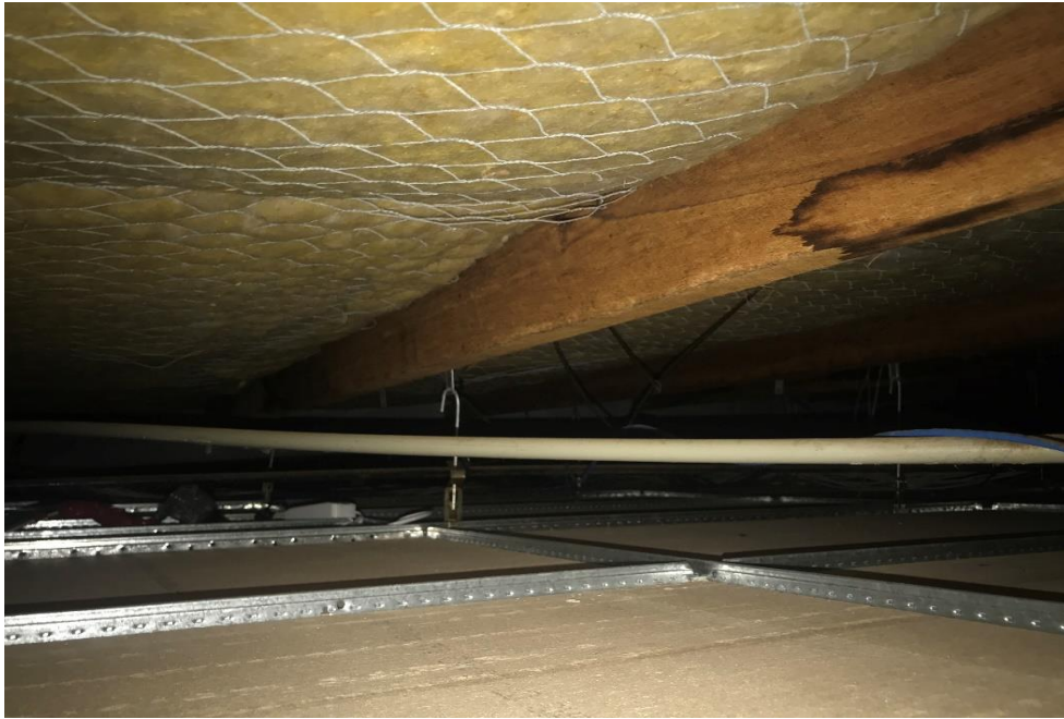
Photograph 17: B00L, LR1025, ceiling cavity, insulation to roof, SMF identified visually.
