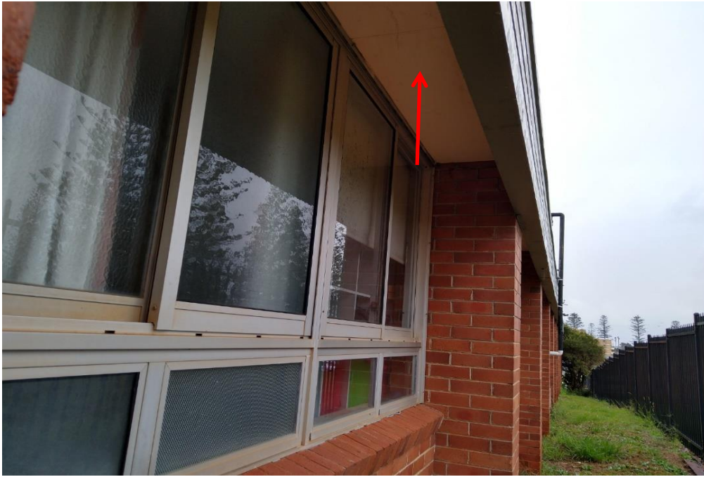
Photograph 3: B00T, exterior, eave lining (eastern aspect), fibre cement, asbestos detected by analysis.
