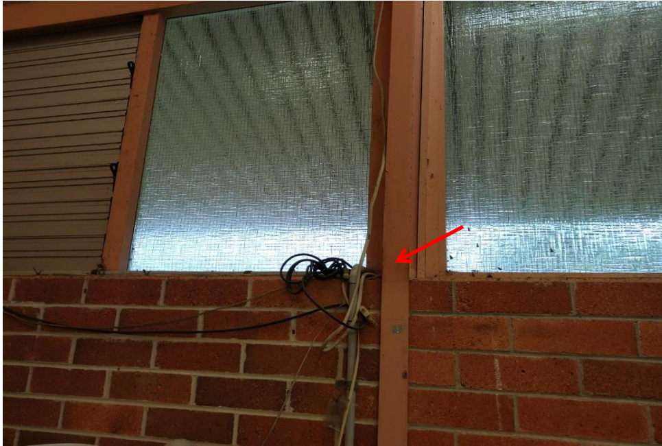
Photograph 3: BMPC, R0009, walls, pink paint , lead paint (>0.1% lead w/w).
