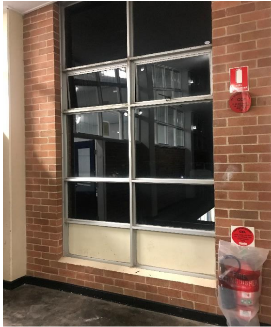
Photograph 11: B00A, first floor, room above AR0046, window frame, infill panels, asbestos (assumed).
