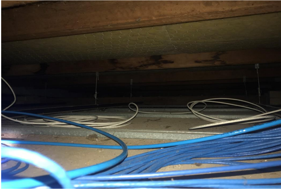
Photograph 21: B00L, LR1022, ceiling cavity, settled dust/debris, elevated lead ( \geq 0.5 \text{ mg/m}^2 ).
