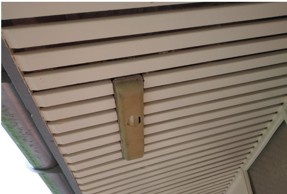
Photograph 4: BMPC, fluorescent lights, nil PCB assumed based on building construction date (circa 1985).
