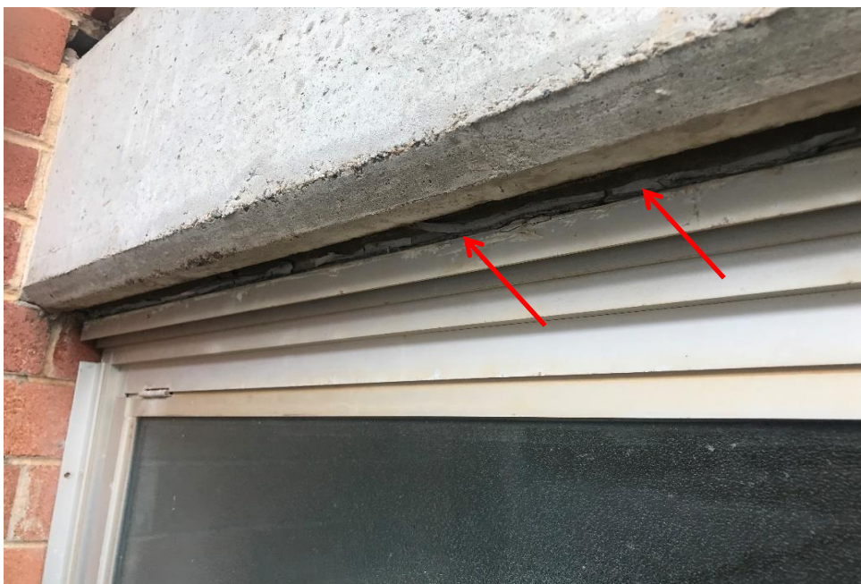
Photograph 3: B00L, exterior, western façade, north end, between window frame and wall, mastic, asbestos detected by analysis.
