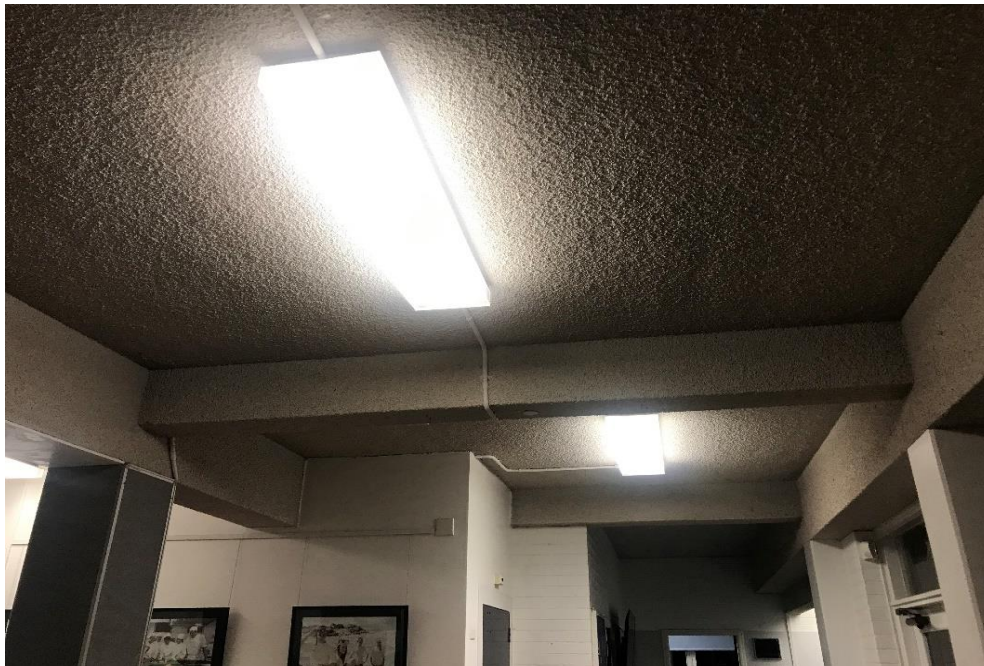
Photograph 6: B00A, AR0022, ceiling, eastern end of room, vermiculite, no asbestos detected by analysis, SMF detected.
