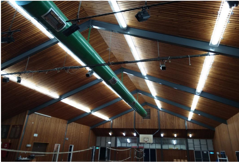
Photograph 7: BMPC, R0005, ceiling, air handling duct work, green paint, lead paint (assumed).
