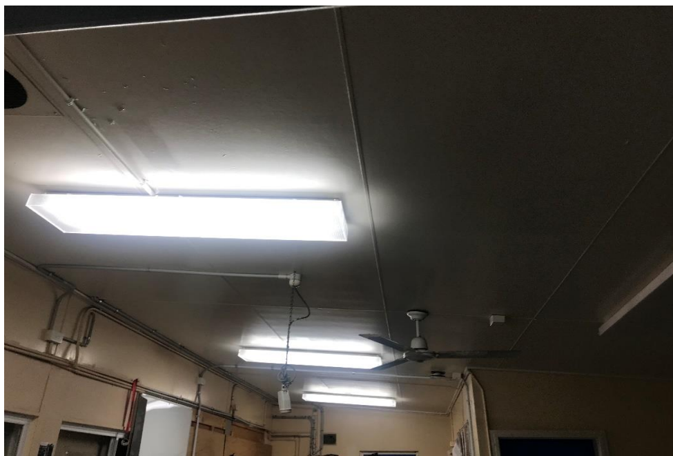
Photograph 4: B00C, CR0001, ceiling, fibre cement sheeting, asbestos detected by analysis.
