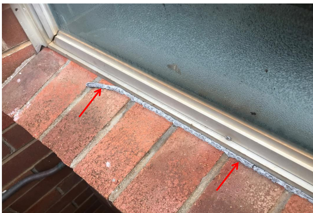
Photograph 4: B00L, exterior, western façade, centre, between window frame and wall, mastic, asbestos detected by analysis.
