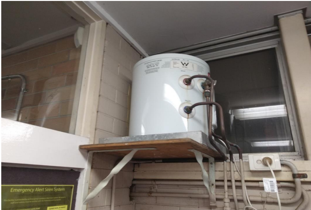
Photograph 9: B00T, R0014, hot water heater, insulation, SMF identified visually.
