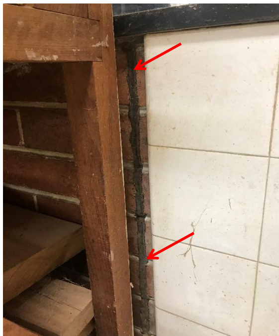
Photograph 7: BTAS, TAS-R0018, brick wall, expansion joint, mastic/sealant, asbestos detected by analysis.
