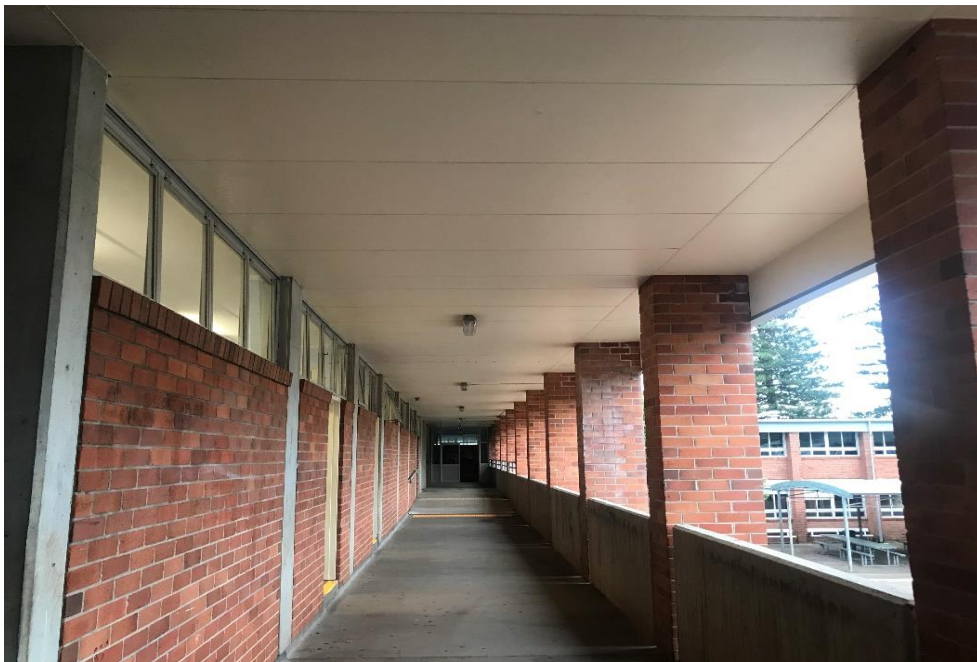
Photograph 20: B00L, LR1036, ceiling, fibre cement sheeting, asbestos detected by analysis.
