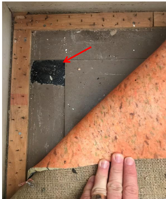
Photograph 12: Typical bituminous adhesive below vinyl tiles with white streaks, asbestos detected by analysis.
