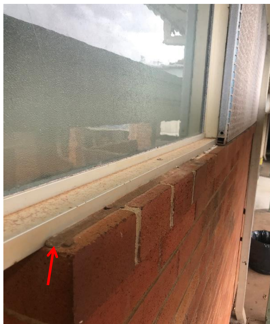
Photograph 2: B00C, exterior, northern façade, window frame, between window frame and wall, typical putty, asbestos detected by analysis.
