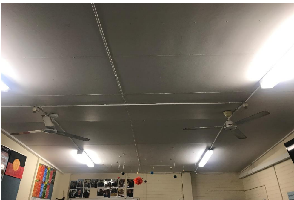
Photograph 6: B00C, CR0016, ceiling, fibre cement sheeting, asbestos detected by analysis.
