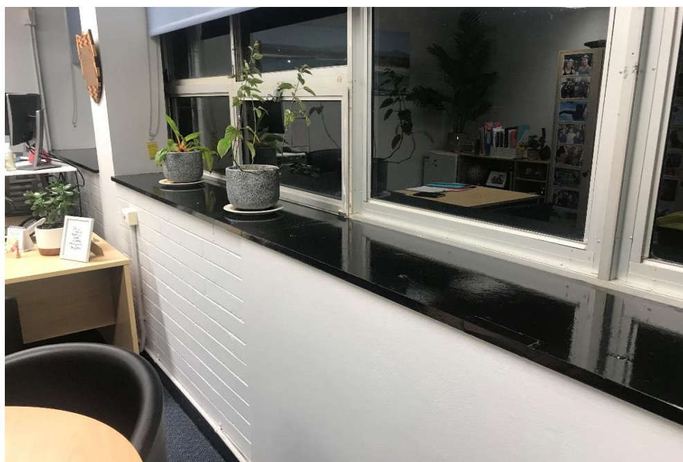
Photograph 2: B00A, AR0015, window sill, fibre cement board, asbestos detected by analysis.
