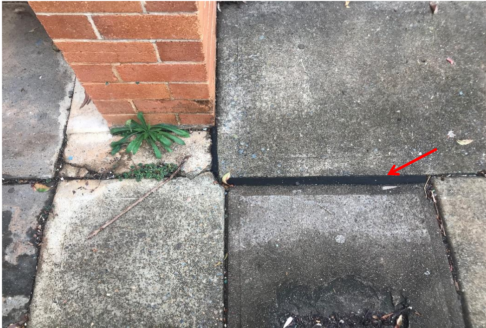
Photograph 13: B00A, exterior, exterior, northwest of building (near AR0024), expansion gap in paving, bitumastic, no asbestos detected by analysis, SMF detected.
