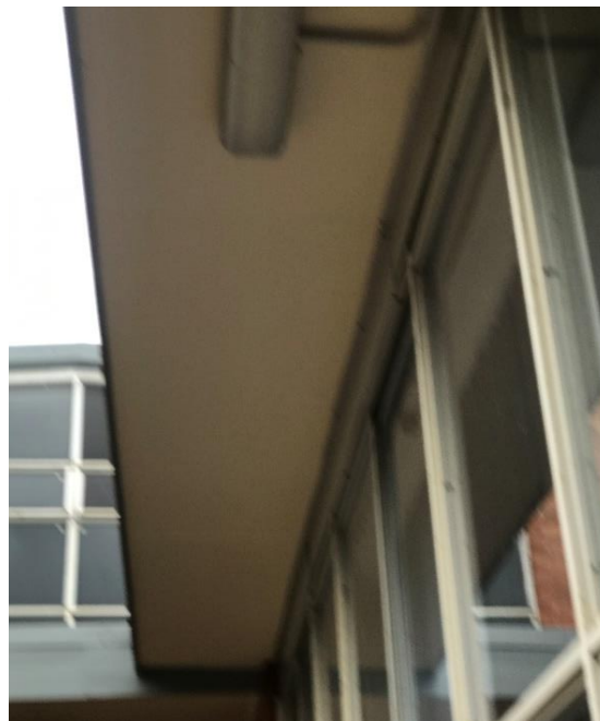
Photograph 16: B00A, exterior, eave lining adjacent wheelchair ramp (north of AR0019 and AR0020), fibre cement, asbestos detected by analysis.
