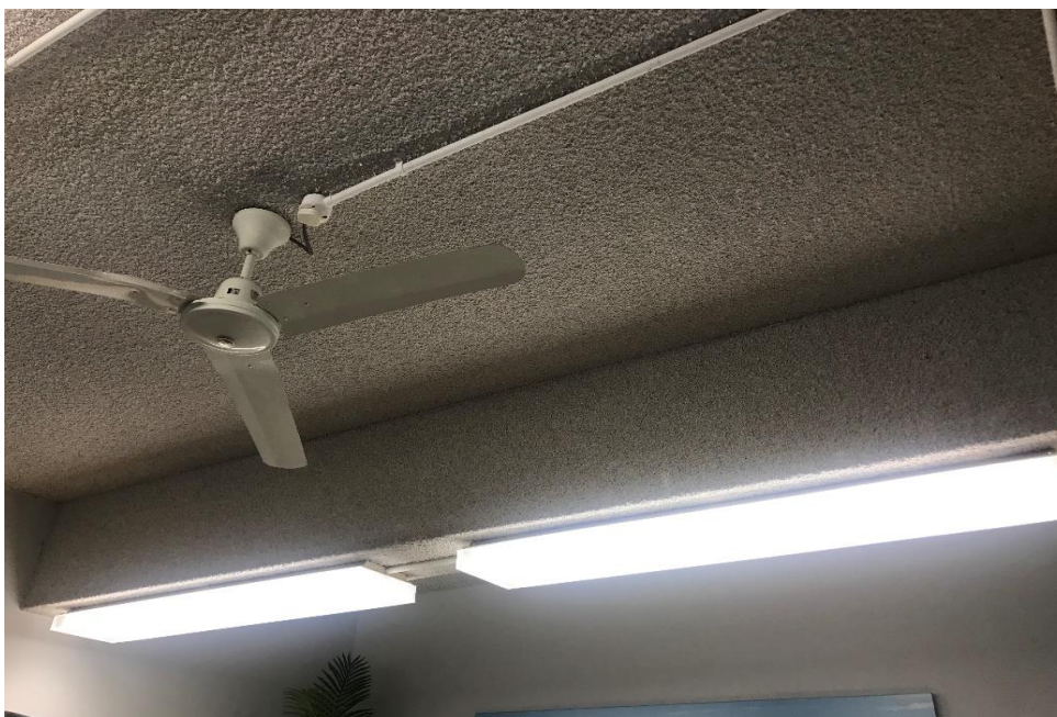
Photograph 3: B00A, AR0015, ceiling, vermiculite, no asbestos detected by analysis, SMF detected.
