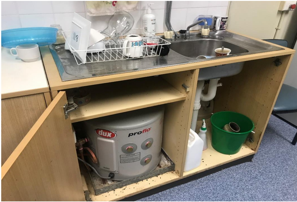
Photograph 5: B00A, AR0019, hot and boiling water unit(s), insulation, assumed SMF or foam insulation.
