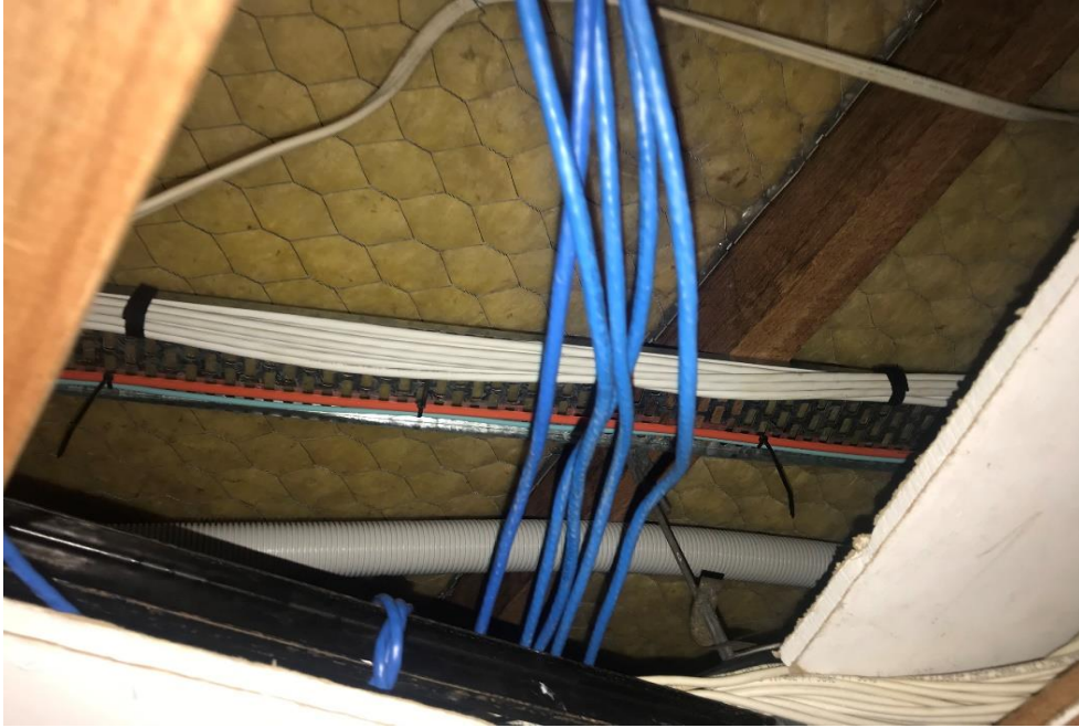
Photograph 15: B00L, LR1022, ceiling cavity, underside of roof, insulation, SMF identified visually.
