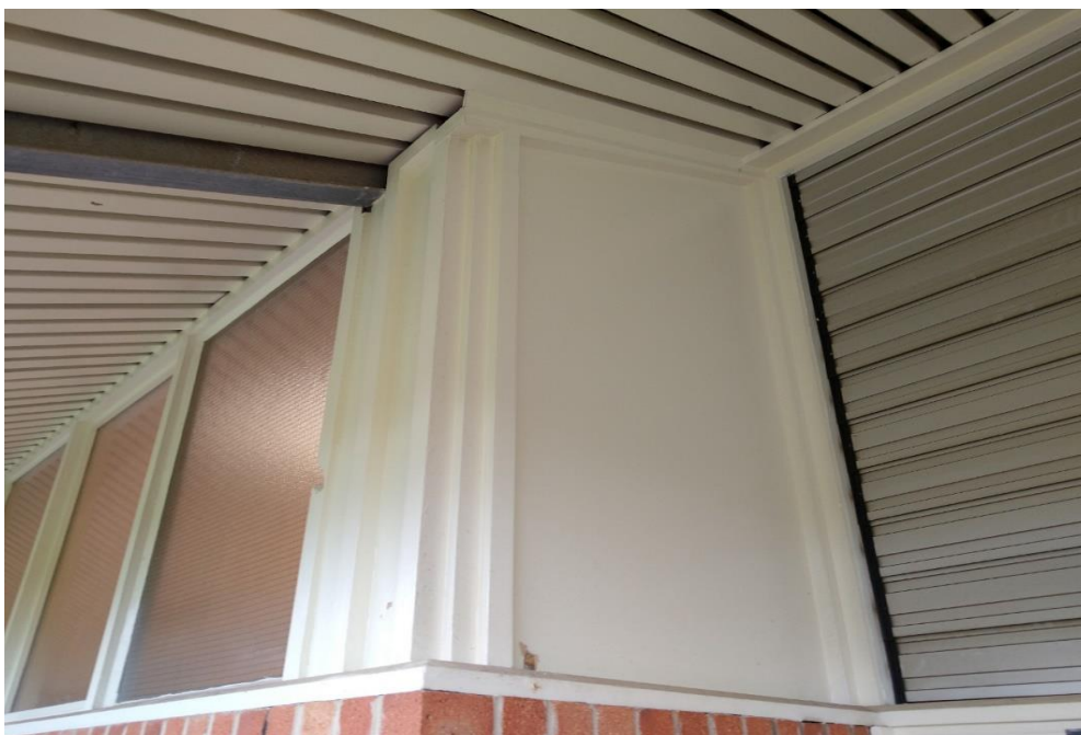
Photograph 1: BMPC, exterior, walls, cream paints and undercoats, non-lead paint ( \leq 0.1\% lead w/w).
