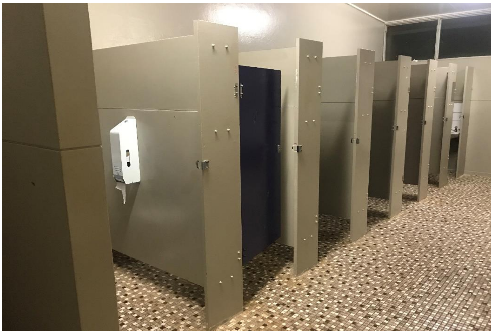
Photograph 8: B00C, CR0010, cubicles, partition walls, fibre cement board, asbestos detected by analysis.
