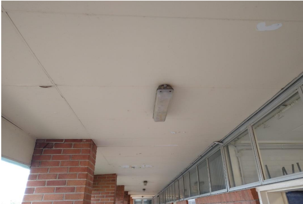
Photograph 1: B00T, R0016, ceiling, fluorescent lights, capacitors, PCB (assumed).
