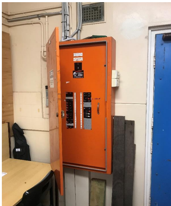
Photograph 5: B00C, CR0001, electrical cabinet, resinous board, asbestos (assumed).
