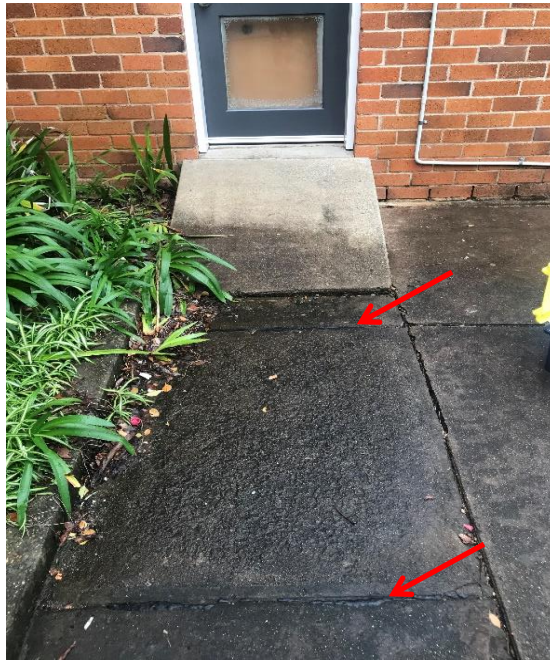
Photograph 15: B00A, exterior, paving outside AR0036, expansion gap, bitumastic, asbestos detected by analysis.
