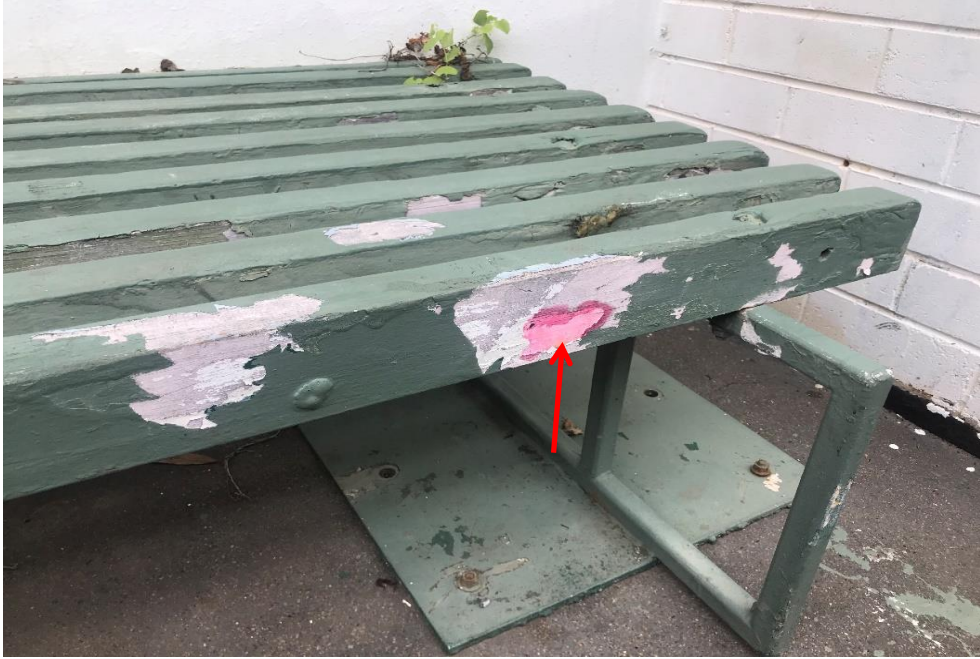
Photograph 23: B00B, exterior, northern façade, timber seating, green and underlying cream paint, lead paint (>0.1% lead w/w).
