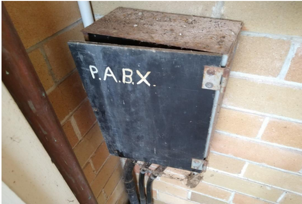
Photograph 11: B00T, R0002, electrical cupboard, electrical backing board, asbestos (assumed).
