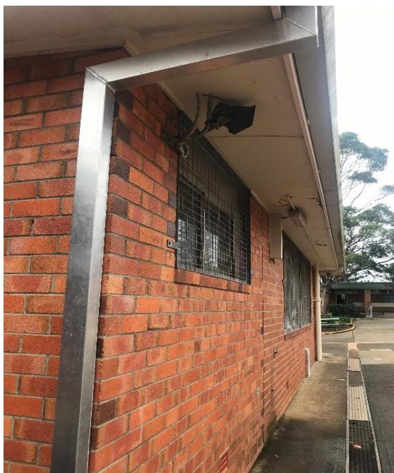
Photograph 1: B00C, exterior, eave linings, fibre cement sheet, asbestos detected by analysis.
