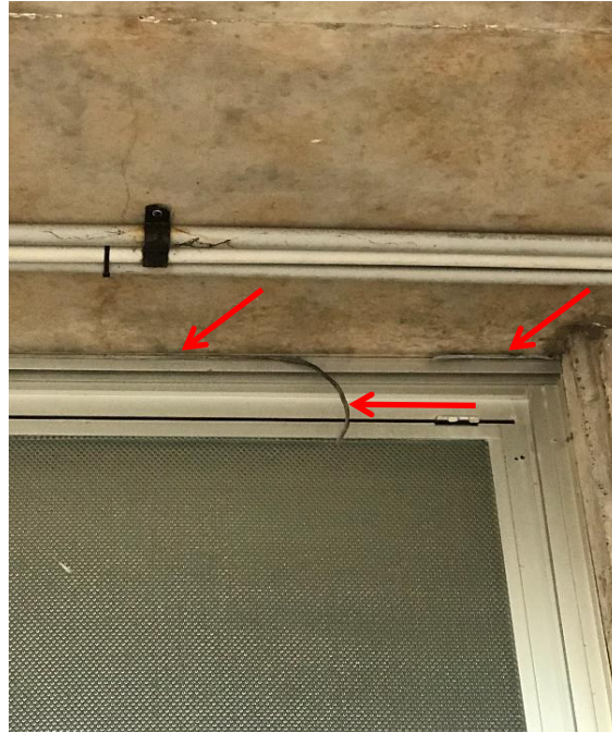
Photograph 9: B00L, LR0042, aluminium window and door sets, between window/door frame and wall, putty , asbestos detected by analysis.
