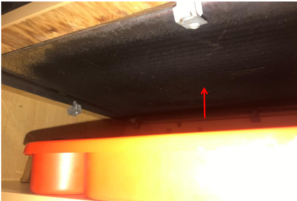
Photograph 12: B00B, BR1002, underside of sink, bituminous lining, asbestos detected by analysis.
