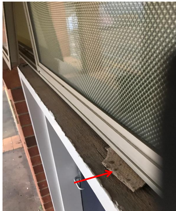
Photograph 10: B00L, LR0042, aluminium window/door frames, packing materials, fibre cement fragments, asbestos detected by analysis.
