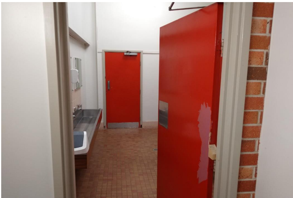
Photograph 5: BMPC, R0002, doors, red paint, non-lead paint (>0.1% lead w/w).
