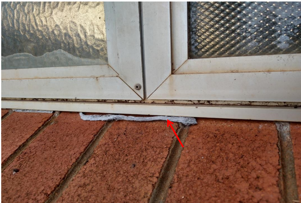
Photograph 4: B00T, exterior, window frames, putty/mastic, asbestos detected by analysis.
