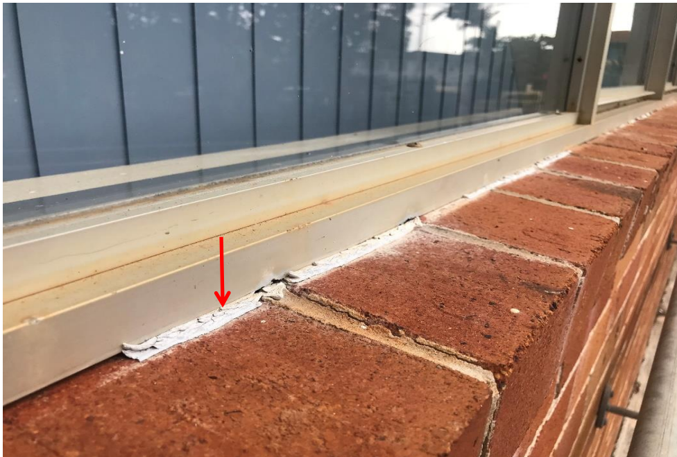
Photograph 14: B00A, exterior, adjacent north AR0020, between window frame and brick wall, putty, asbestos detected by analysis.
