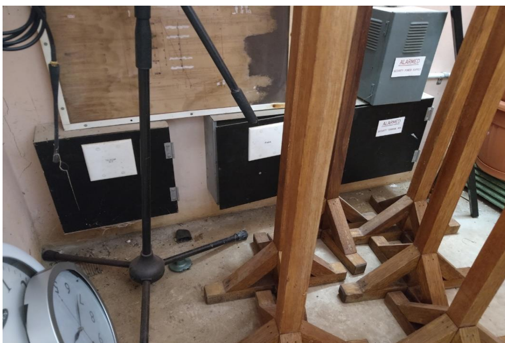
Photograph 6: BMPC, R0014, electrical cupboard, electrical backing board(s), asbestos (assumed).
