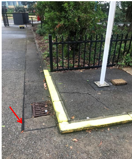
Photograph 12: B00A, exterior, exterior, northwest of building (near flagpole), expansion gap in paving, bitumastic, no asbestos detected by analysis, SMF detected.
