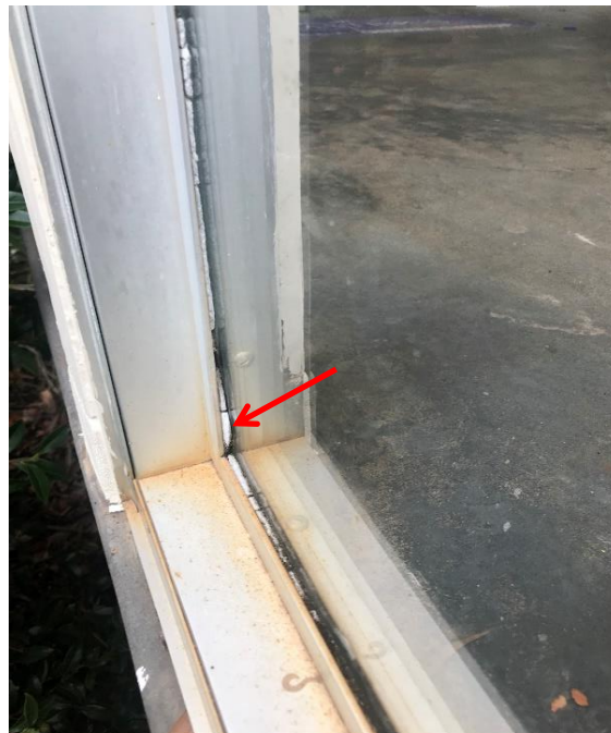
Photograph 8: B00A, AR0042, north side of room, window frame set, glazing putty, no asbestos detected by analysis, SMF detected.
