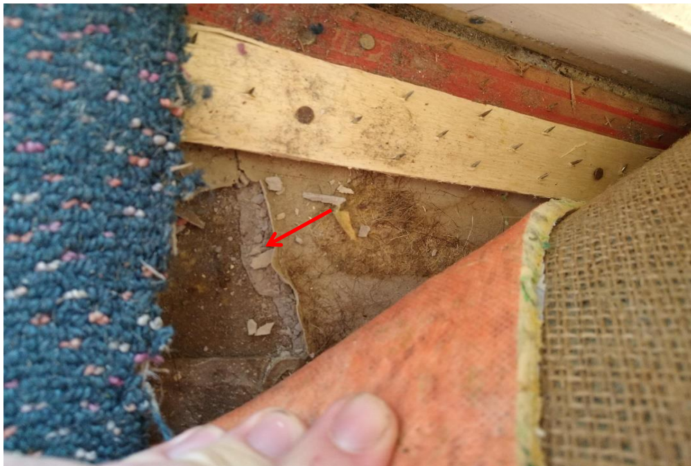
Photograph 6: B00T, R0018, under carpet, vinyl, asbestos detected by analysis.
