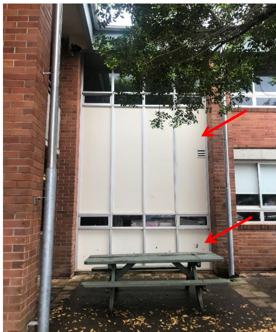
Photograph 5: B00L, exterior, window set at southern side of LR0044, infill panels, fibre cement, asbestos (assumed).
