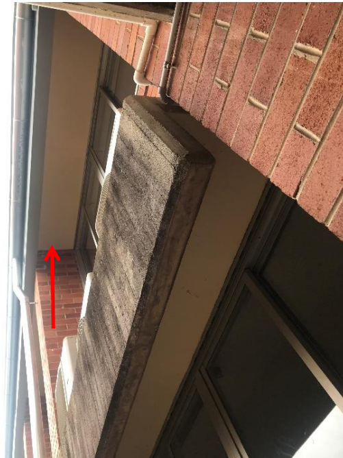
Photograph 1: B00L, exterior, western eave, fibre cement, asbestos detected by analysis.
