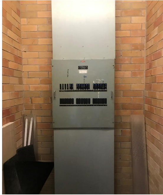
Photograph 19: B00L, LR1027 (adjacent west LR1028), enclosed within electrical cabinet, resinous backing board(s) and/or other components, asbestos (assumed).
