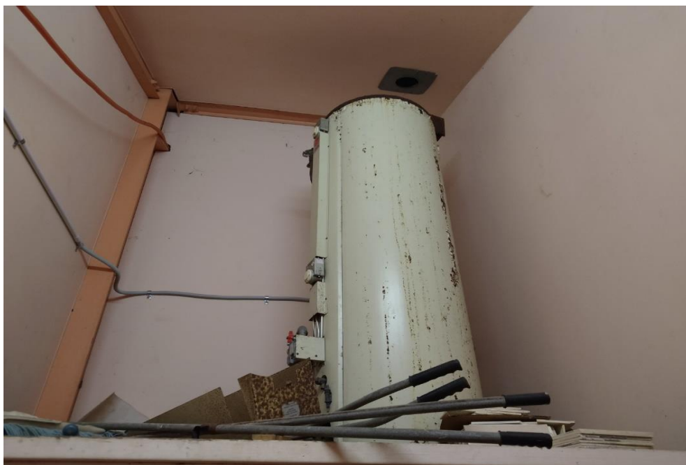
Photograph 2: BMPC, R0003, hot water heater, insulation, asbestos (assumed).
