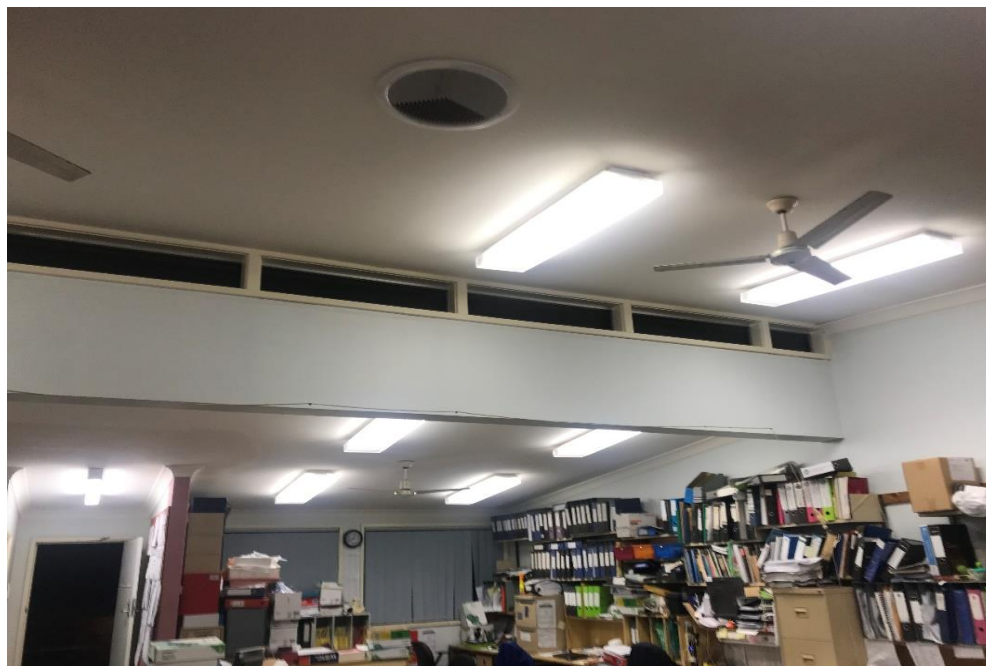
Photograph 6: BTAS, TAS-R0013, ceiling lining(s), fibre cement, asbestos detected by analysis.
