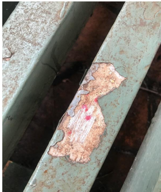
Photograph 10: B00C, CR0014, eastern end, timber seating, green paint and underlying cream paint, positive for lead.
