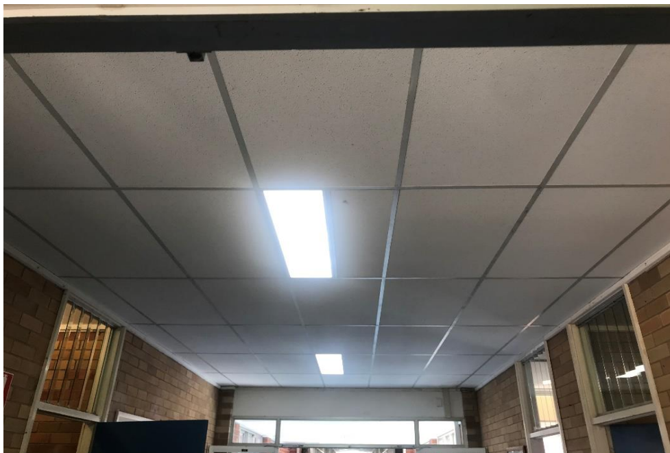
Photograph 16: B00L, LR1025, false ceiling, ceiling tiles, SMF identified visually.
