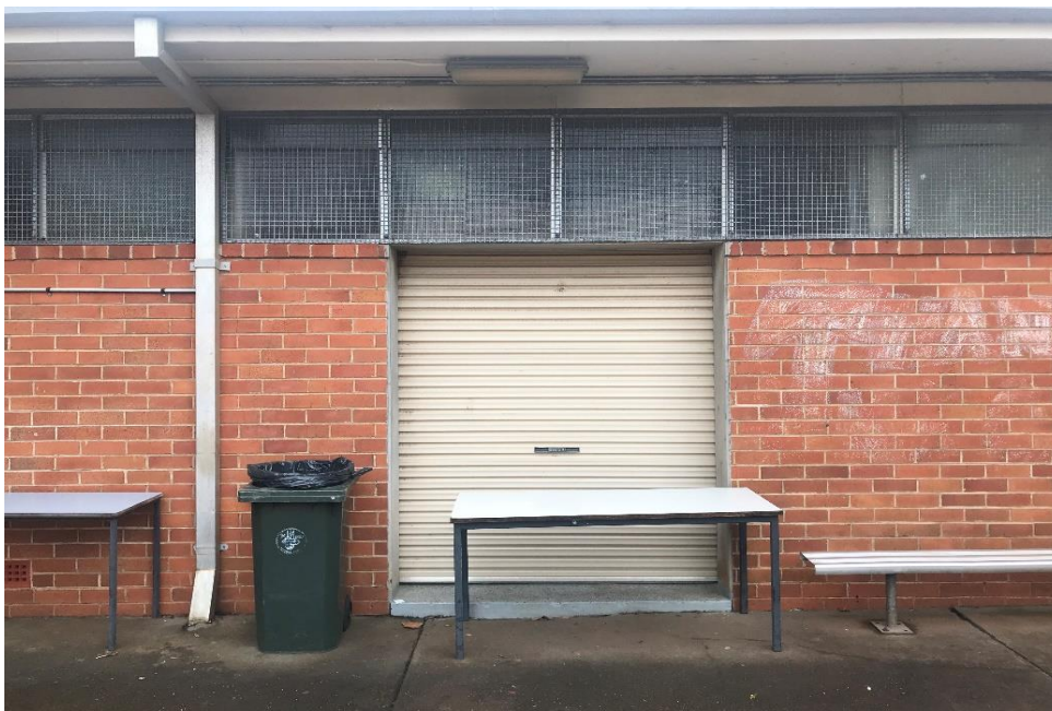
Photograph 3: B00C, exterior, concrete paving outside CR0006 roller door, expansion gap, bitumastic, asbestos detected by analysis.
