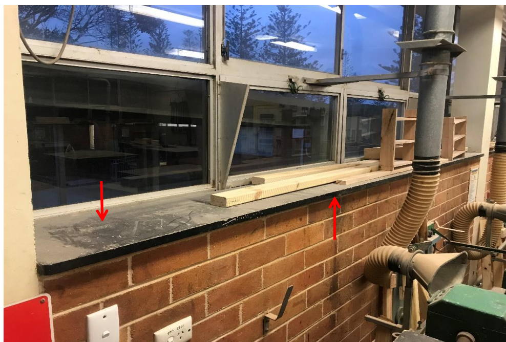
Photograph 2: BTAS, typical window sill lining(s), fibre cement, asbestos detected by analysis.
