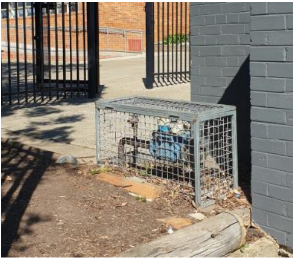
Figure 7.1: Master water meter (site main entry)
