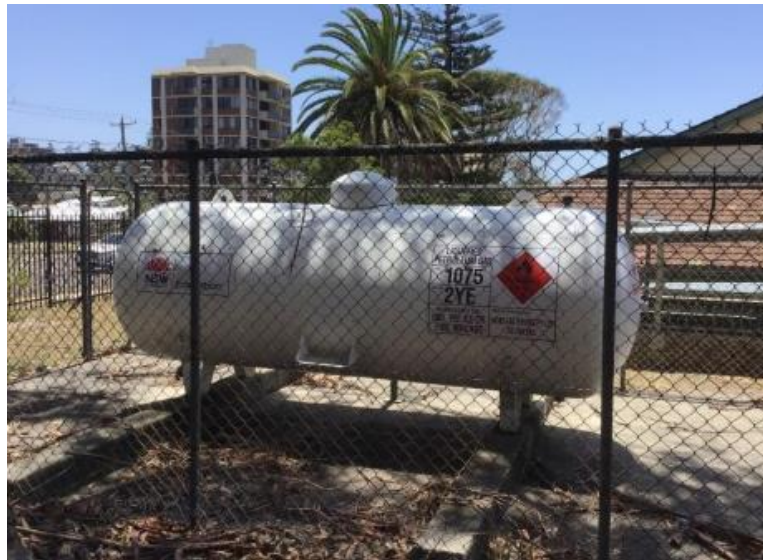
Figure 7.4: 1 Tonne Bulk LPG Storage vessel adjacent MPC building
