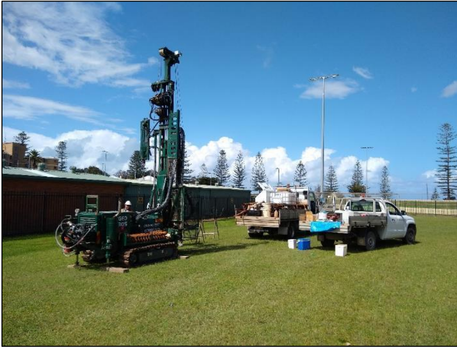
Figure 4: Drill rig on Bore 202 within Area 1 near the north-western boundary of the site
