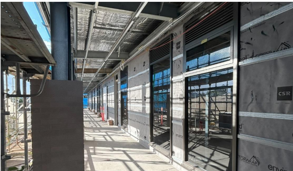
Metal framing and sheeting installation for Building T
