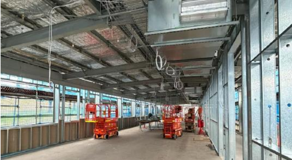
Installation of services for Building T
