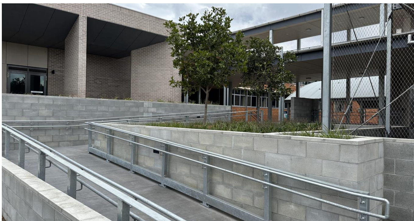
Access ramp from the TAS forecourt to the North South Link
