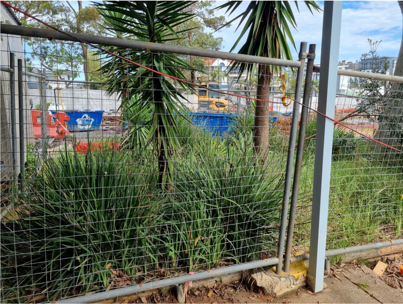
Plate 3 – Tree protection zone in place
