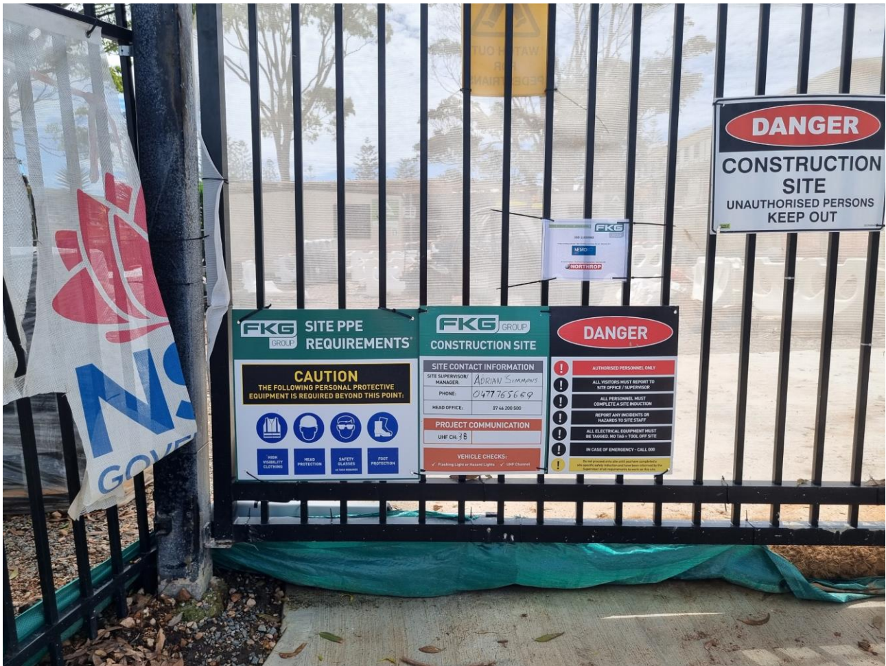
Plate 8 - Site notice at entry gate
