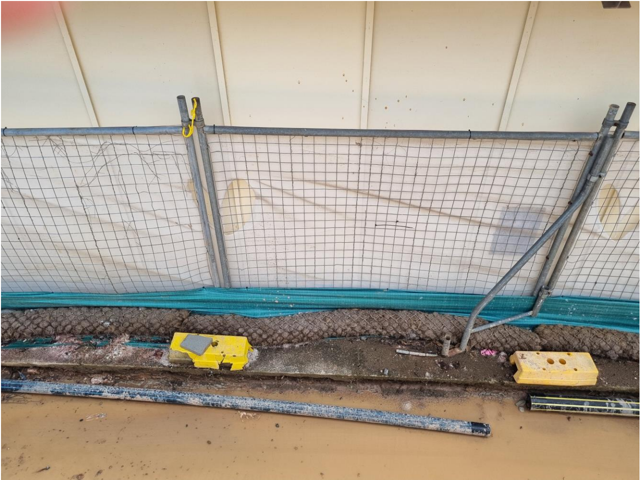
Plate 4 – Coir log and silt fence protecting north side of site
