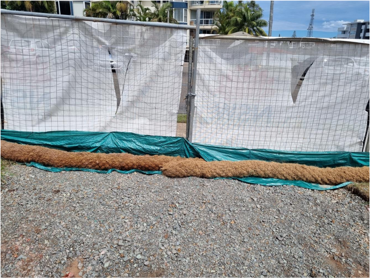
Plate 5 – Coir log and silt fence protecting Owen Street side of site
