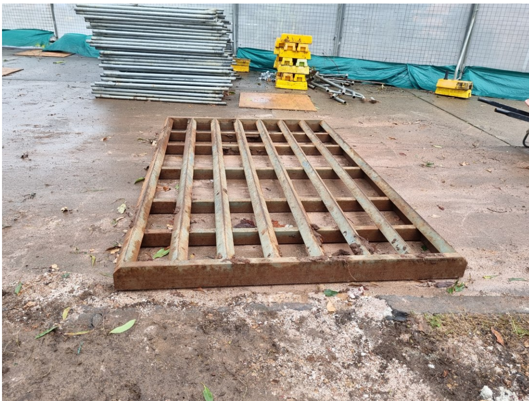
Plate 7 - Rumble grid to be installed
