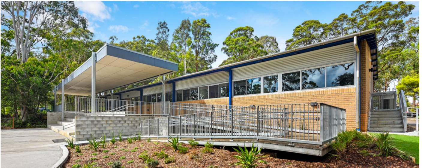
Upgraded access and ramp access
