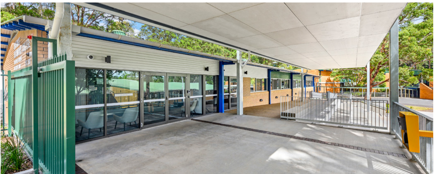
Entrance to new school reception area
