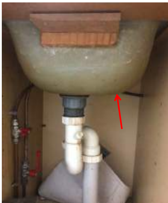
Photograph 9: B00B, BR0012, teacher's desk, moulded sink, no asbestos detected by analysis, SMF detected.
