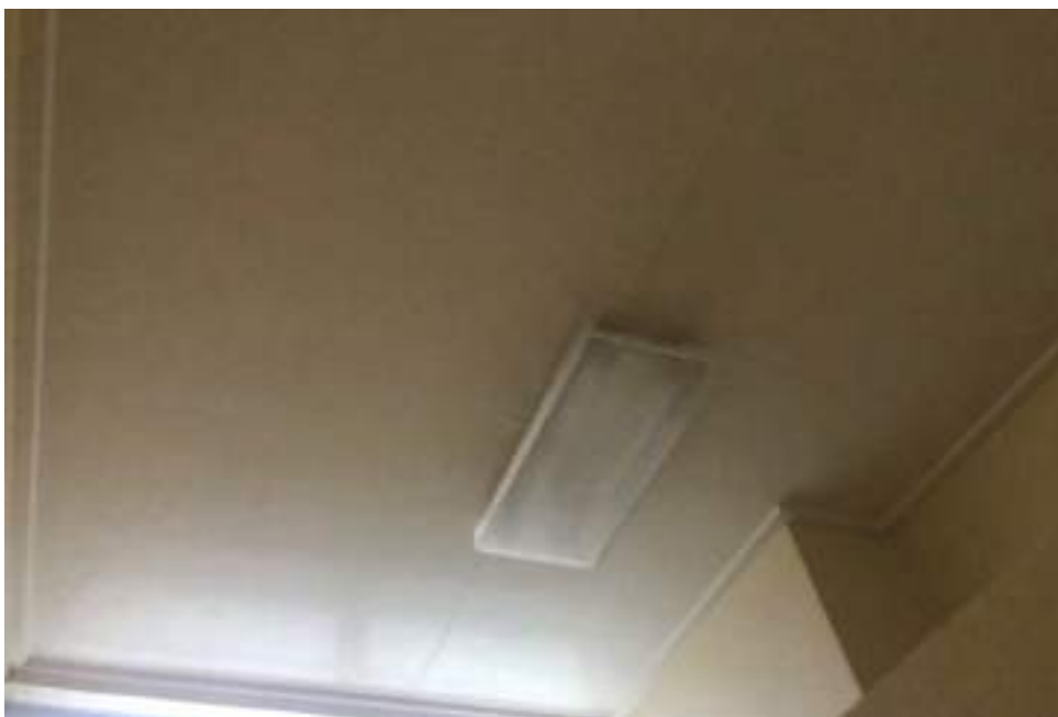
Photograph 3: B00B, BR1020, ceiling, fibre cement sheeting, asbestos detected by analysis.
