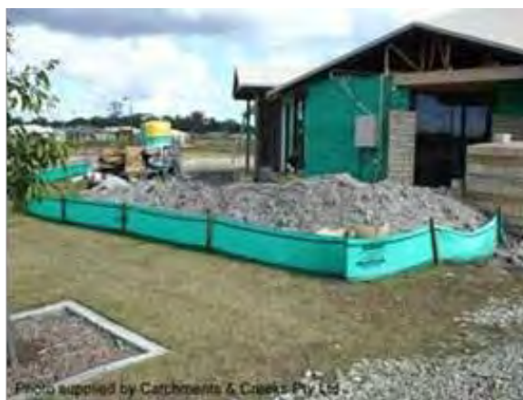
Figure 18 - Sediment fence stockpile control
