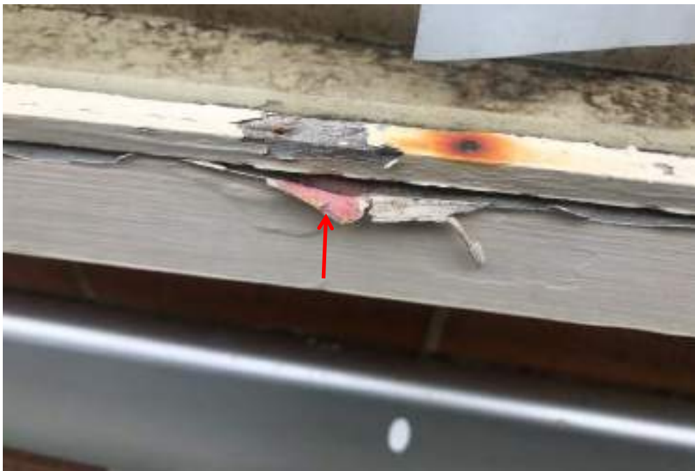
Photograph 22: B00B, exterior, northern façade, notice board, cream and underlying white paint, lead paint (>0.1% lead w/w).
