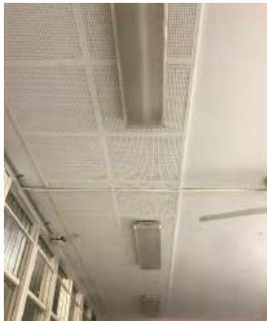
Photograph 24: B00B, rooms and areas in general, fluorescent light fittings in general, capacitors, insulating oil, PCB (assumed).
