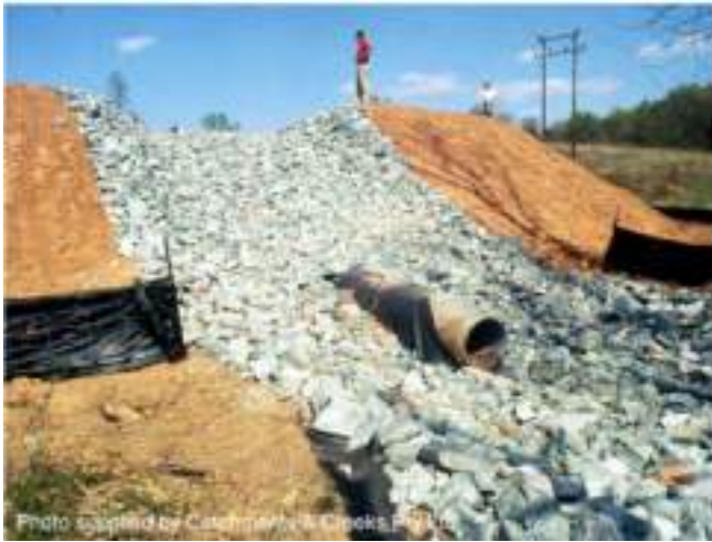
Figure 32 - Sediment Basin Spillway
