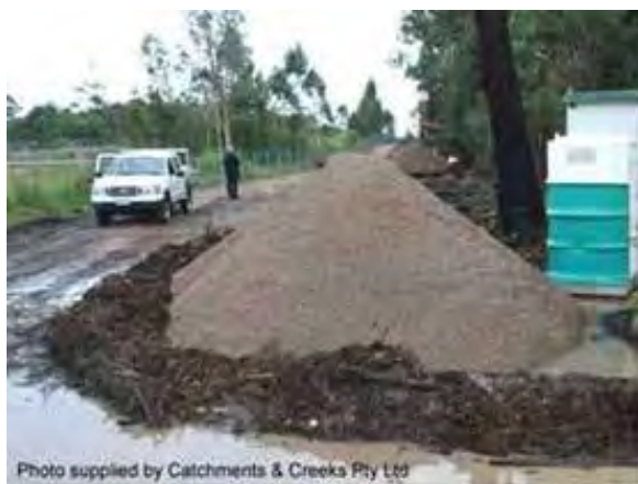
Figure 17 - Mulch berm stockpile control
