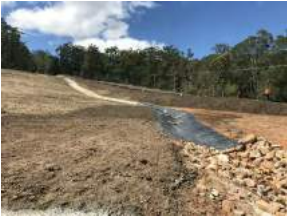
Figure 1 – Plastic-lined catch drain
