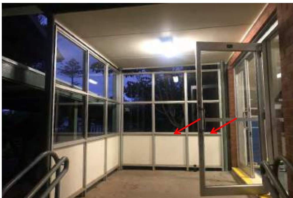
Photograph 10: B00B, BR0019, portion of infill panels (type 3), fibre cement, asbestos detected by analysis.
