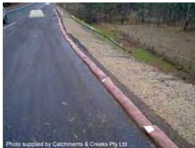
Figure 3 -Flow Control Berm
