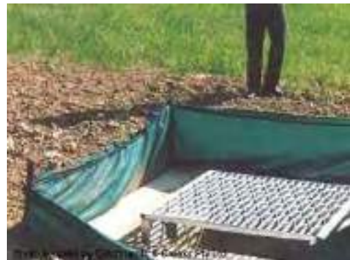
Figure 22 - Fabric drop inlet protection
