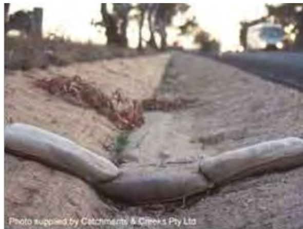
Figure 8 - Sand bag check dams
