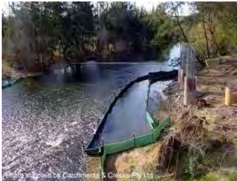
Figure 12 - Instream isolation barrier
