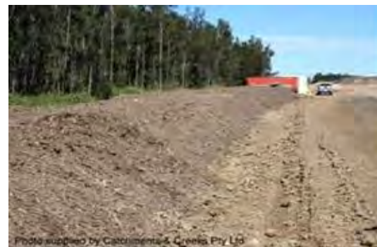
Figure 24 - Mulch berm
