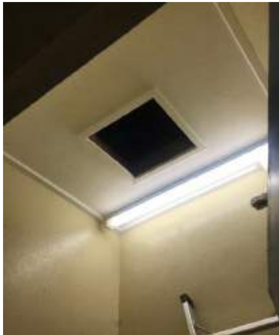
Photograph 16: B00B, BR1021, ceiling, fibre cement sheeting, asbestos detected by analysis.
