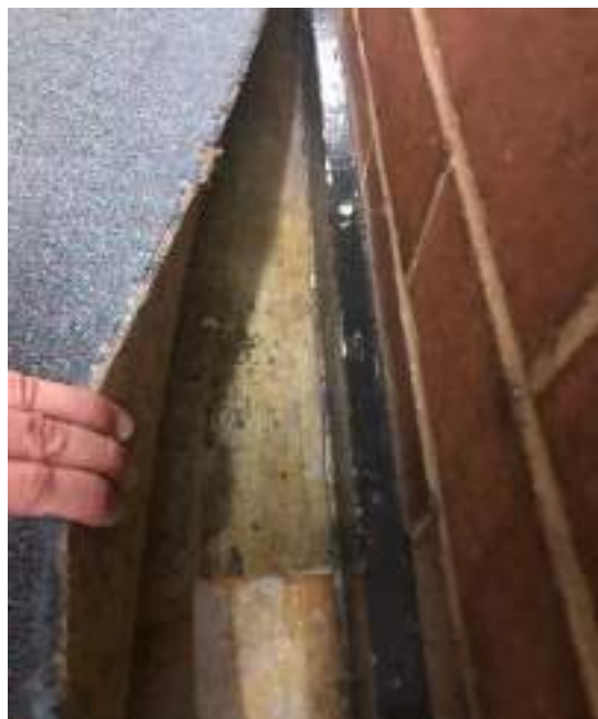
Photograph 18: B00B, BR1022, floor, below carpet, vinyl tile, asbestos detected by analysis.
