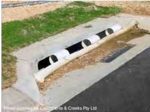
Figure 19 - Kerb Inlet sediment trap
