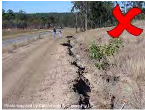
Figure 2 - Severe erosion from a catch drain cut into dispersive soils
