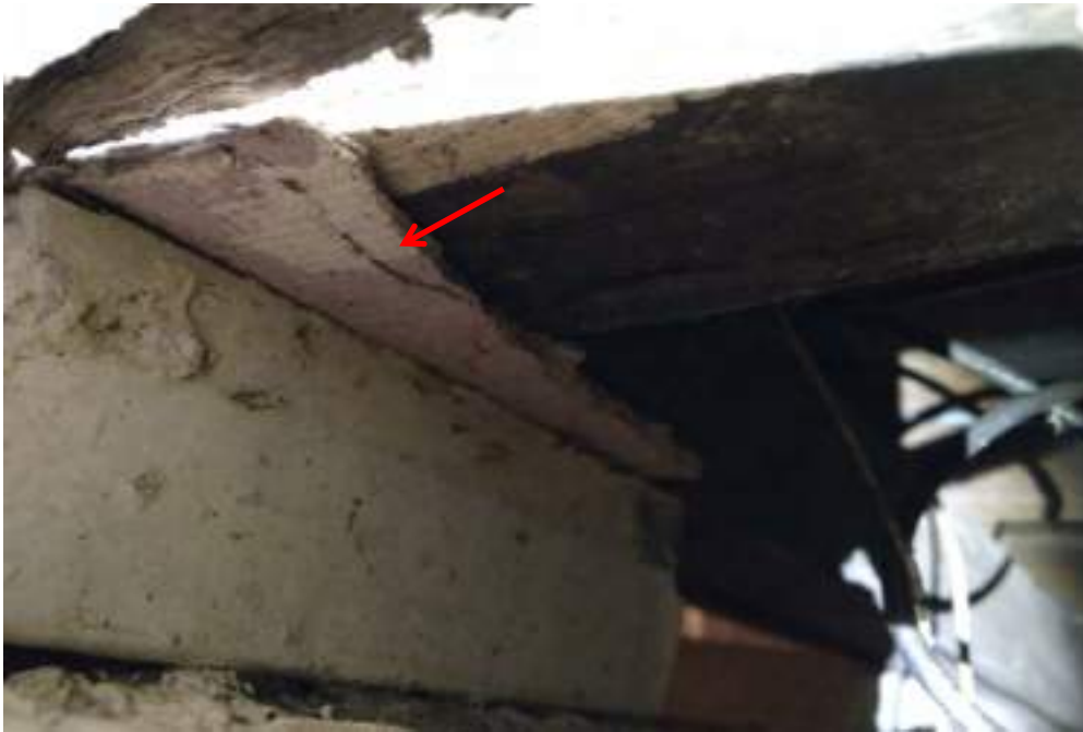
Photograph 1: B00S, subfloor, packing to accessible brick pier, fibre cement, no asbestos detected by analysis.
