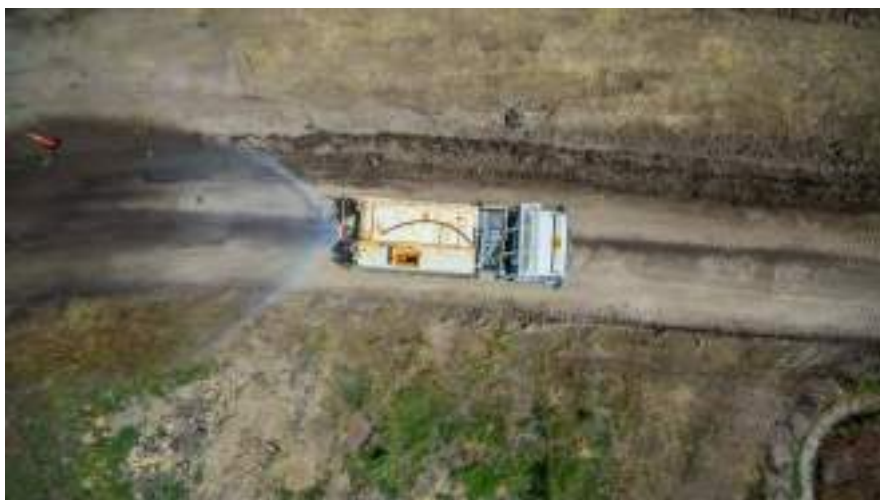
Figure 15 - Water cart application of soil binder
