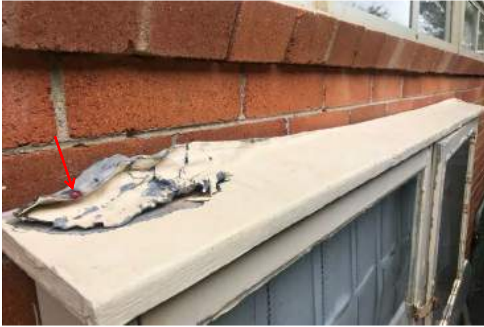
Photograph 25: B00B, exterior, northern façade, notice board, flashing, positive for lead.
