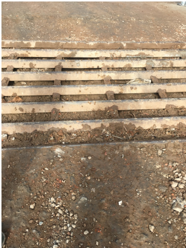
Figure 4 Entry/ exit point to site with rumble grid
