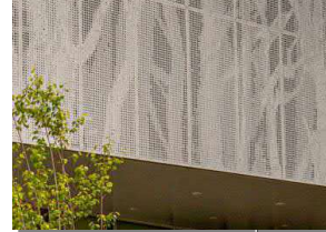
SCN-203 Perforated Metal - Art pattern Arcadia: Profiled, Perforated Metal Screens and Support System, Colours and pattern to be confirmed
