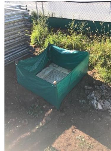
**Photo 14 – Stormwater Pit Protection – C26 & 28**
