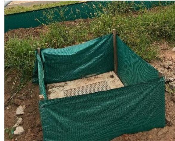
**Photo 10 – Silt fence around drain**
