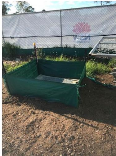
**Photo 13 – Stormwater pit protection – C26 & 28**
