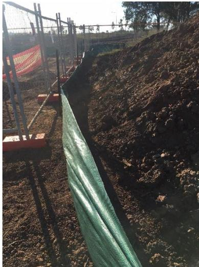
**Photo 15 – Silt Fence to stockpile – C26 & 28**
