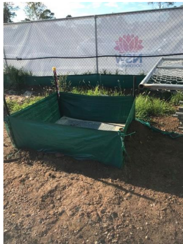
Photo 13 – Stormwater pit protection
