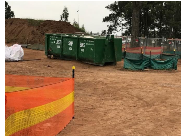
Photo 8 – Skip bins in various site locations
