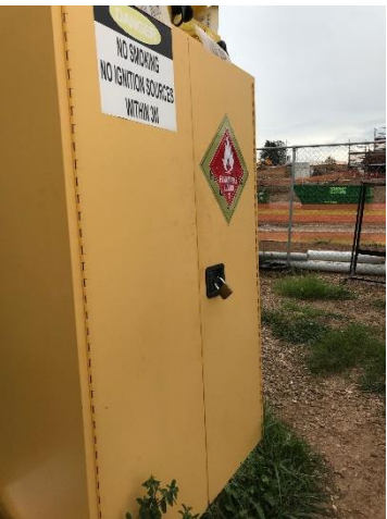
Photo 2 – Container for Hazardous Materials
