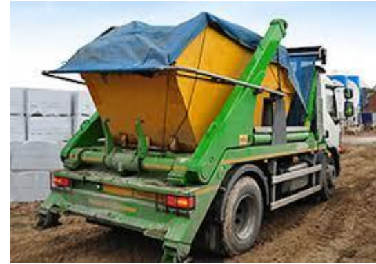
Photo 18 – Covered waste removal
