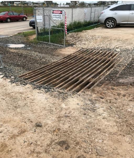
Photo 4 – Rumble grid at site entrance
