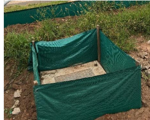
Photo 10 – Silt fence around drain
