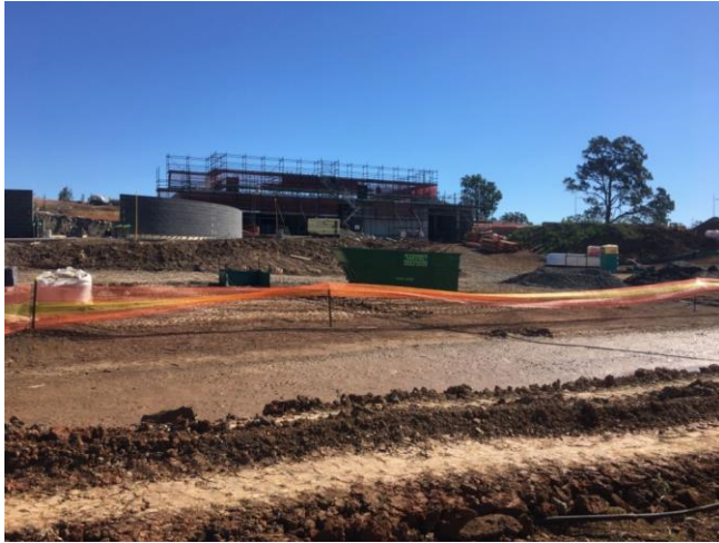
Photo 21 – Sediment basin modification
