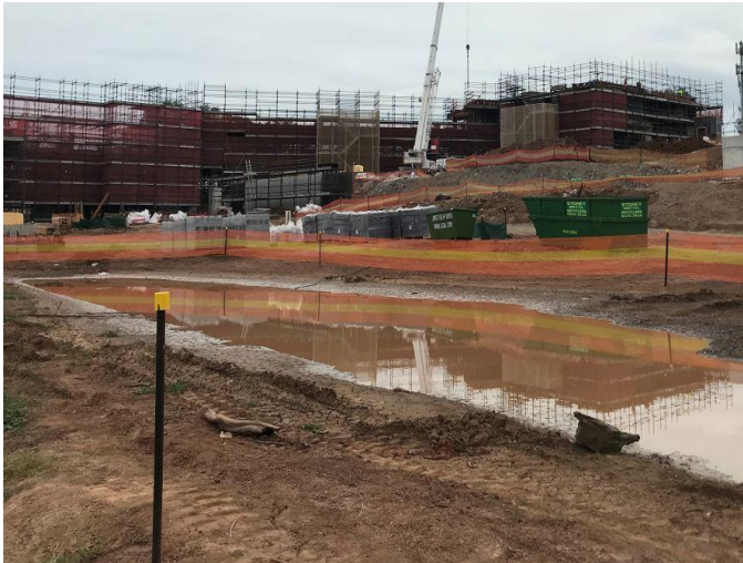
Photo 5 – Sedimentation Basin
