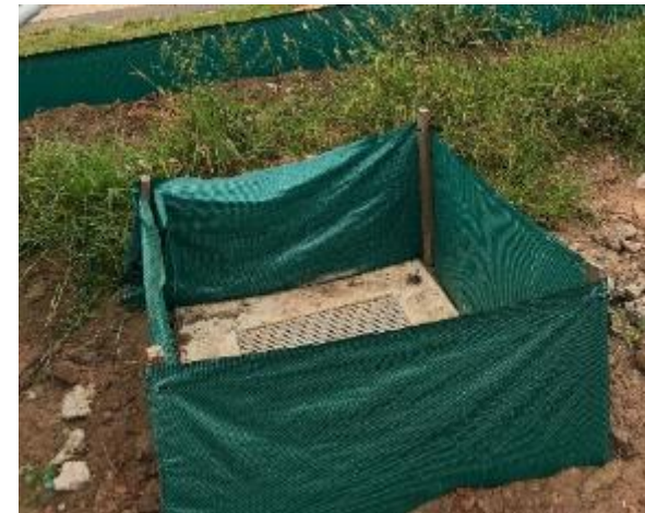
Photo 11 – Silt fence around drain
