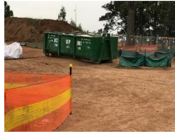
Photo 9 – Skip bins in various site locations
