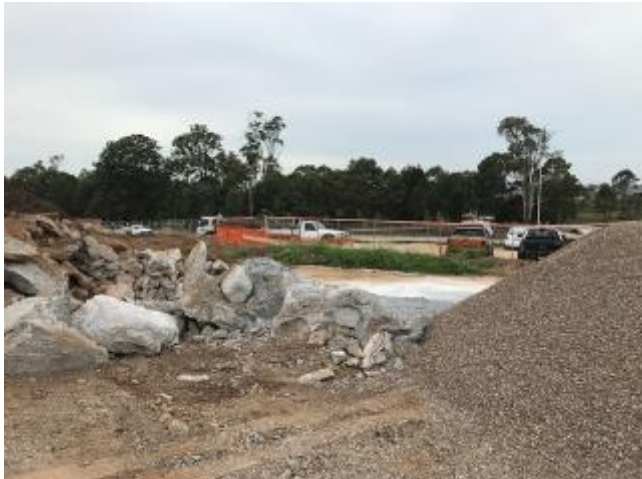
Photo 1 – Concrete Washout Bay – concrete was noted to be removed.
