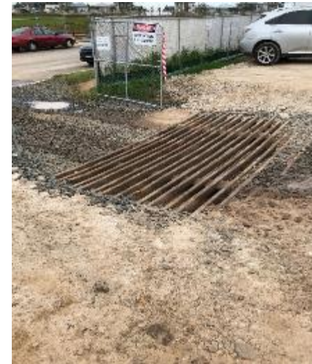
Photo 5 – Rumble grid at site entrance
