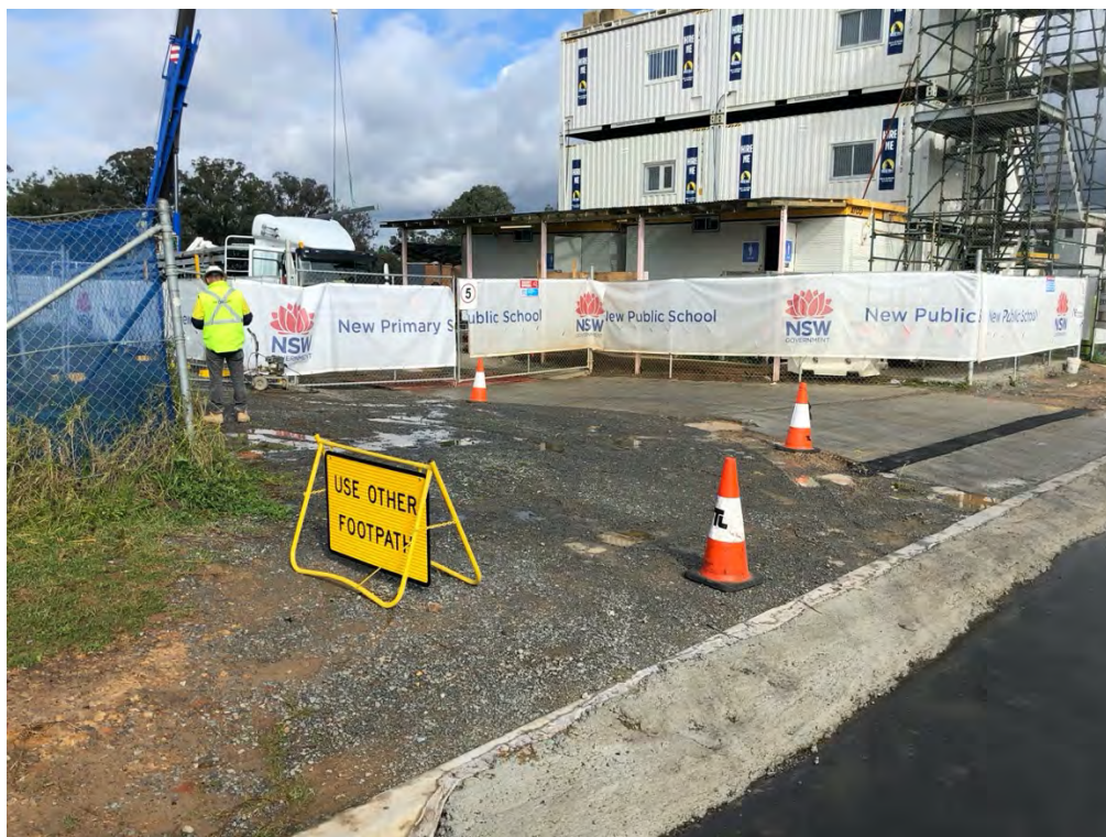
Figure 4 Site entrance with manual wheel wash and rumble grid
