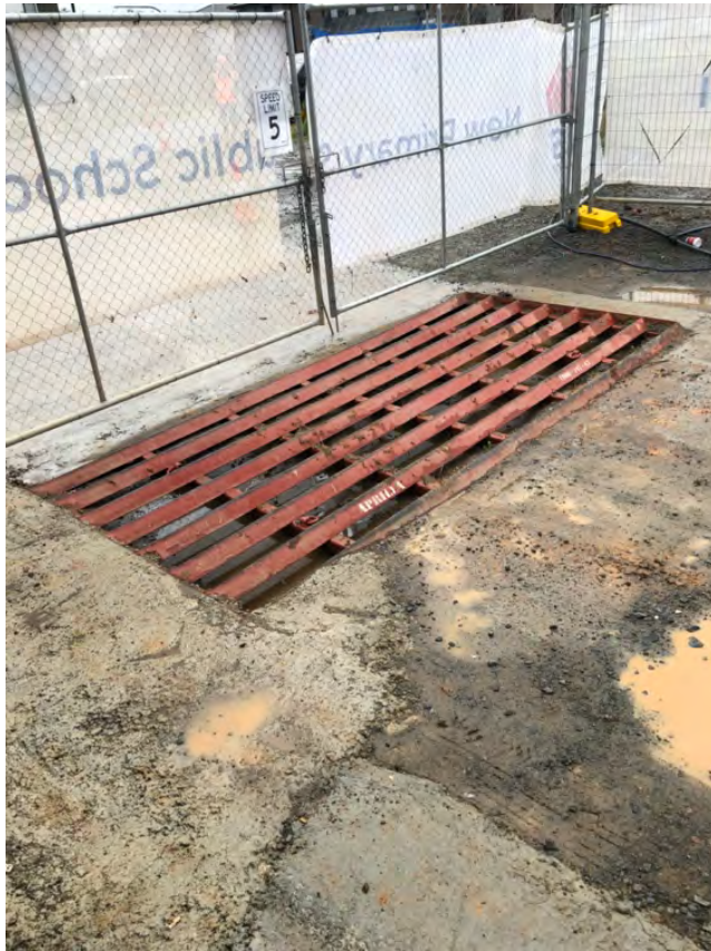
Figure 5 Entry/ exit point to site with rumble grid
