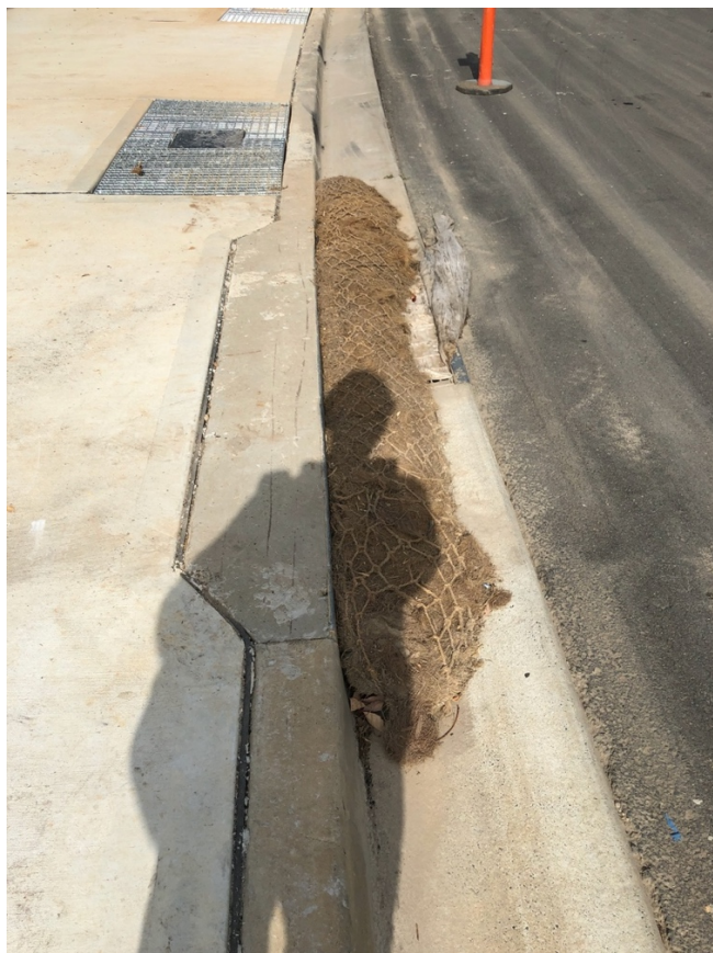
Figure 6 Stormwater sediment controls
