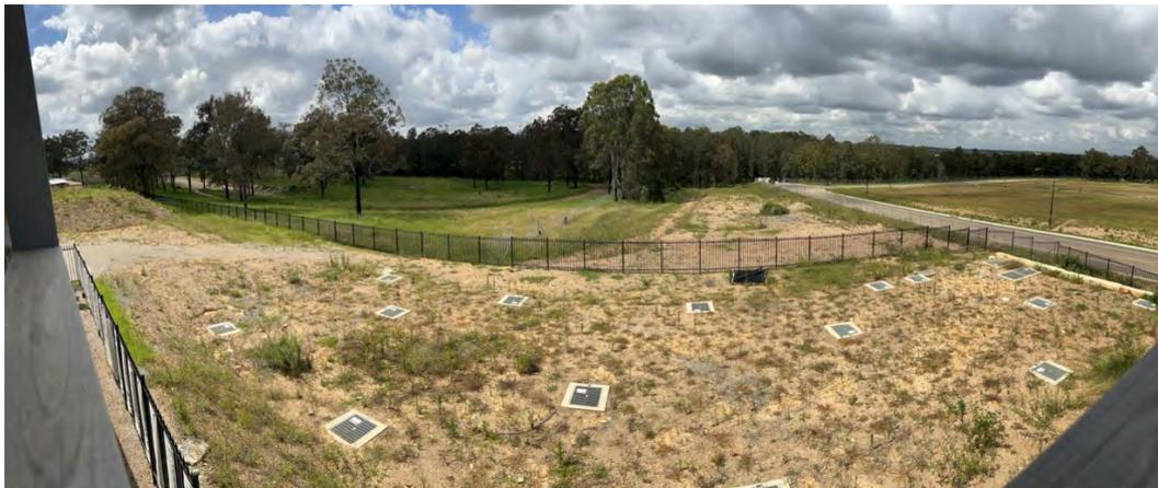
Figure 20 Adjacent OSD drainage and offsite discharge
