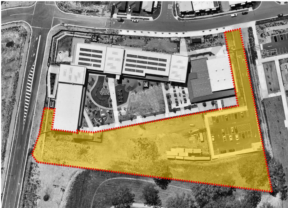
Figure 1: Stage 2 construction works location and Stage 1 buildings.
