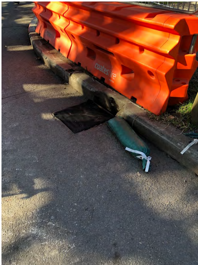
Figure 7 Adequate protection of stormwater drains
