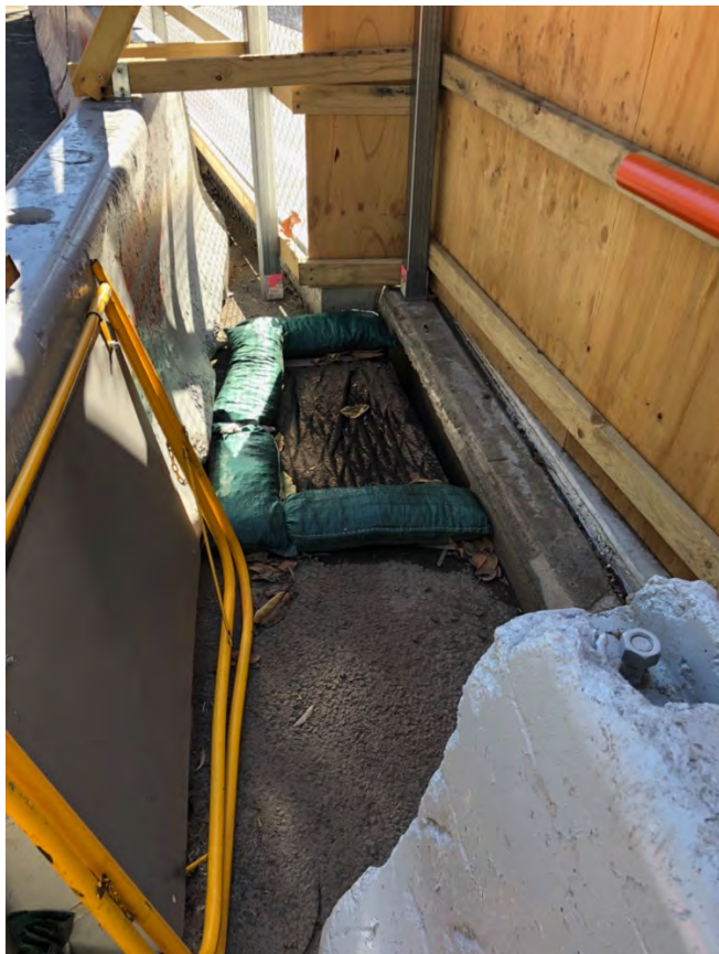
Figure 8 ERSED controls in place to protect stormwater drains
