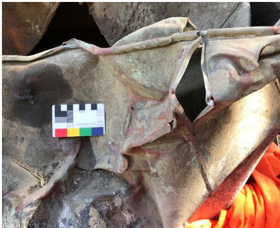
Figure 21. Detail of split seam on wall of outer pan
