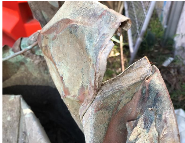
Figure 22. Detail of split seam on outer pan at rim
