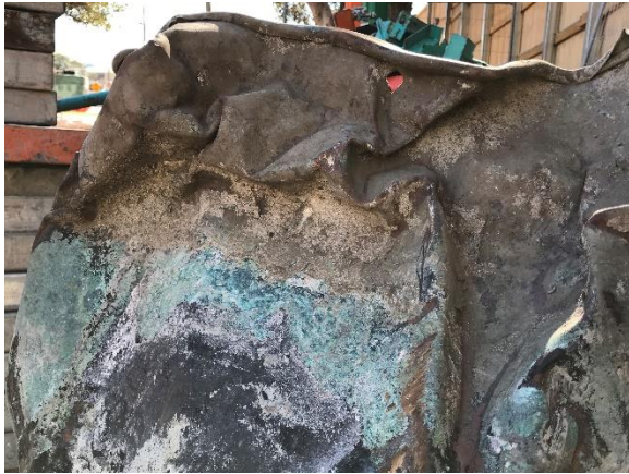
Figure 19. Detail of adherent dirt and corrosion product with clear line indicating depth to which the pans were set in soil/ concrete
