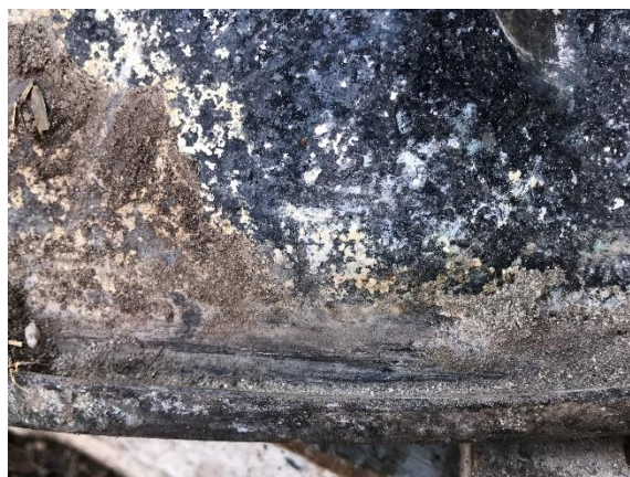
Figure 18. Detail of folded seam at base of outer pan
