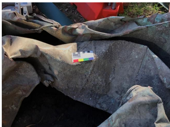
Figure 17. Detail of two folded seams in wall of inner pan
