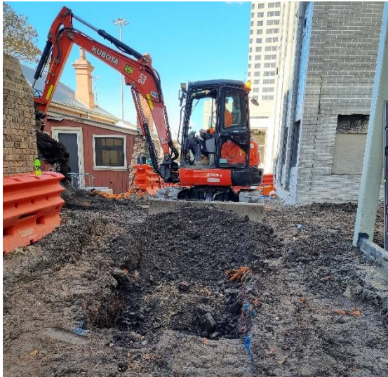
Figure 6-13 Excavator between Messenger's Cottage and Building H..
