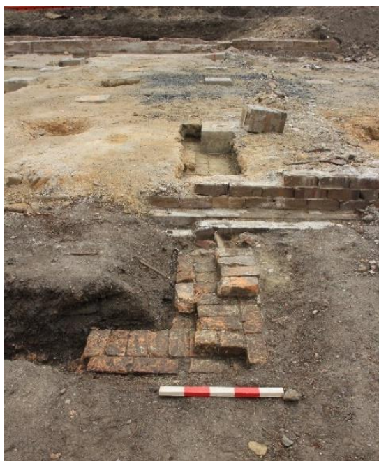
Figure 6-32. View north showing truncated return for the Cottage's southern and eastern elevations (Room 4). Modern brick footings and concrete pads for the EEC Building are visible in the background, also truncating the Cottage foundations
