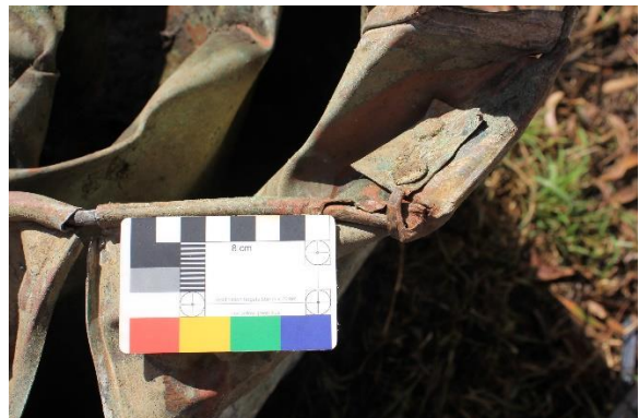
Figure 6-6 Detail of rivetted joint at basin side
