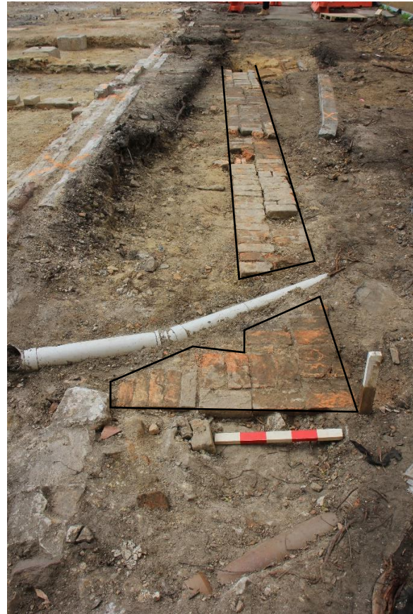
Figure 6-43. View east along the Cottage's southern elevation (outlined in black) showing a modern PVC pipe truncating its southwest return.
