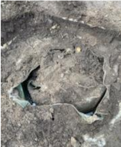
Figure 6-1 Copper basin as exposed in the ground. Note that it filled with concrete.
