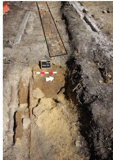
Figure 6-39. View west along the southern elevation of the Surgeon's Cottage (outlined in black) showing modern garden soils to the right (south) of exposed Cottage and EEC Building footings and partially exposed bedrock in the foreground. Two services in the bottom left of the photo may represent Phase 5-7 utilities.
