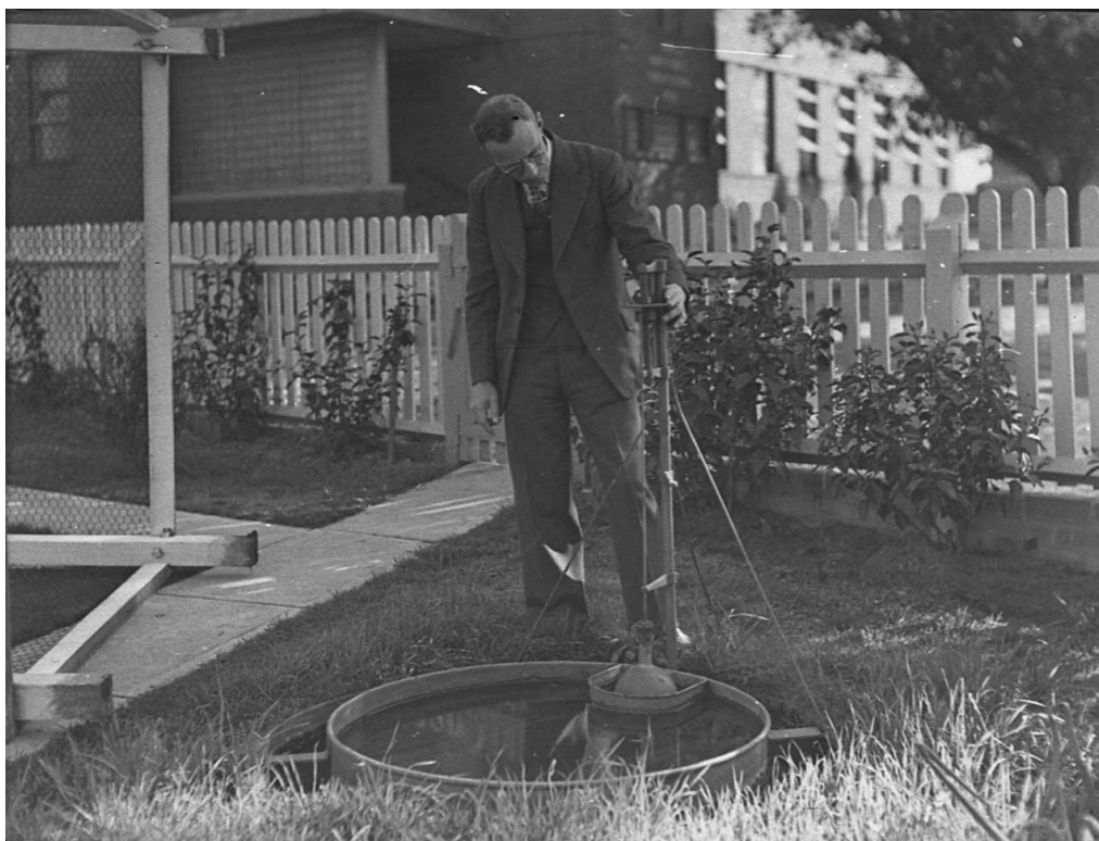
Figure 1. 1947 Image of meteorological evaporation pans in use (supplied by Curio Projects)
