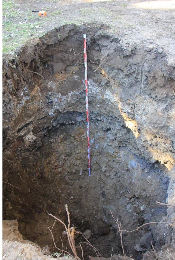
Figure 2-13. Environmental Pit 10 showing disturbed construction fills to over 3m depth. Source: Curio, 2019.
