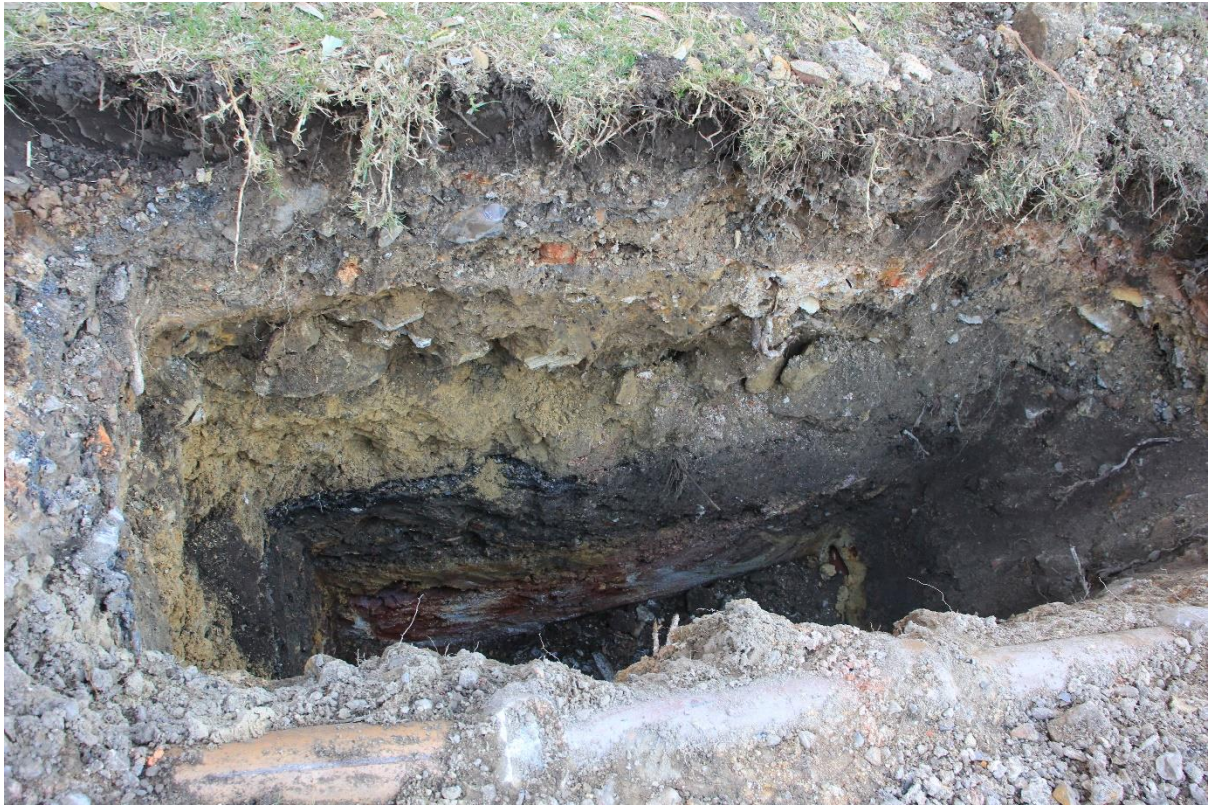
Figure 2-10. Western section of Test Trench 7 showing mixed fills and 7.004 (bitumen surface). Source: Curio 2019.
