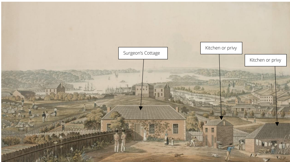
Figure 3-6. Panoramic view of Port Jackson c.1820 drawn by Major James Taylor and engraved by R. Havell & Sons looking east towards the back of the Surgeon's Cottage. The detached kitchen is visible to the right along with what is likely a privy. The Military Hospital is just out of frame, to the right. Convicts quarrying windmill hill are visible in left of frame. Source. SLNSW, Call numbers: V1/ca. 1821/4, V1/ca. 1821/5, V1/ca. 1821/6.
