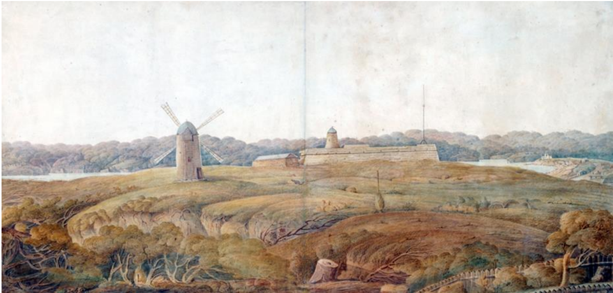
Figure 3-3. Detail of image showing the third Government (smock) windmill with the first stone mill within Fort Phillip.c.1818 Third Government Windmill (current Fort Street School Site) in front of Fort Phillip. Source. Mitchell Library SLNSW A1528797/M1942.
