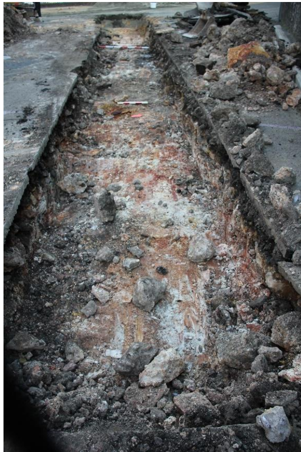
Figure 2-5. Test Trench 2 after excavation showing 2.006 exposed at the base of trench. Source: Curio, 2019.
