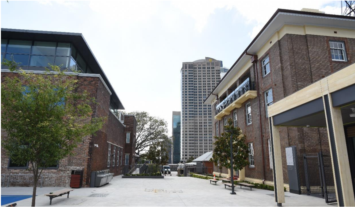
Figure 10-19: View east along central circulation spine between the Bureau of Meteorology (right) and Fort Street Public School (Left) (Source: Curio, 2023)
