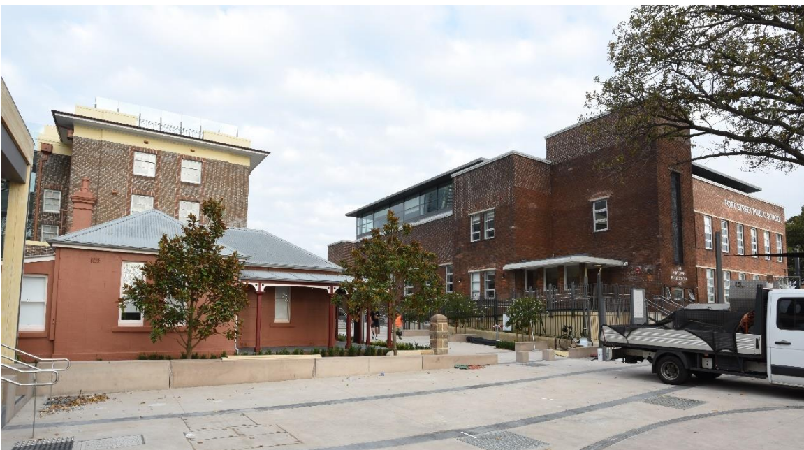
Figure 10 -20: View east along central corridor, with all three heritage listed buildings in view (Source: Curio, 2023)
