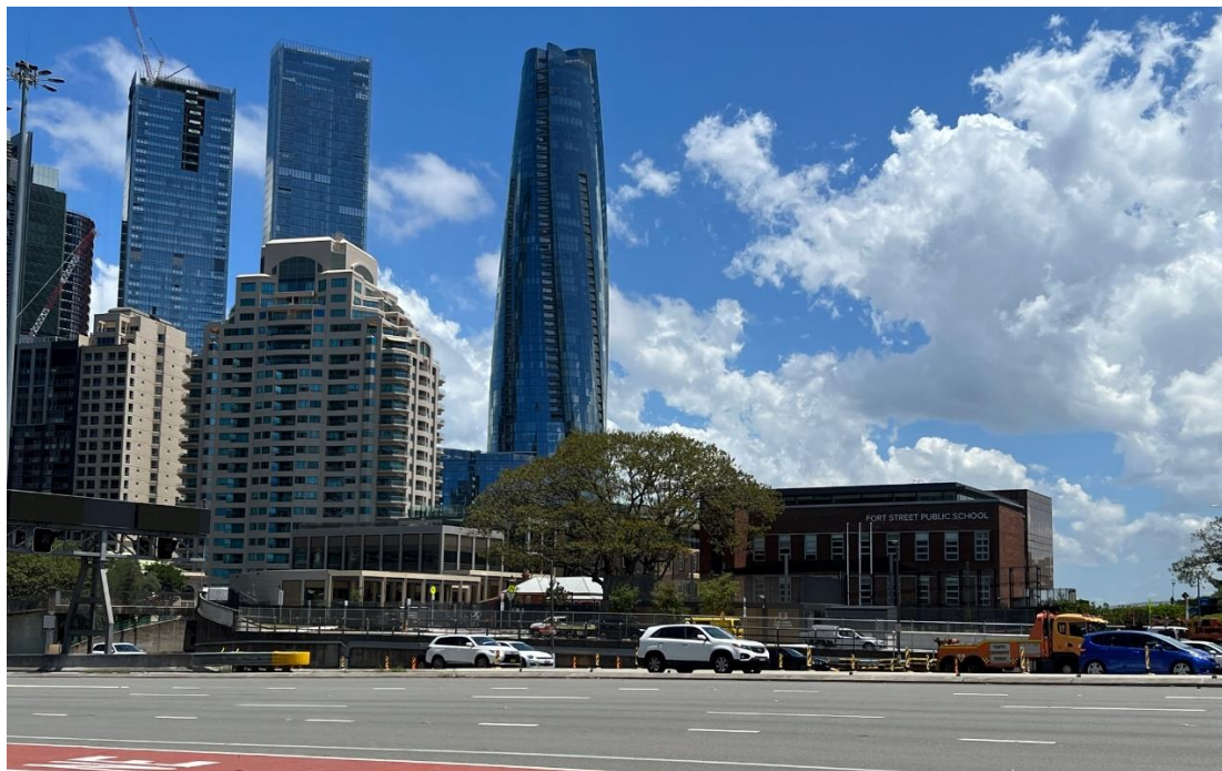
Figure 10-8: Fort Street Public School Building visible from eastern side of Bradfield Highway (Source: Curio 2024)
