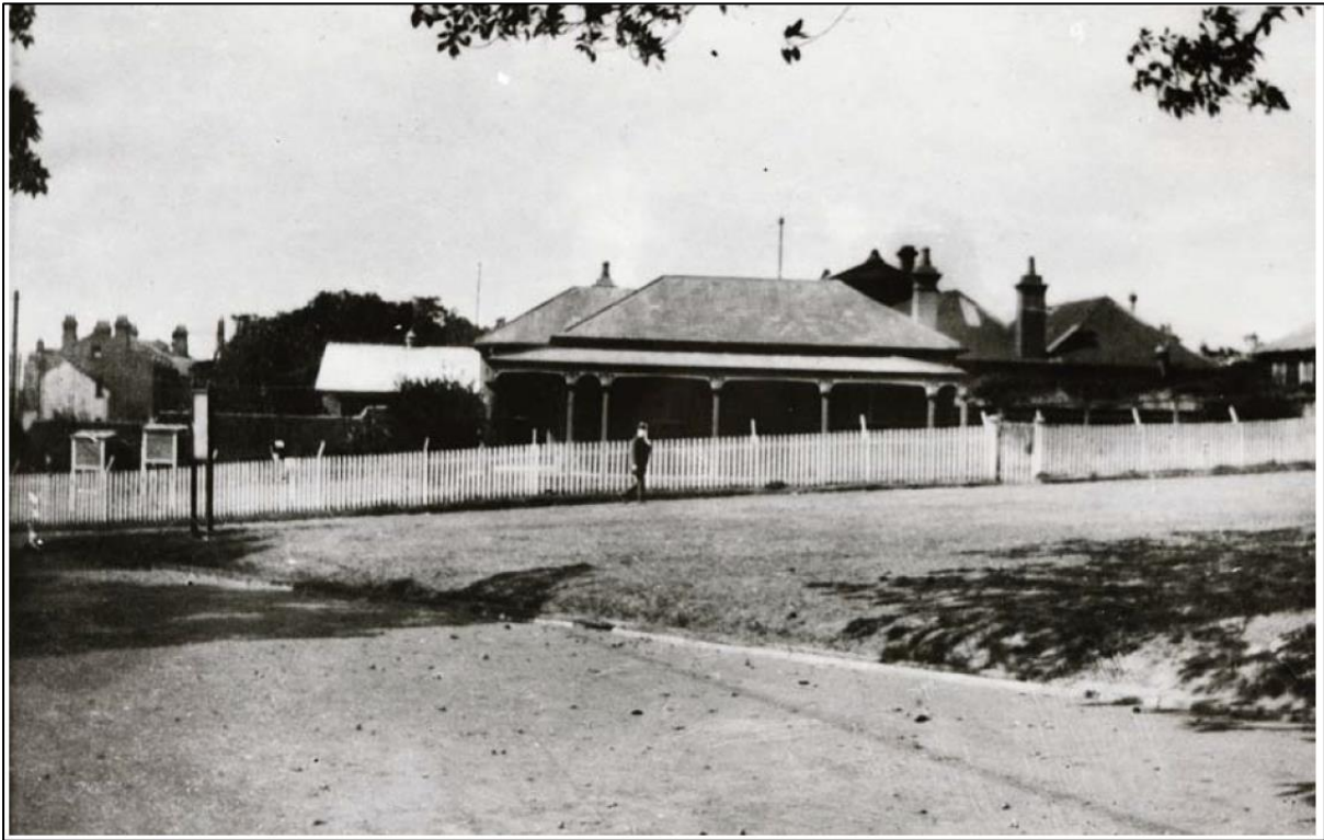
Figure 0-37: The Messenger's Cottage in 1918, after occupation by the Meteorological Bureau. (Source: observatoryhilleec.nsw.edu.au.)
