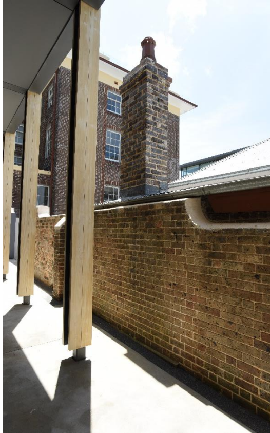
Figure 10-21: View of the Boundary Wall behind the Messenger's Cottage (Source: Curio, 2023)
