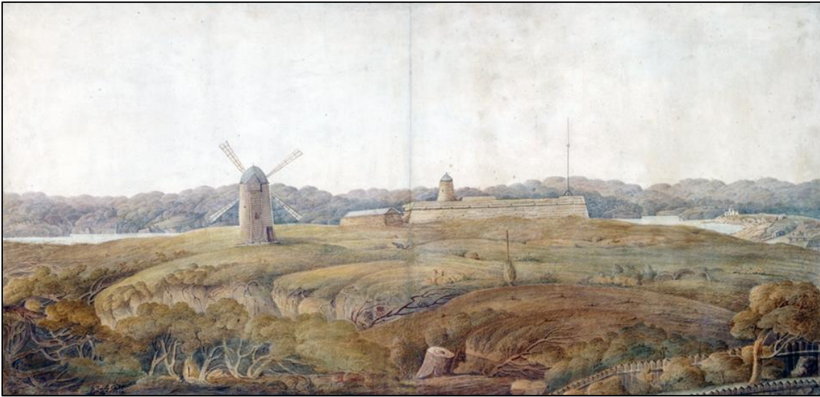
Figure 0-4: c.1818 Third Government Windmill (Current School Site) in front of Fort Phillip (Source: Mitchell Library SLNSW A1528797/M1942).
