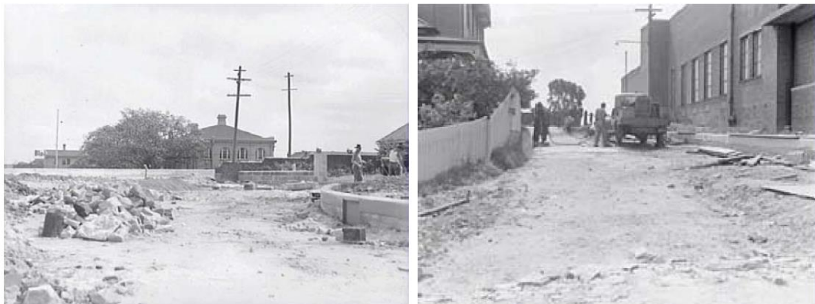
Figure 0-26: Photographs taken in 1941 showing construction of roadworks and fencing in the vicinity of the Public School. (Source: City of Sydney Archives SRC13421 and SRC13420.)
