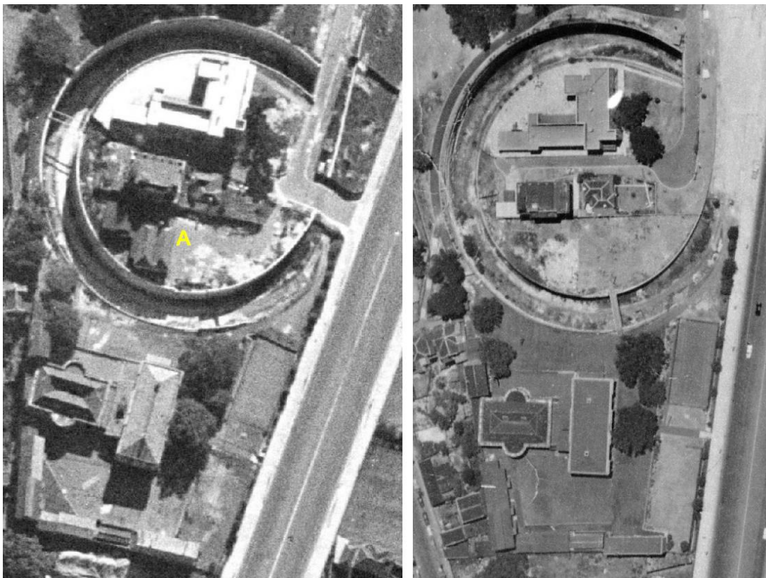
Figure 0-27: Aerial photographs taken in 1943 (left) and 1949 (right). During the intervening period of six years buildings associated with Fort Street School that were situated behind the Bureau of Meteorology, including the former surgeon's cottage associated with the Military Hospital (indicated at A), were demolished. (Sources: City of Sydney Archives Historical Atlas of Sydney; Spatial Information Exchange.)
