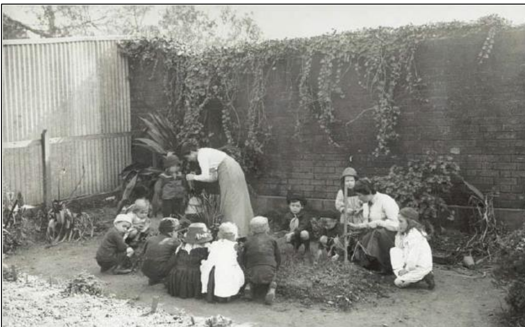
Figure 0.51: Circa 1910 photograph showing children being taught about gardening in front of the southern side of the wall. (Source: State Records Digital ID 15051_a047_005381)
