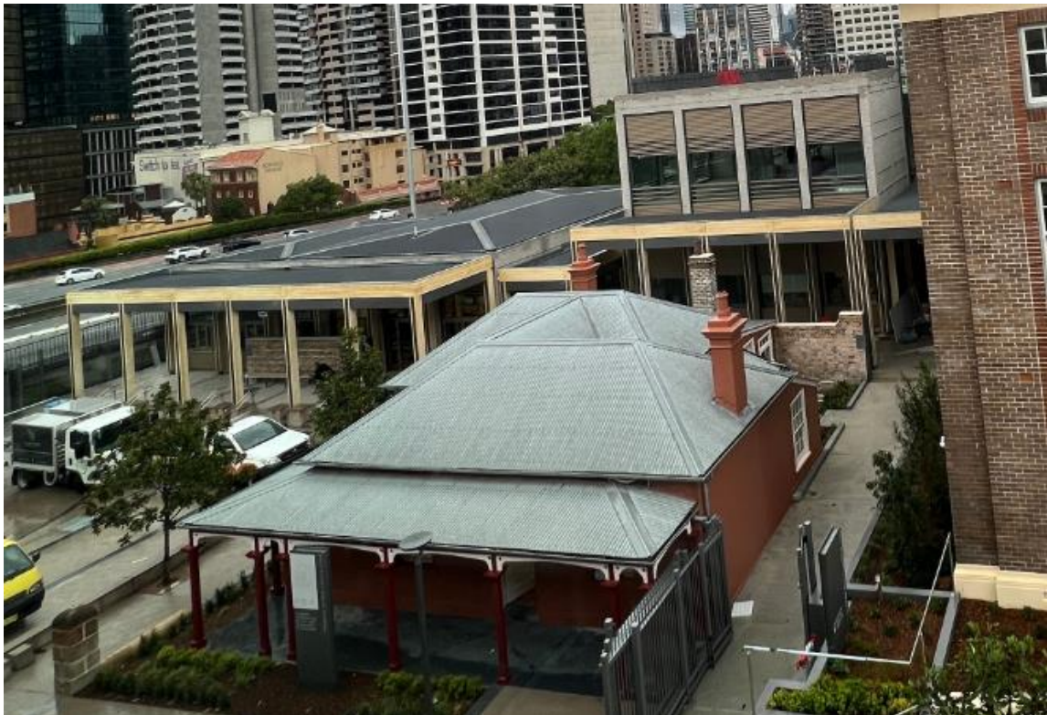
Figure 5-81: Looking South towards Building J and Building H. (Source: Curio 2023)
