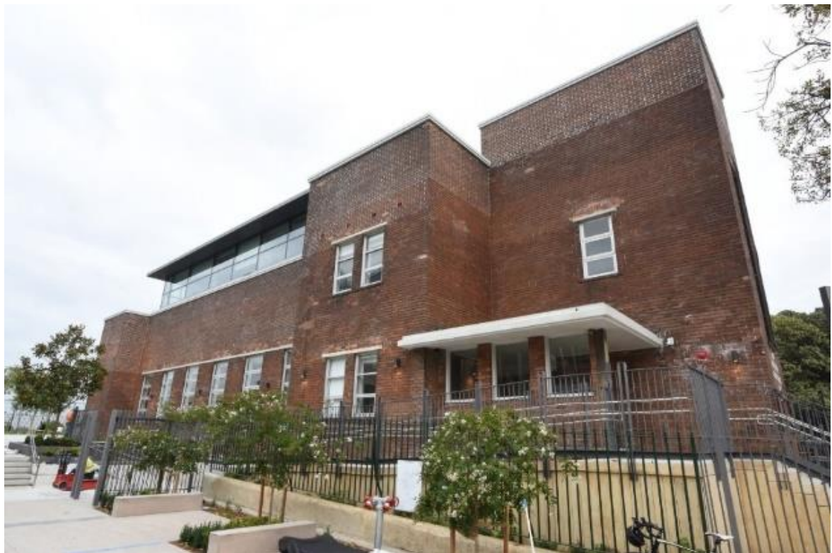
Figure 5-62: The Southern elevation of the Fort Street Public School Building (Source: Curio 2023).
