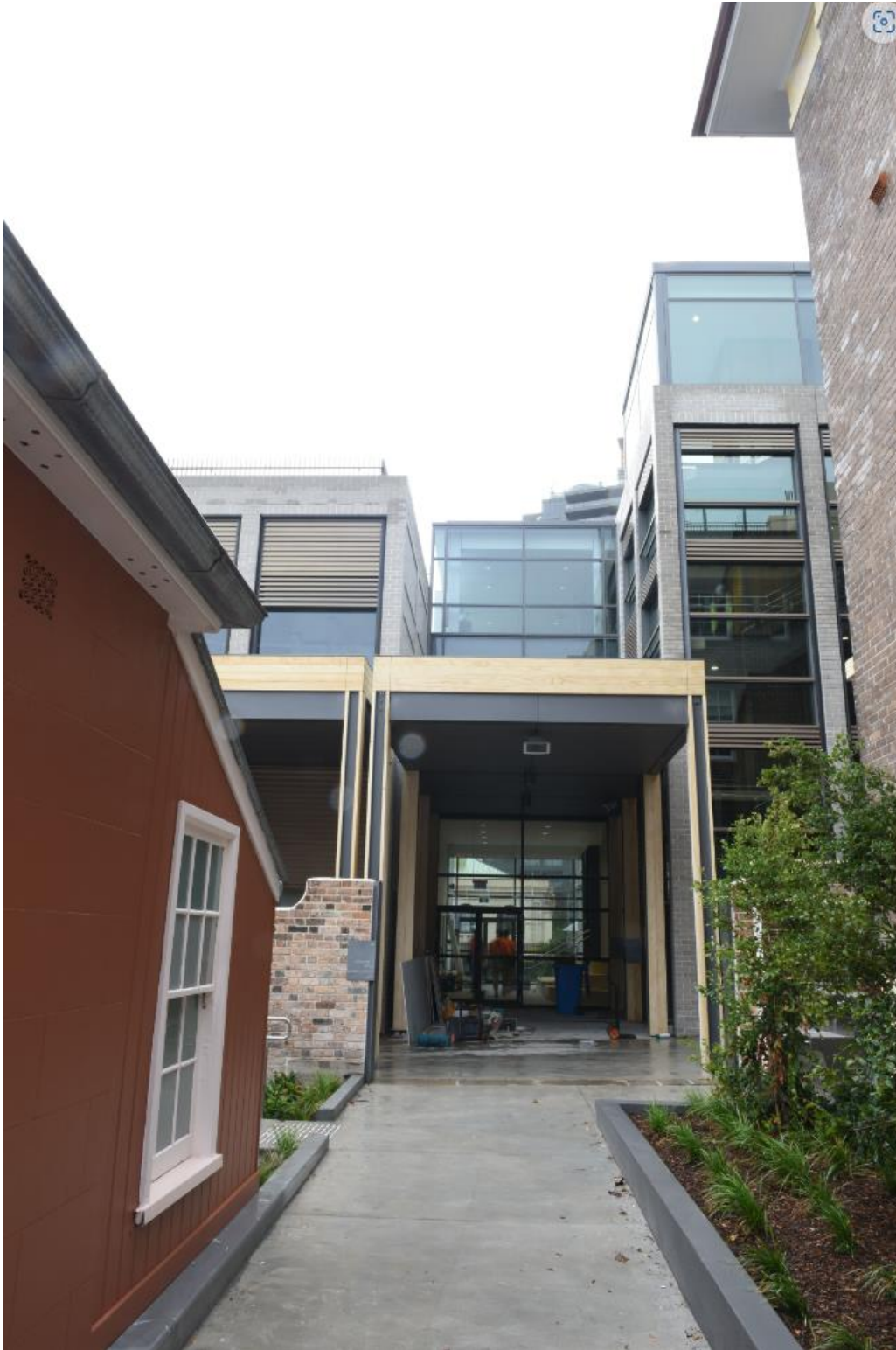
Figure 5-84: Looking north towards the Southern façade of Building J and Building H standing outside the western side of the Messenger's Cottage. (Source: Curio 2023)
