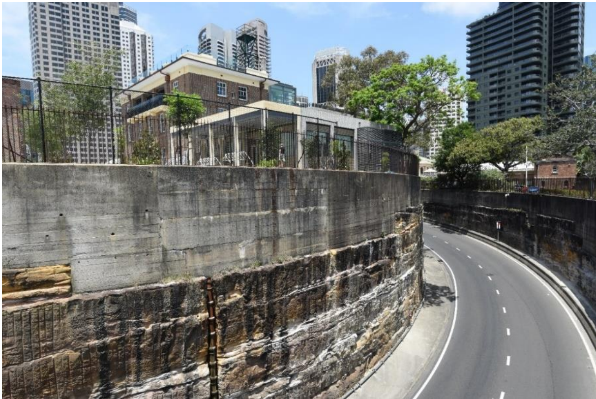
Figure 5-79: Cahill Expressway Cut, with Fort Street Public School on the left and the National Trust to the right background (Source: Curio 2023)
