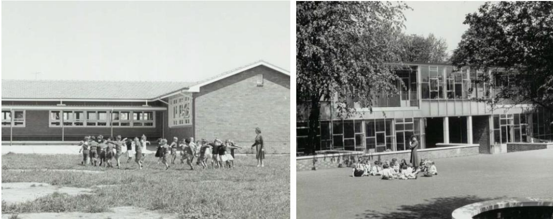
Figure 6-8: Primary school buildings from the 1950s demonstrate the tendency towards increased areas of glazing and access to sunlight in buildings: Goulburn North Public School (left) and Hornsby Public School (right). (Source: State Records digital ID 15051_a047_005925 and 15051_a047_006629, TKD 2016 Fig. 126)
