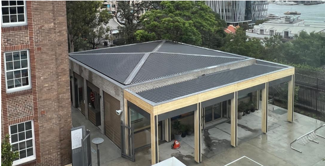
Figure 5-85: Looking directly towards Building F. (Source: Curio 2023)
