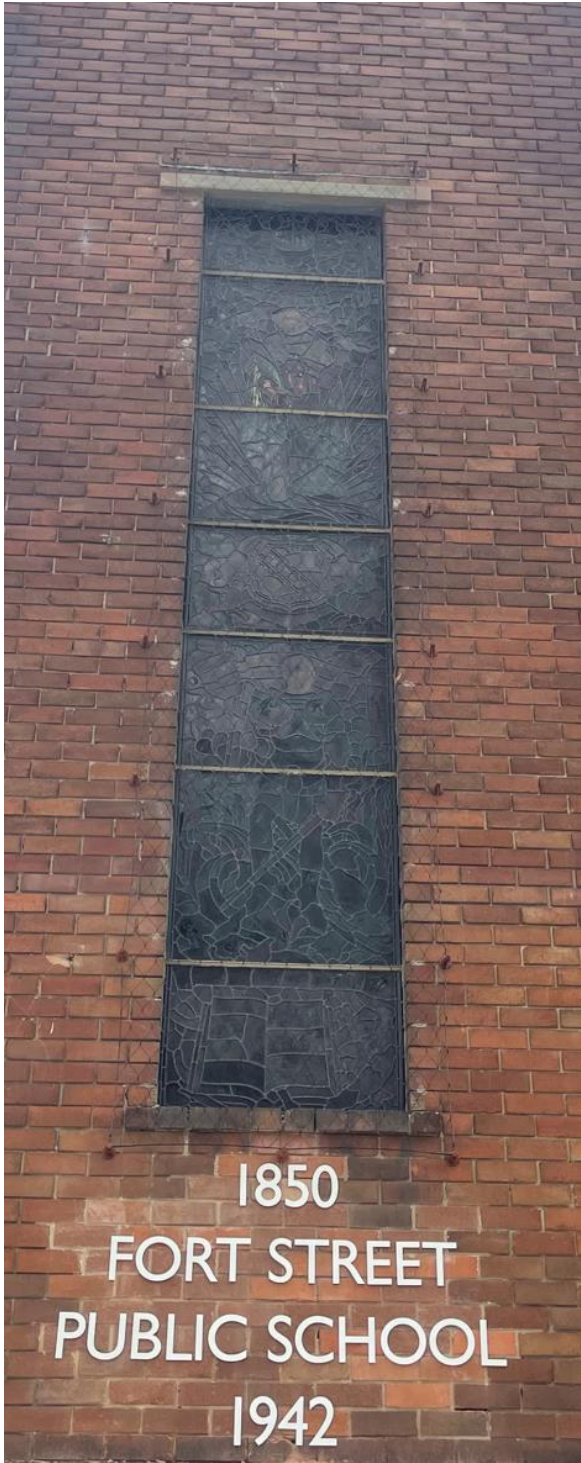
Figure 5-63 Non-Visible Tensile Protective Mesh for the Stain Glass (Source Curio 2023).
