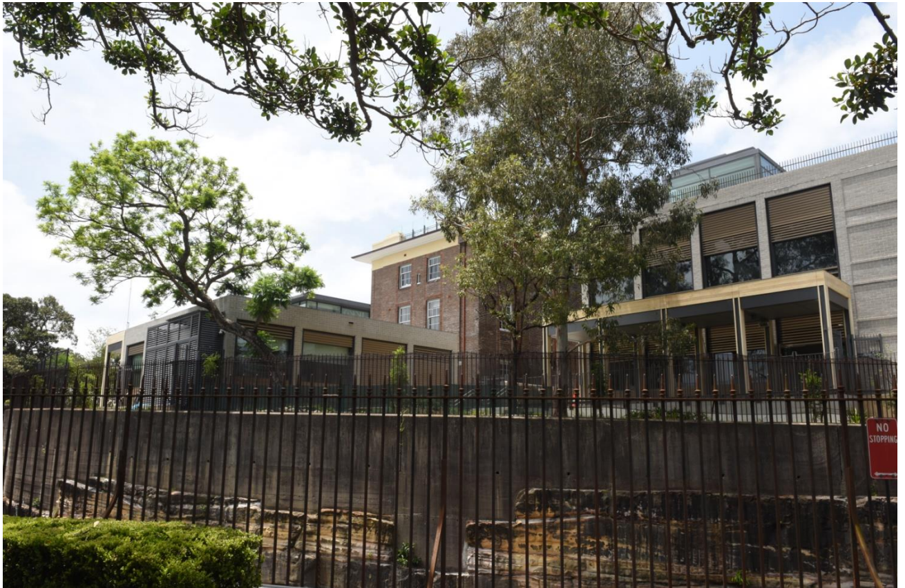
Figure 5-83: The south-western rear elevation of Buildings J and H with the Bureau of Meteorology to the rear of the photo (Source: Curio 2023)
