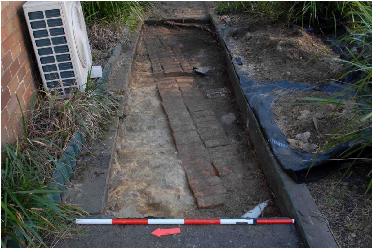
Figure 5-99 Remnant footings of Surgeons Cottage on southern side of EEC (Source: Curio 2019).
