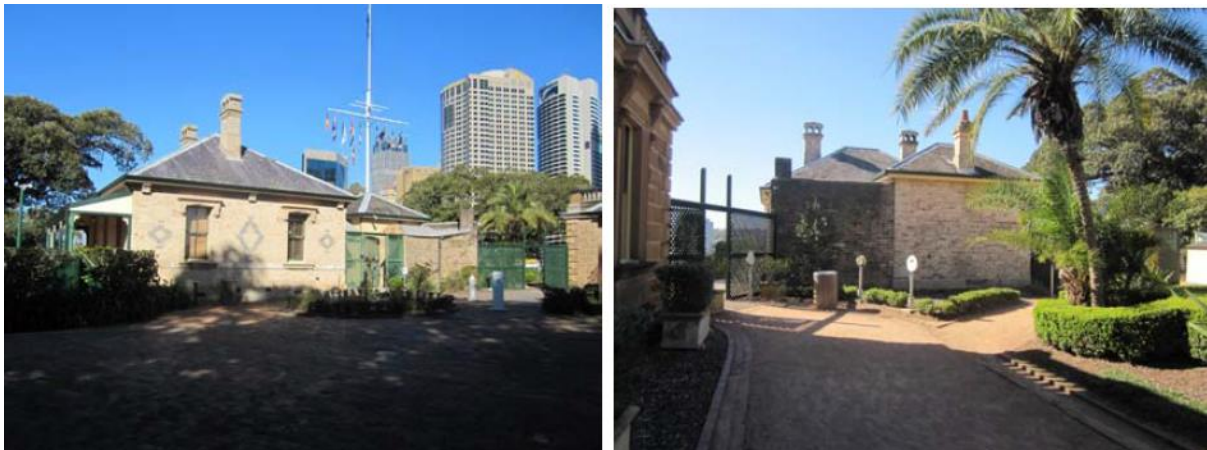
Figure 6-18: The Messenger's Cottage viewed from the west (left) and south (right), 2015 (Source: TKD 2016, Fig. 136)
