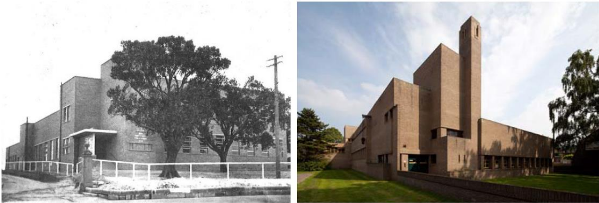
Figure 6-4: The blocky brick composition and massing of Fort Street Public School (left) is very reminiscent of buildings by Willem Dudok such as the Bavinckschool in Hilversum (right). (Sources: Building, August 1942; archinect.com – Ossip van Duivenbode photograph. TKD 2016 Fig. 122)
