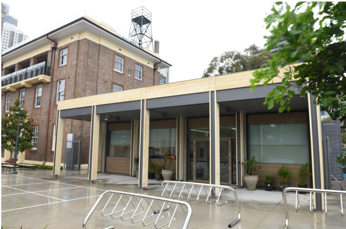
Figure 5-86: Looking towards the front elevation of building F (Source: Curio 2023)
