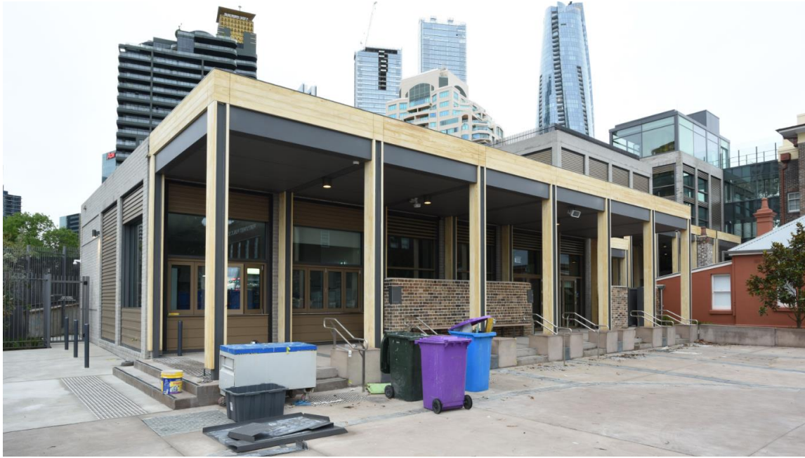
Figure 5-80: Looking South towards the front elevation of Building G (Source:Curio 2023)
