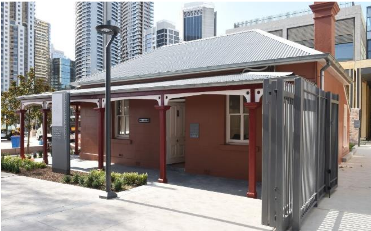
Figure 5-20: The front northern elevation of the Messengers Cottage (Source: Curio 2023)
