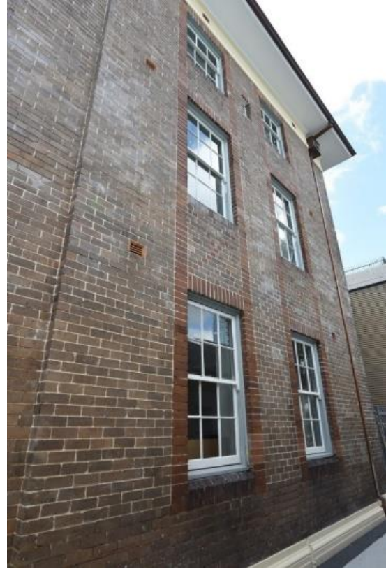
Figure 5-34: The side western elevation (Source: Curio Projects 2023)
