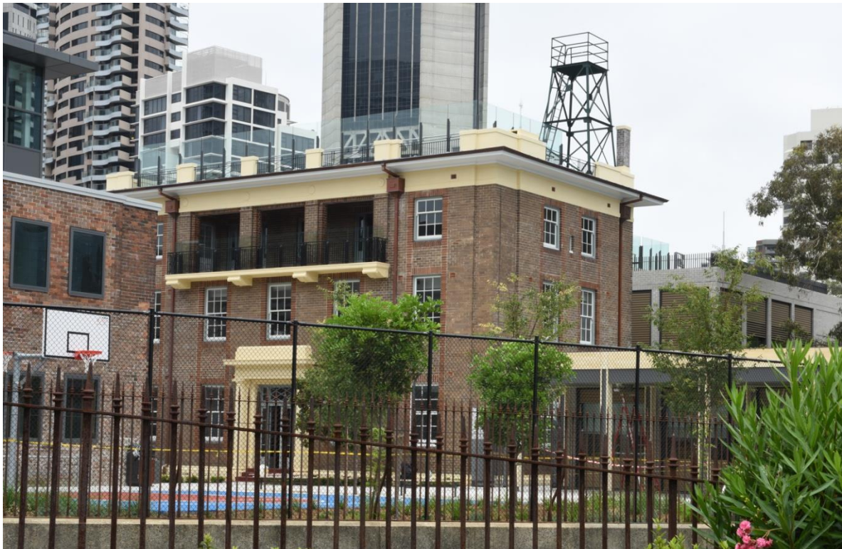
Figure 5.50 Outdoor rooftop area (Source Curio Projects 2023)
