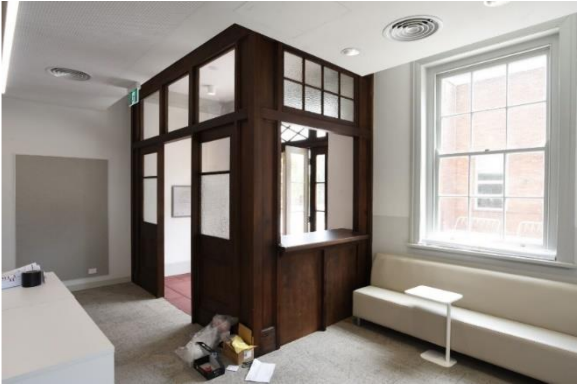
Figure 5-37: The Ground Floor Entry Vestibule (Source Curio Projects 2023)
