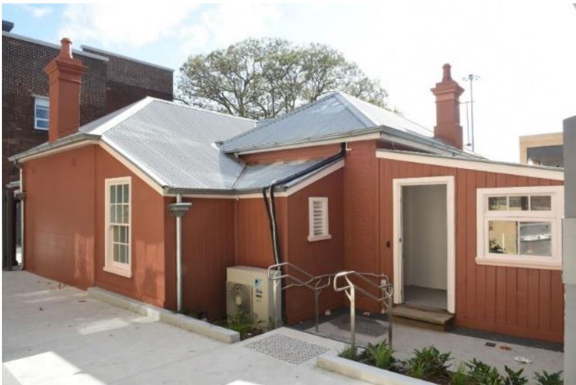
Figure 5-22: The side western elevation of the Messengers Cottage, with the later addition shed demolished (Source: Curio 2023)
