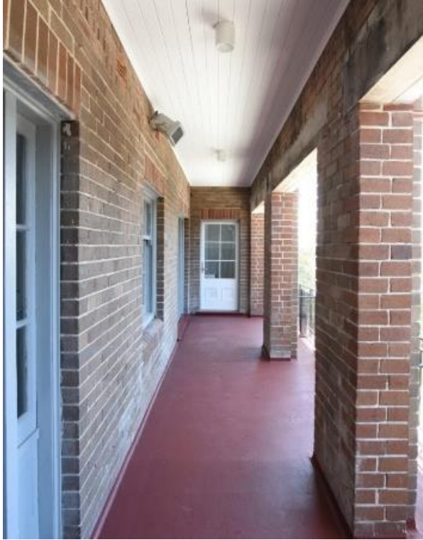
Figure 5-48: Image of outdoor covered space (balcony). (Source Curio Projects 2023)
