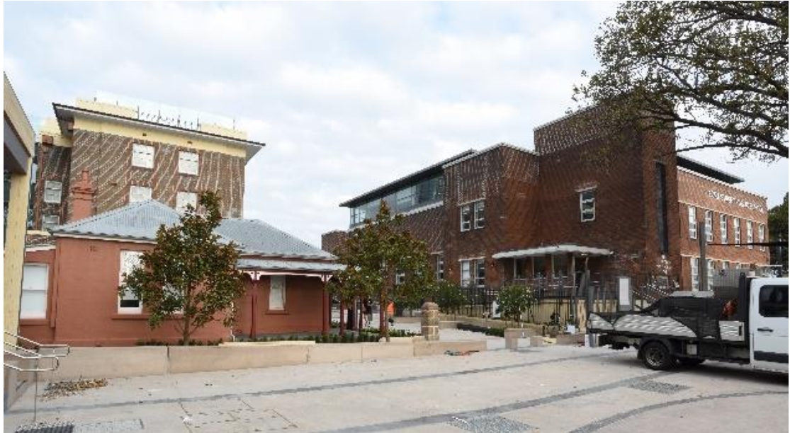
Figure 5-4: Looking West towards the Messenger's Cottage and Bureau of Meteorology. The Fort Street Public School is visible to the north. (Source: Curio: 2023)
