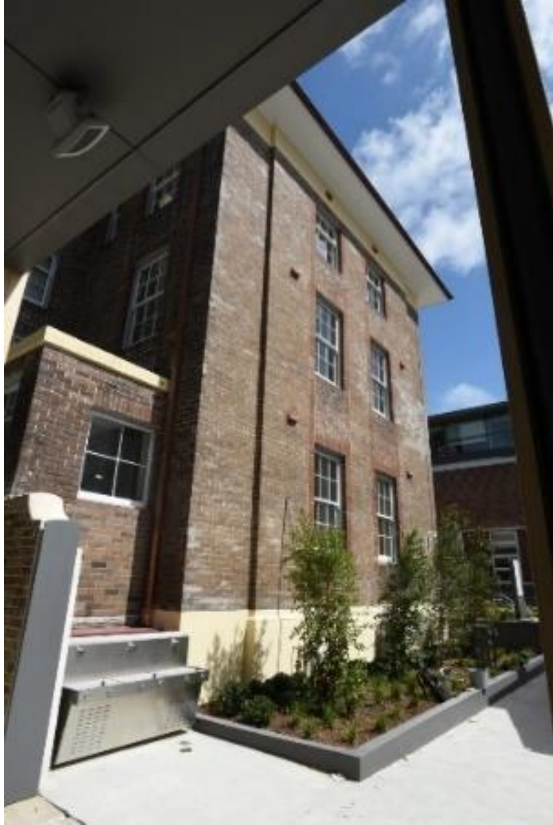
Figure 5-33: The side Eastern elevation (Source Curio Projects 2023)
