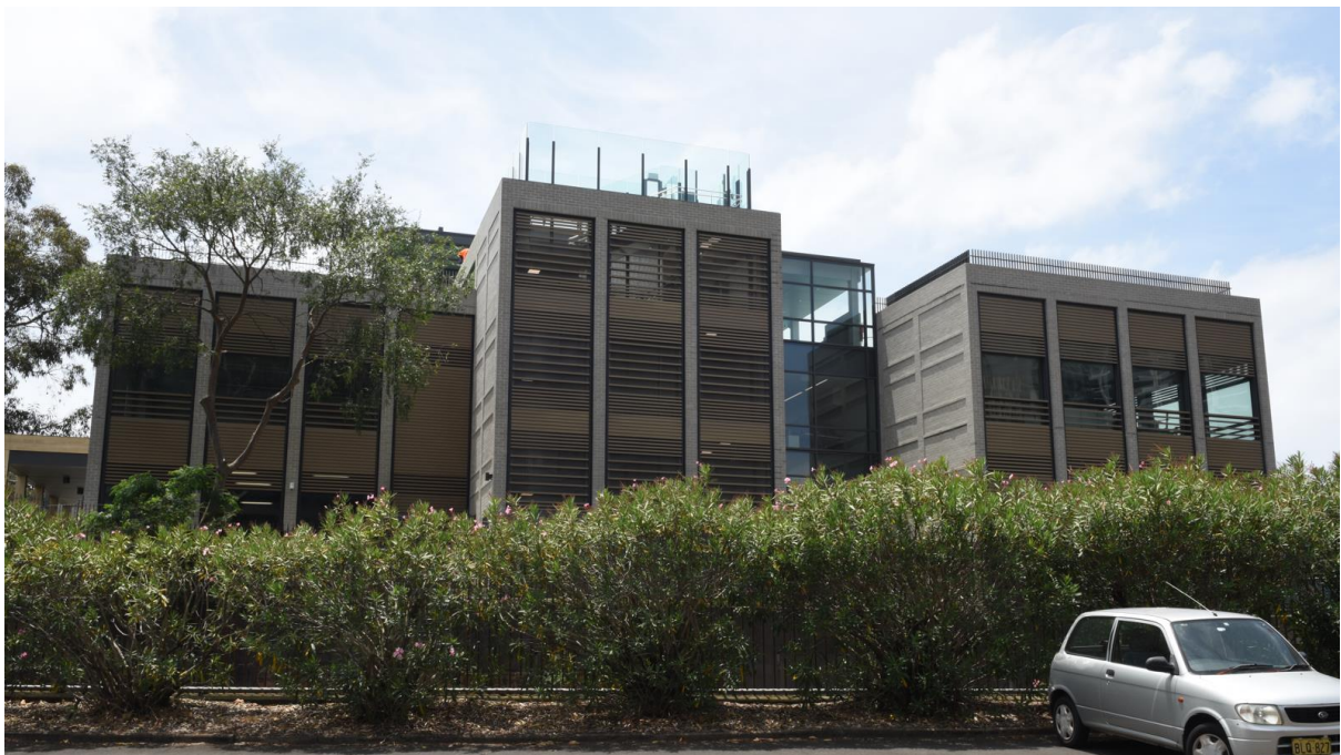
Figure 5-10 The site when viewed from the South (National Trust Carpark) is not dissimilar to the previous site constraints in terms of impacting on views to and from the National Trust to Observatory Hill. See Figure 5.11, on the following page, which shows the former view from the National Trust site for comparison.
