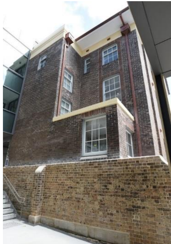
Figure 5-36: The Eastern Elevation of the Building
