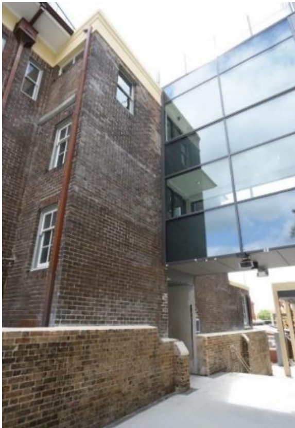
Figure 5-35: The Southern Elevation of the Bureau of Meteorology
