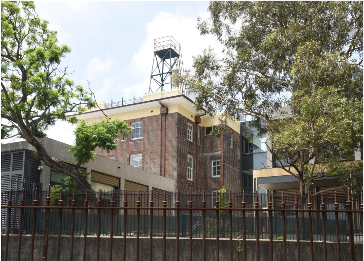
Figure: 5- 51 View of the Rooftop Weather Station, copper downpipes and contemporary bridge connection to Building J (to the right).
