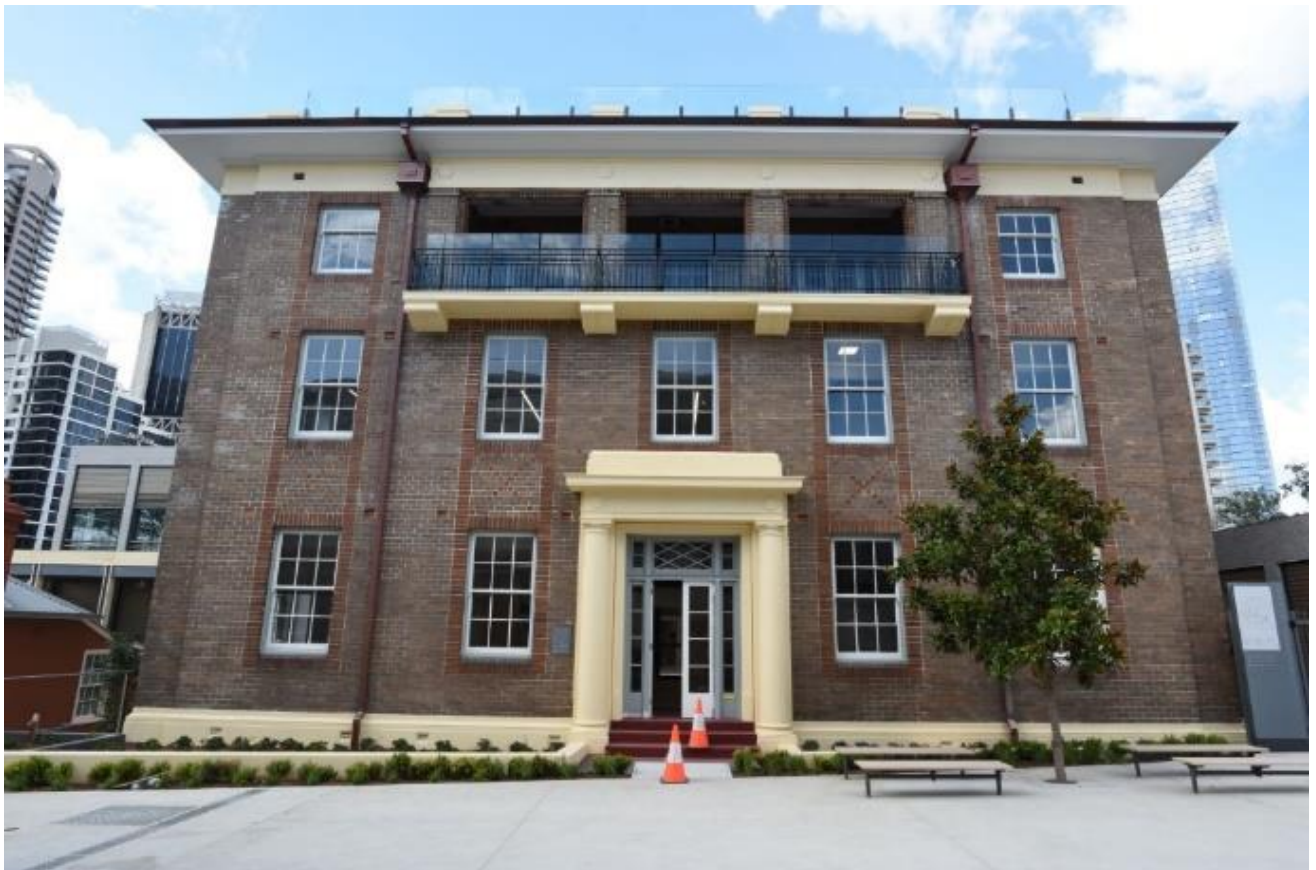
Figure 5-32: The Front Northern elevation of the conserved Bureau of Meteorology (Source: Curio 2023)
