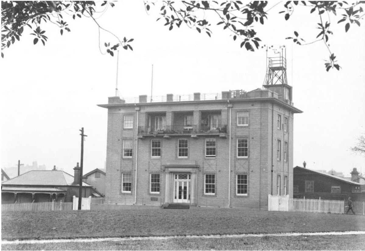
Figure 4-20: Bureau of Meteorology, photographed circa 1932. The recessed balcony of the residential apartment appears to have also served as a drying area. The building directly addressed Observatory Hill Park. (Source: TKD 2016: Fig 36).
