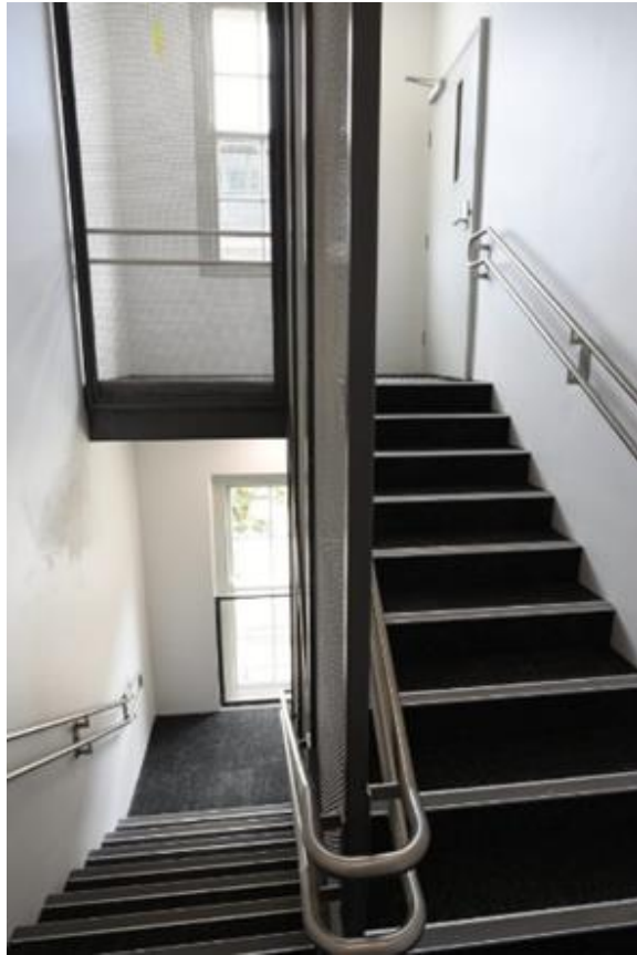
Figure 5-44: The stair at first-floor level. (Source Curio Projects 2023)
