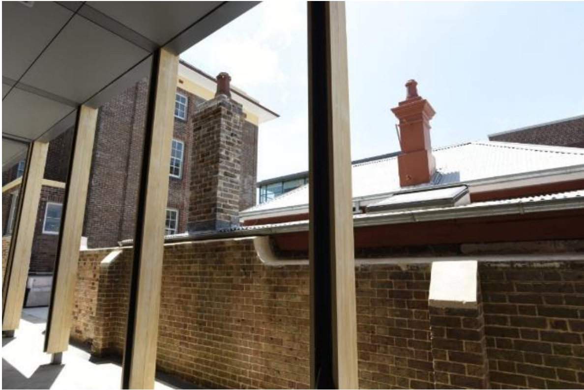
Figure 5-23: The rear southern elevation of the Messengers Cottage, showing the reconstructed chimney (unpainted brick chimney) and reconstructed section of boundary wall (to the left). (Source: Curio 2023).
