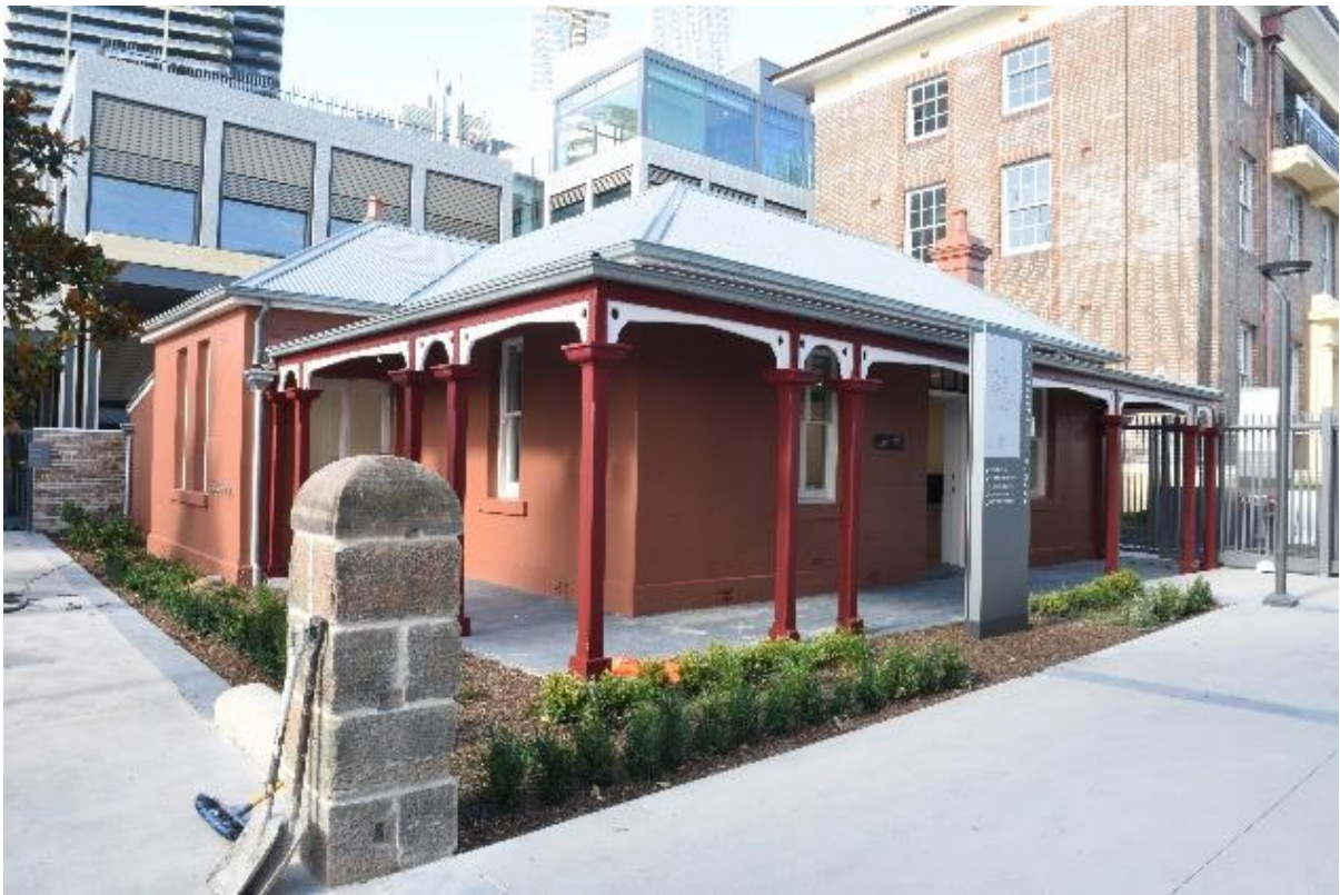
Figure 5-14: Looking South towards the Messengers Cottage and the relocated sandstone pier (Source: Curio, 2023)
