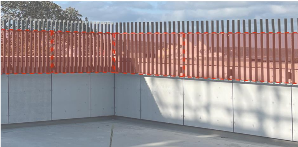
Figure 5: The proposed tensile mesh to be located behind the metal balustrade of building J and building H. Source: FJC Studio
