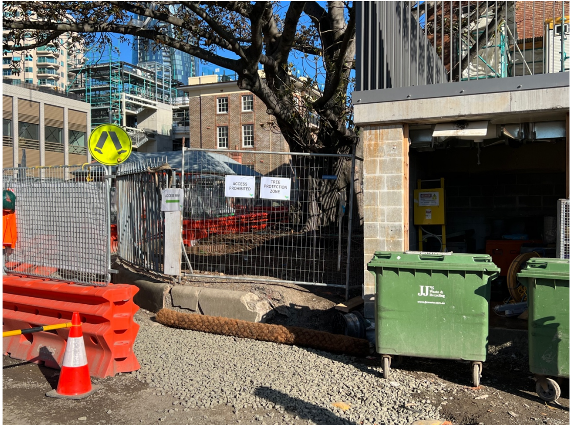
Figure 16 Site laydown area and in-gutter sediment control
