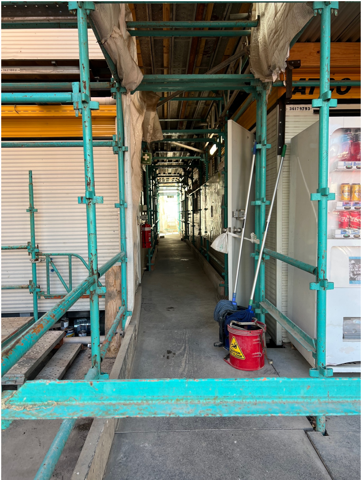
Figure 26 Site compound sheds – materials storage in bottom left
