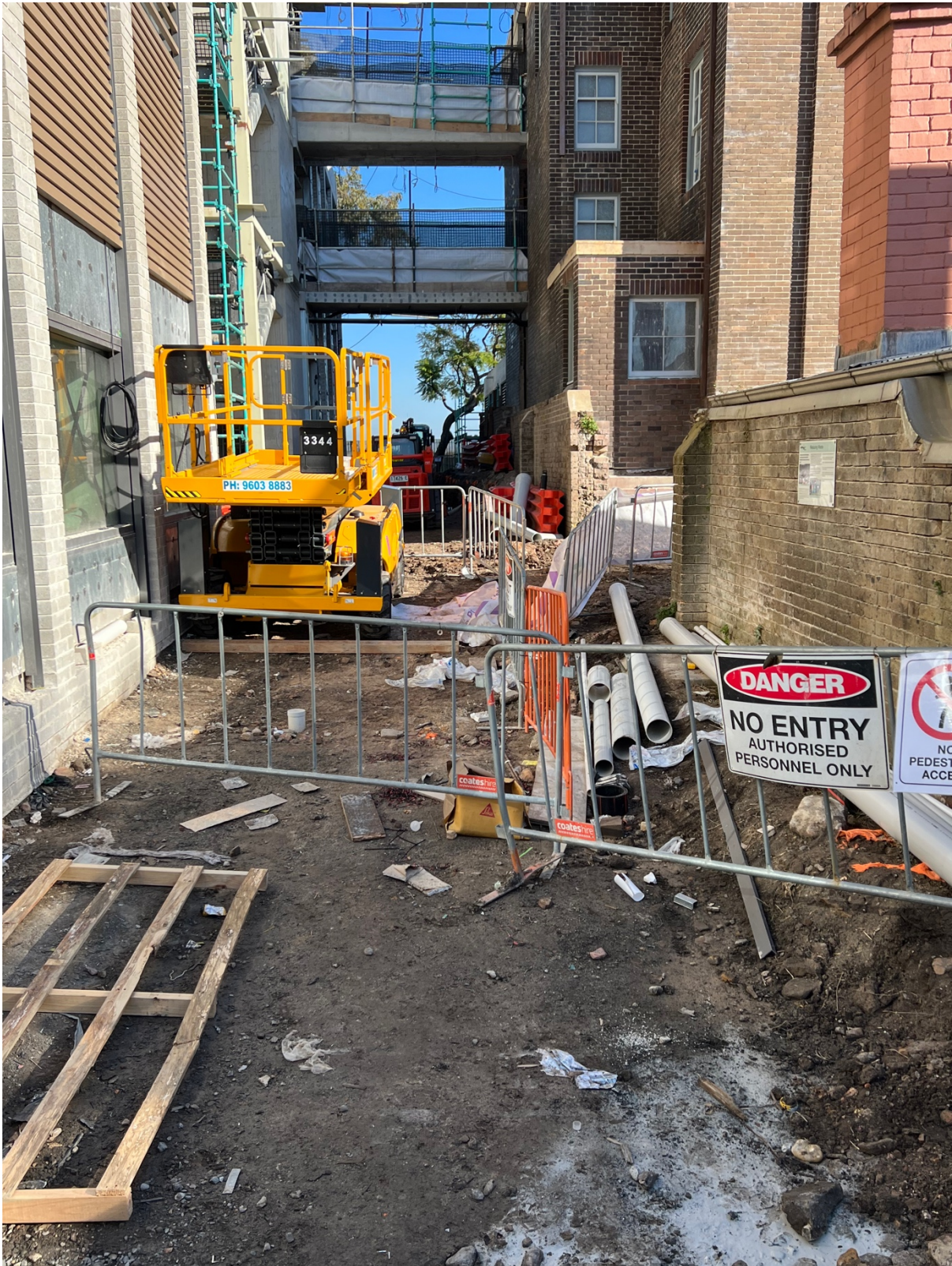
Figure 31 Mobile plant and Heritage Boundary Wall – showing exclusion zone
