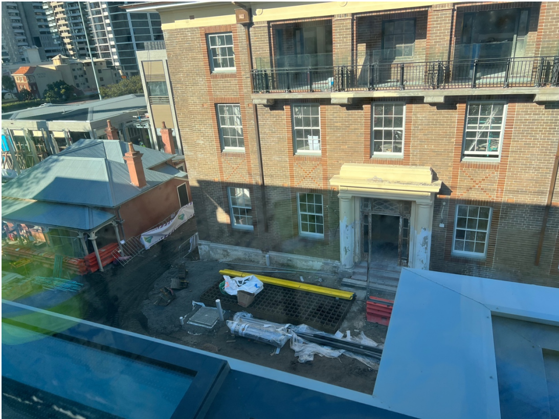
Figure 22 Laydown area front of Met Building
