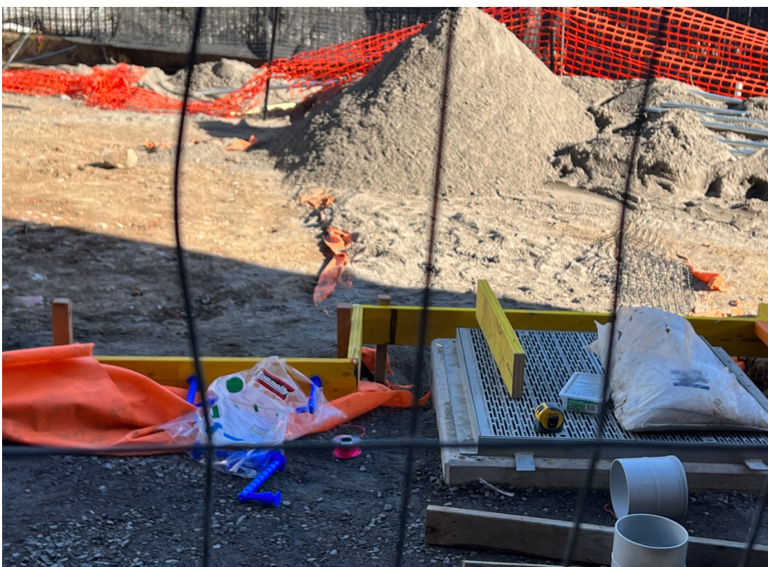
Figure 21 Site landscaping works in progress
