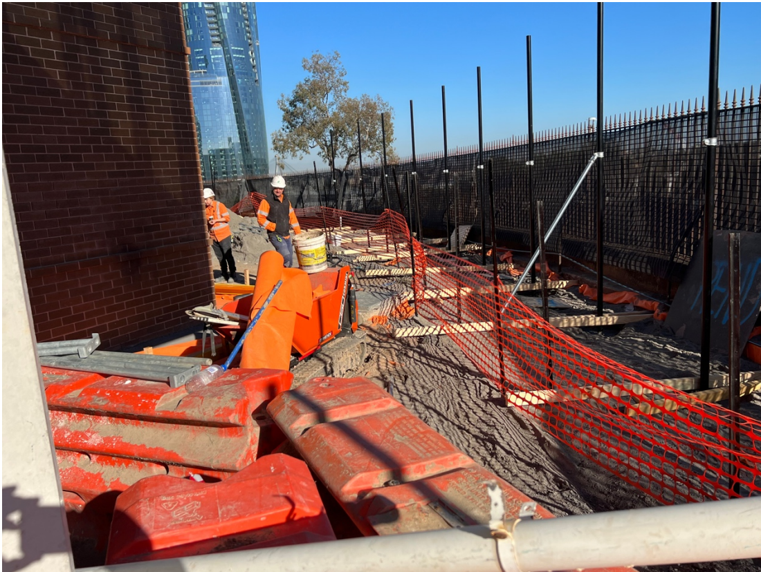
Figure 20 Site landscaping works in progress
