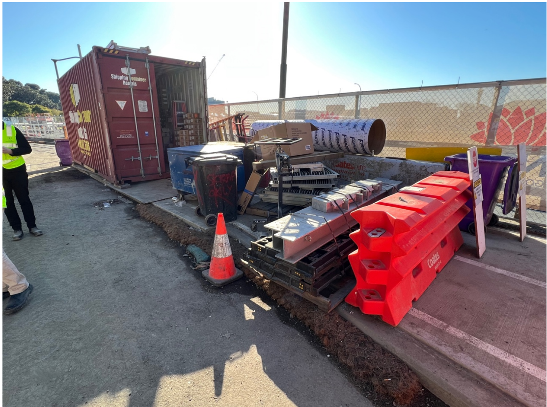
Figure 16 Site laydown area and in-gutter sediment control
