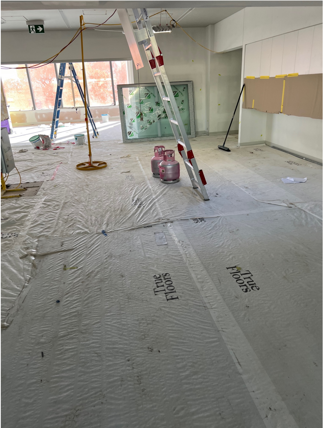
Figure 24 Works internal to FSPS building
