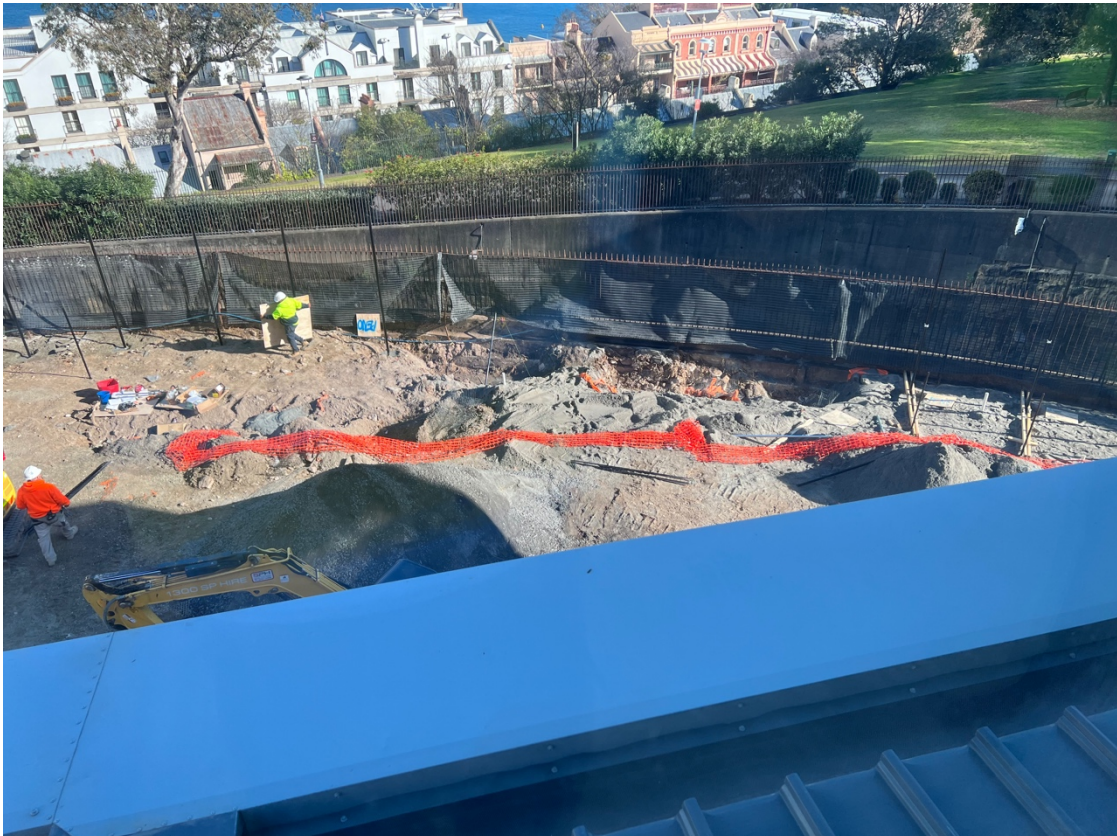
Figure 23 Landscaping works in progress
