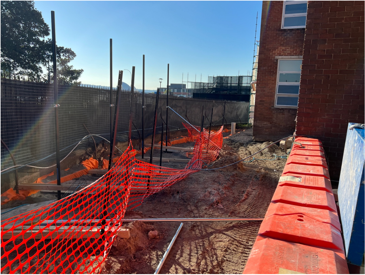
Figure 13 Site landscaping works in progress
