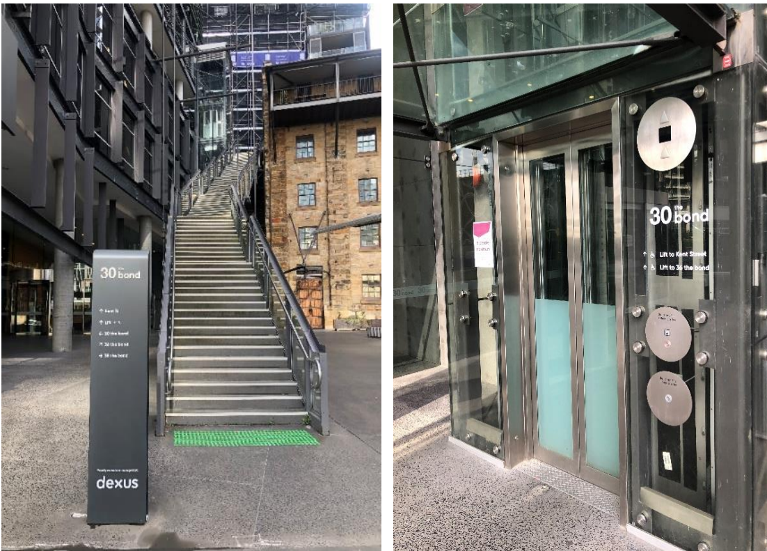
Figure 14: Stair (left) and lift (right) access from Hickson St to Kent St
