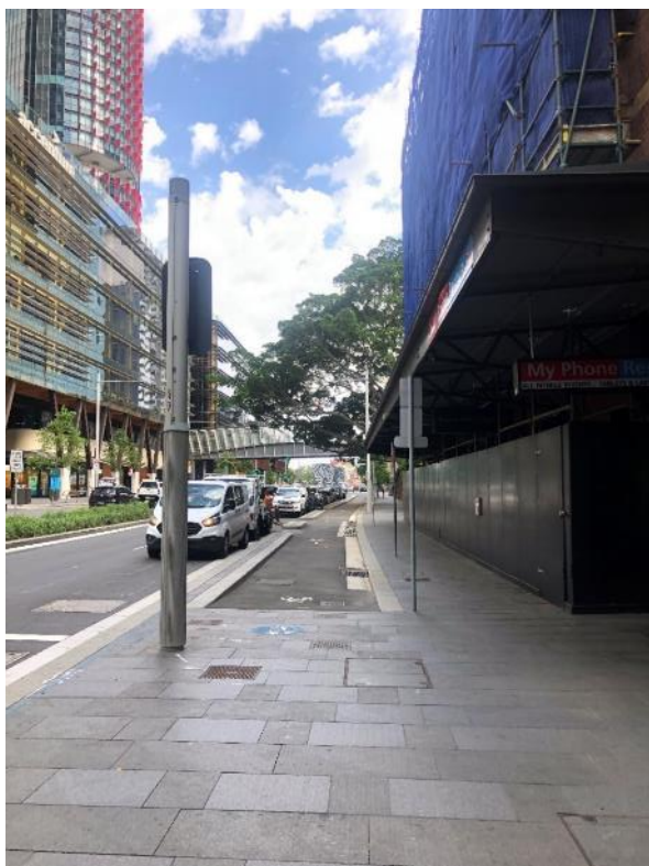
Figure 12: Dedicated one-way southbound cycleway connecting into a shared path along Hickson Road
