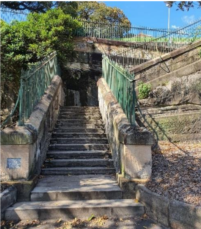
Figure 29: Steps connecting Argyle Street to Watson Road
