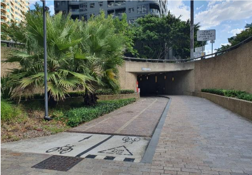
Figure 21: Wayfinding at underpass directing to Sydney Harbour Bridge
