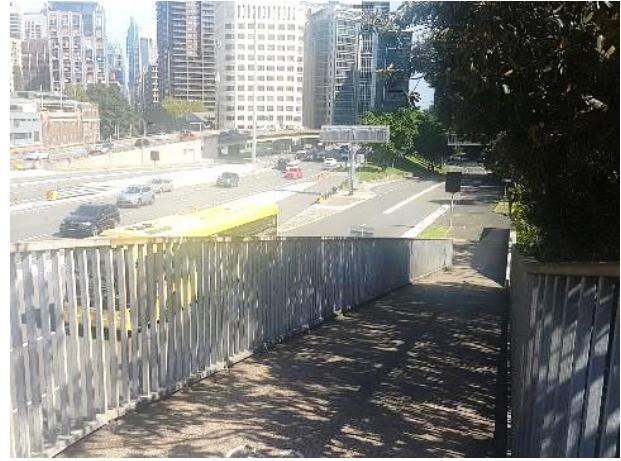
Figure 6: Shared path overpass on the south-east side of the school
