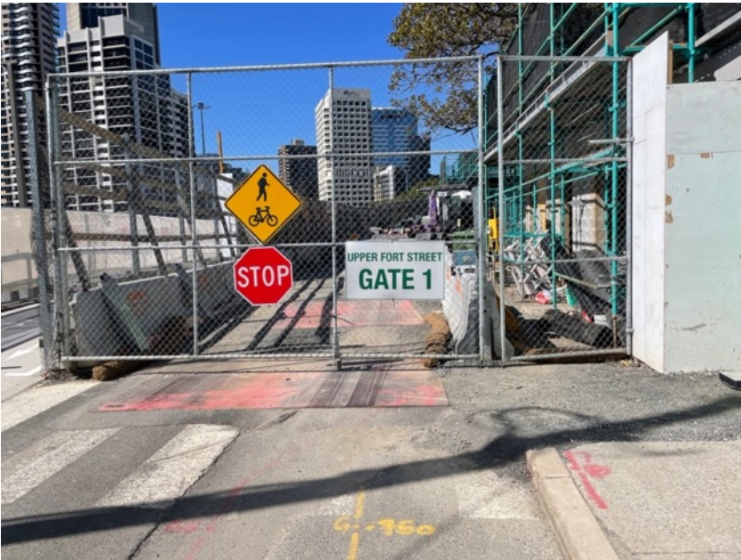
Figure 6 Upper Fort Street Gate 1
