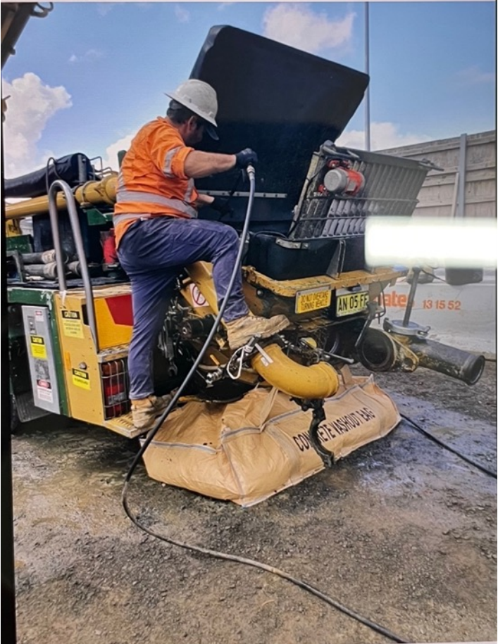
Figure 12 Concrete washout bag and disposal
