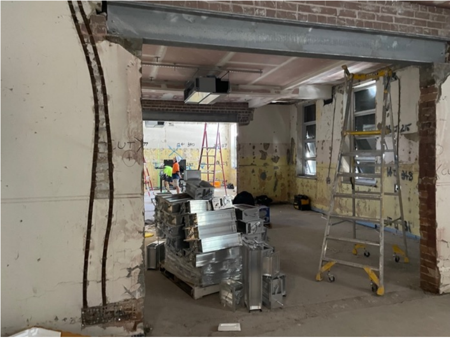
Figure 7 Internal building fit out
