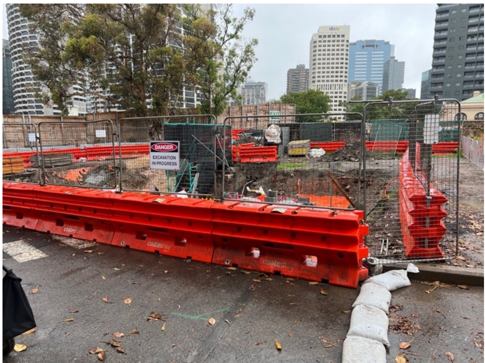
Figure 24 Excavation zone, safety fence and warning signage
