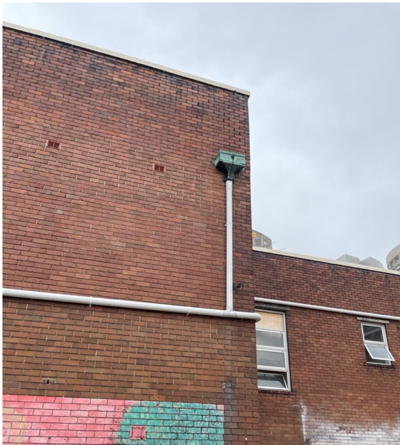
Figure 12 Temporary stormwater installation to control runoff
