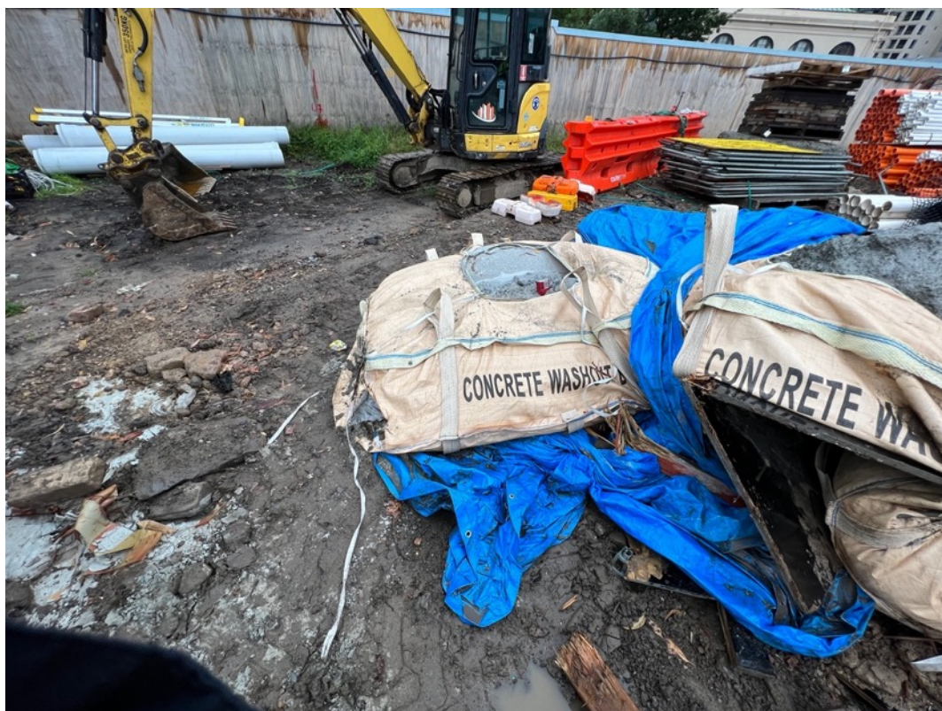
Figure 17 Concrete washout bags ready for disposal
