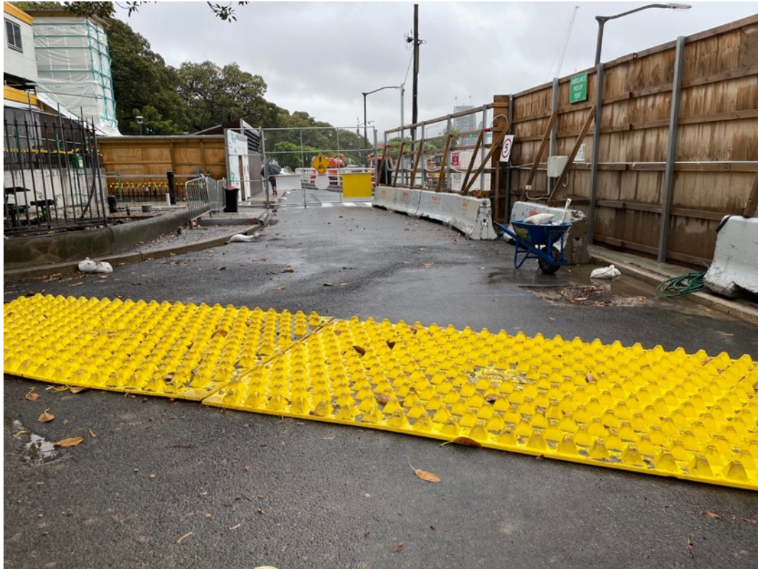
Figure 11 Rumble grid in place looking north
