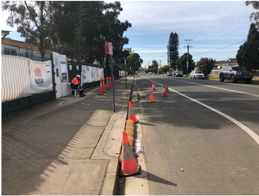
Figure 7 Protection of stormwater drains on public road
