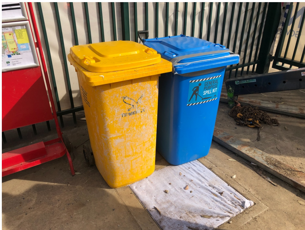
Figure 2 Spill kits and stormwater drain protection
