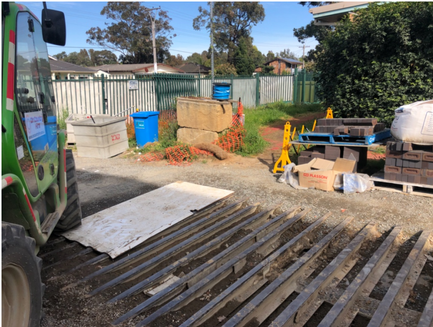
Figure 5 Entry/ exit point to site with rumble grid
