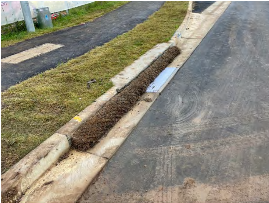
Figure 7 ERSed controls in place to protect stormwater drains
