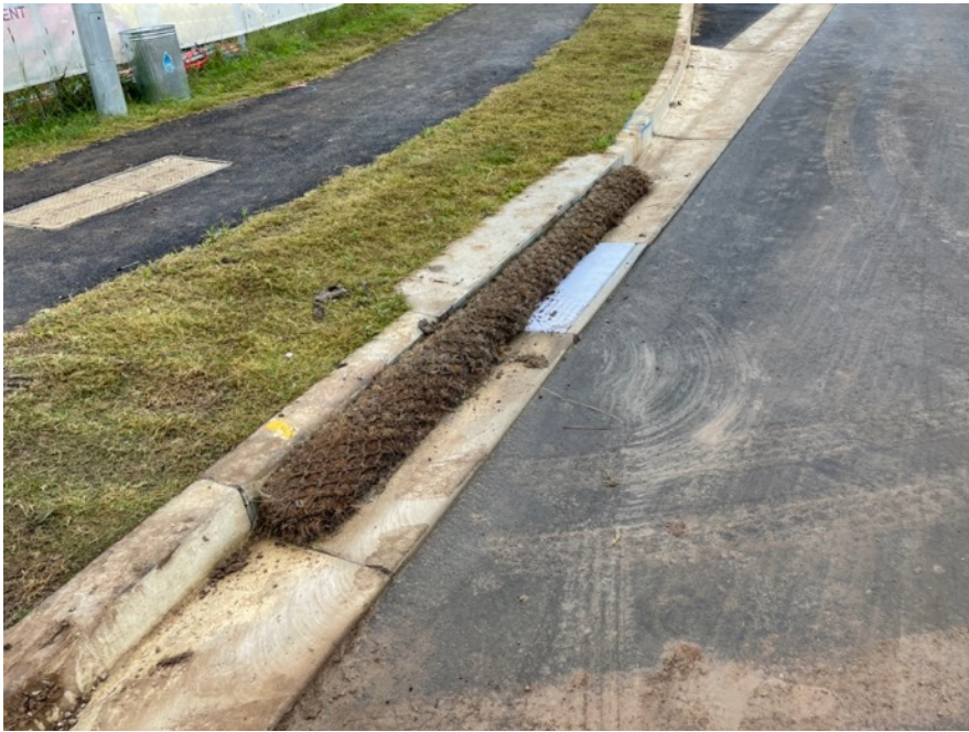
Figure 7 ERSERD controls in place to protect stormwater drains
