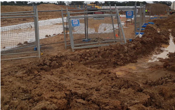
Photo 7: Rectification of bunding for sediment basin
