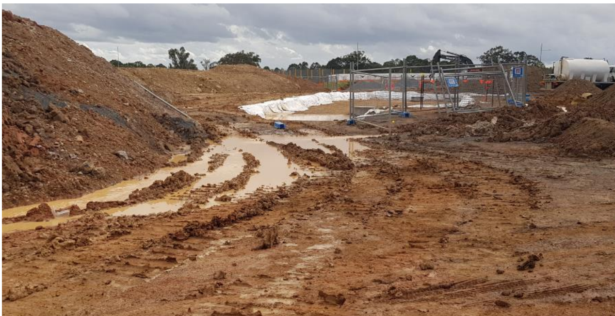
Photo 4: Untested / untreated pumped water bypassing the sediment basin
