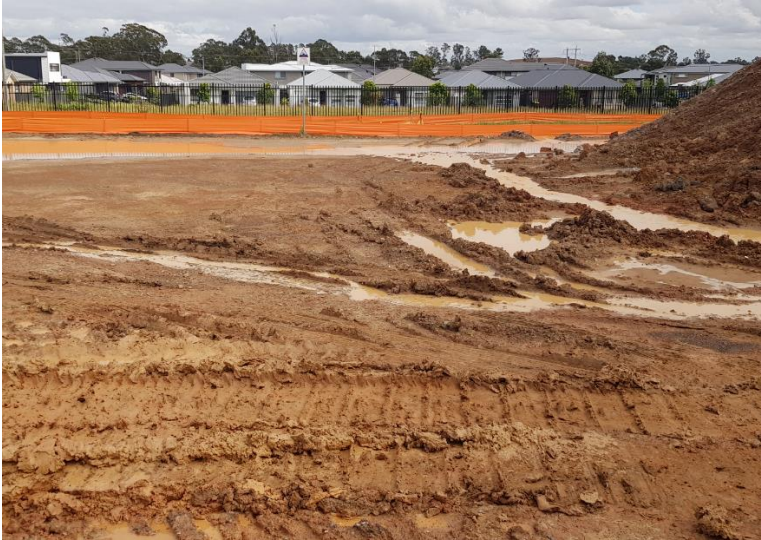
Photo 6: Untested / untreated pumped water flowing to boundary sediment fence
