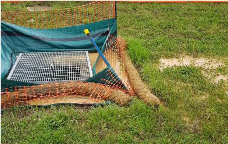
Photo 6: Untested / untreated pumped water flowing to off-site stormwater
