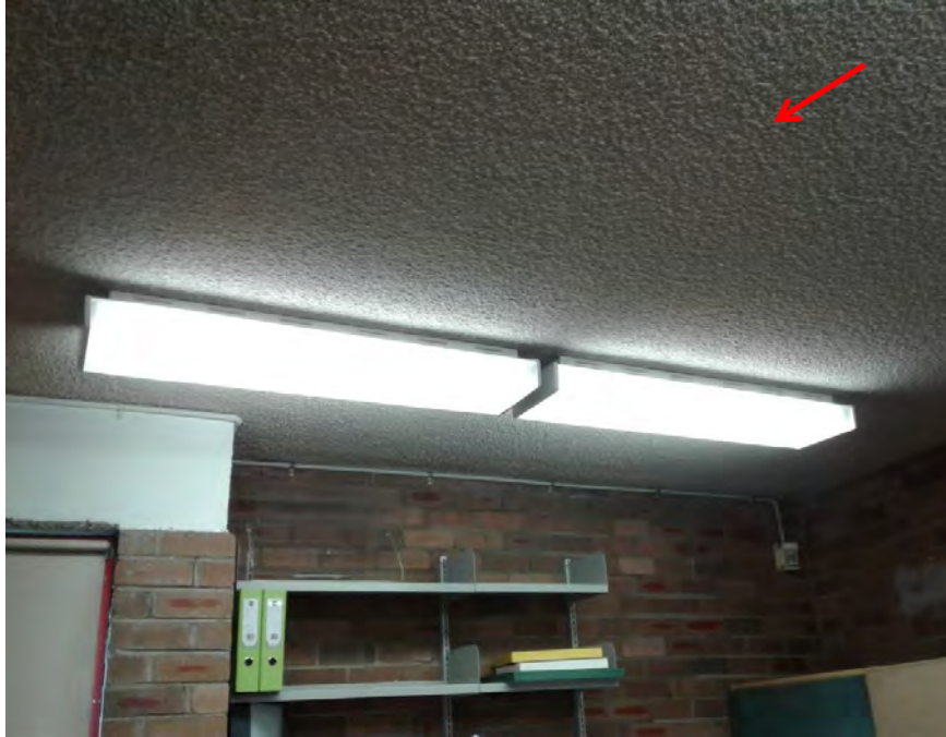
Photograph 5: B00A - R0011, Interior, Ceiling structure, Vermiculite, no asbestos detected by analysis.
