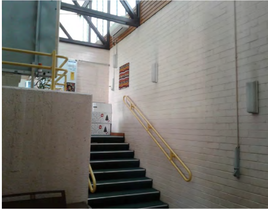
Photograph 17: B00A - R1017, Interior, -, -, nil hazardous materials identified.
