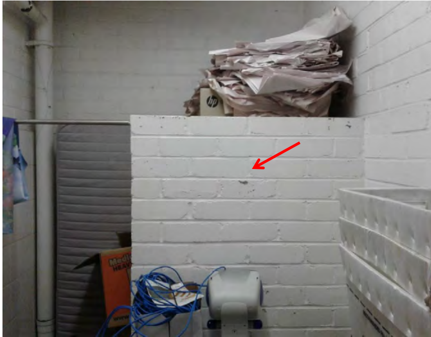
Photograph 11: B00A - R0023, Interior, Brick walls, Beige paint, non-lead paint ( \leq 0.1\% lead w/w).
