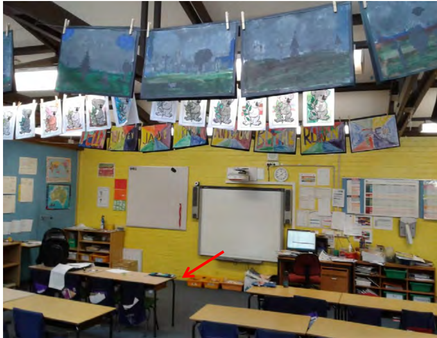
Photograph 28: B00B - R1011, Interior, Timber skirting board near flooring, Yellow Paint, non-lead paint ( \leq 0.1\% lead w/w).
