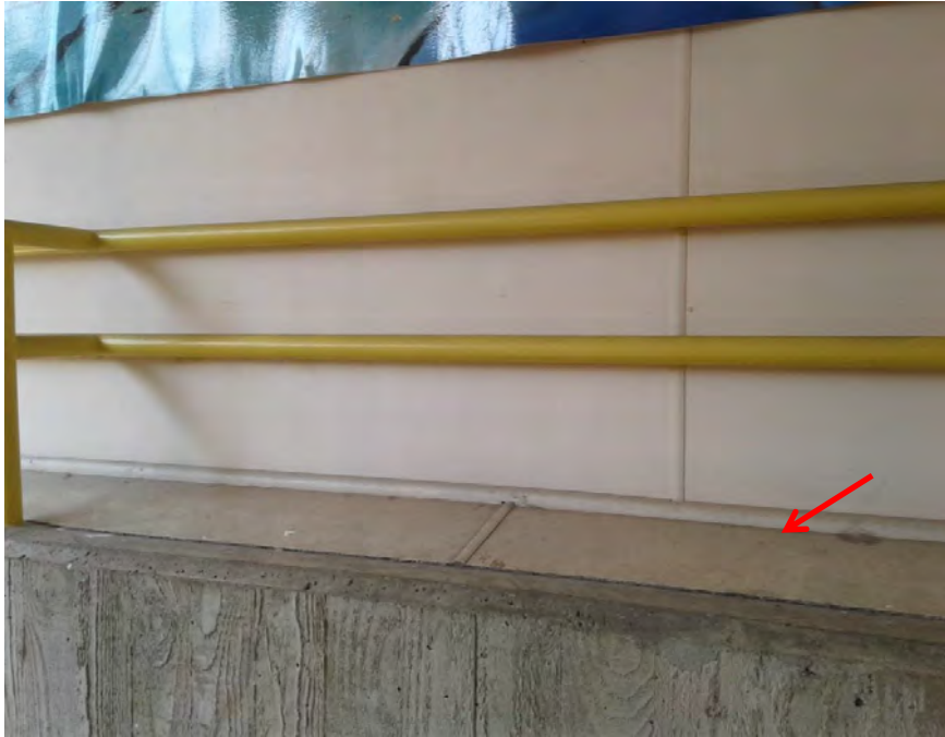
Photograph 22: B00B - R0025, Interior, FCS sheeting on wall, FCS sheeting, no asbestos detected by analysis.
