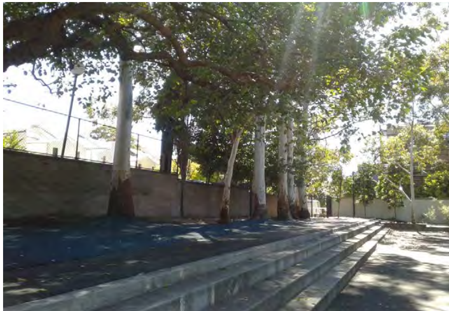
Photograph 6 - Far northern portion of site . Elevated area with rubber safety seal material covering majority of area.
