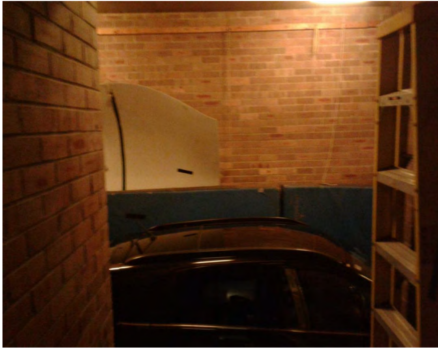
Photograph 1: B00A - R0002, Interior, Garage walls, Brick, nil hazardous materials identified.
