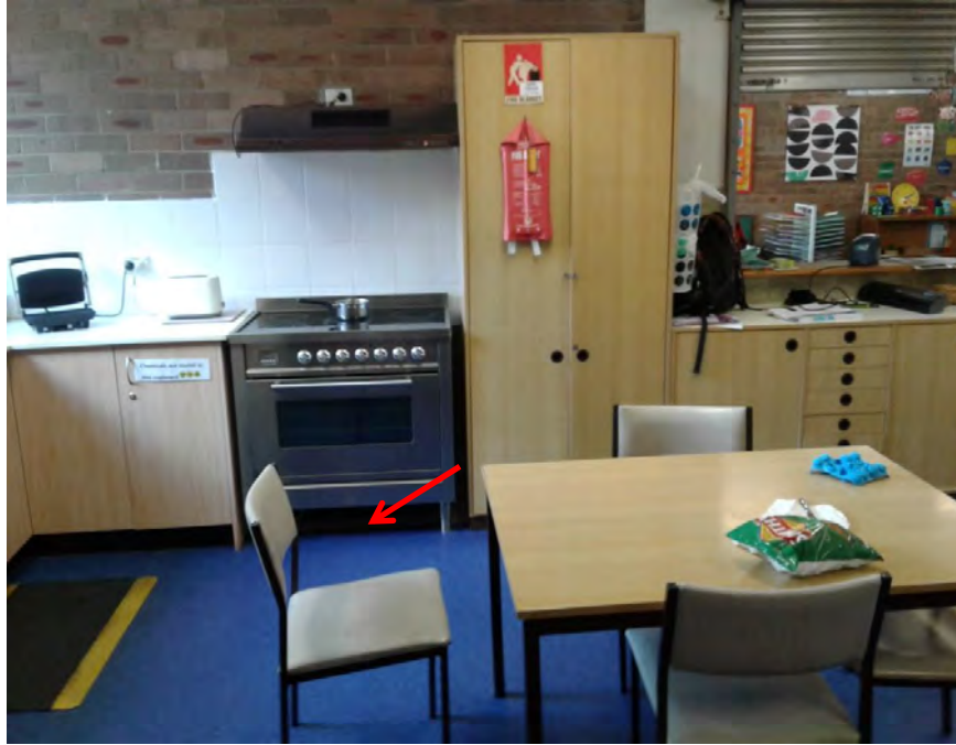
Photograph 34: B00C - R0006, Interior, Flooring material, Vinyl tiles, no asbestos detected by analysis.
