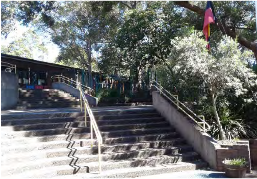
Photograph 3 - Central portion of site
