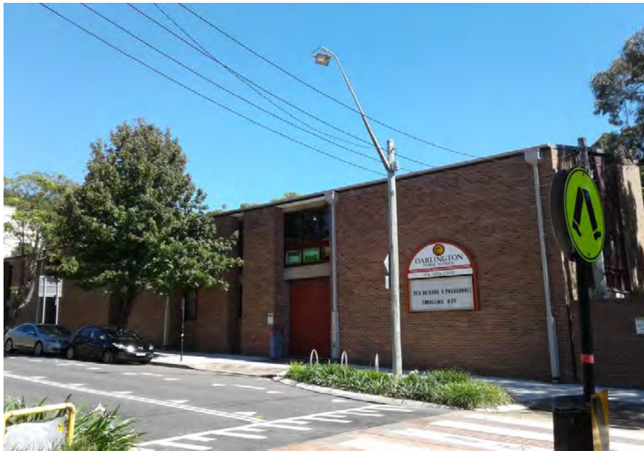
Photograph 1 - South facing school building in south western portion of site with Abercrombie Street in foreground
