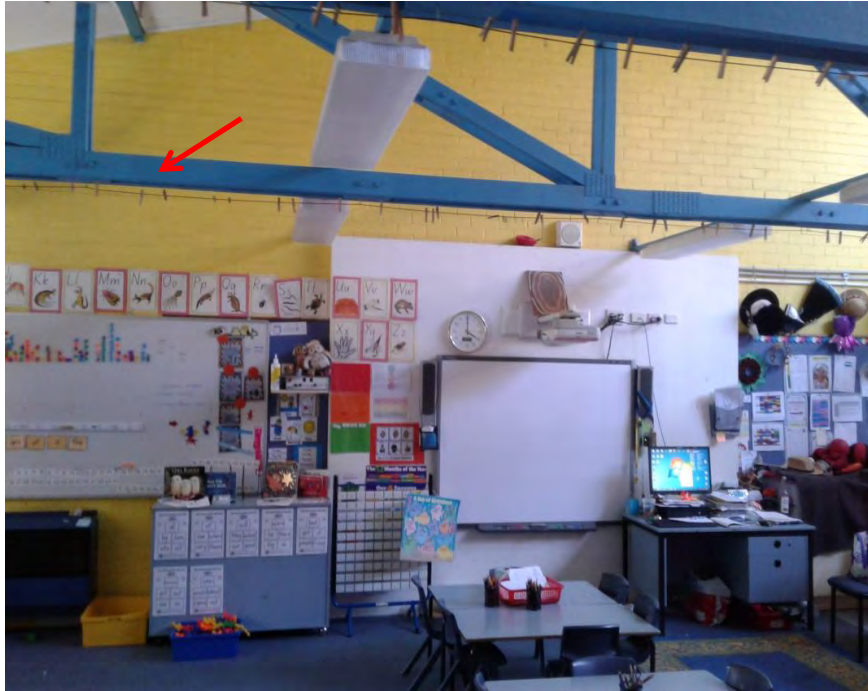
Photograph 20: B00B - R0020, Interior, Timber rafters, Blue paint, non-lead paint ( \leq 0.1\% lead w/w).
