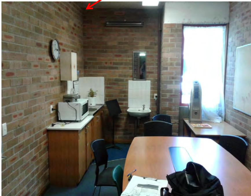
Photograph 2: B00A - R0006, Interior, Ceiling structure, Vermiculite, no asbestos detected by analysis.
