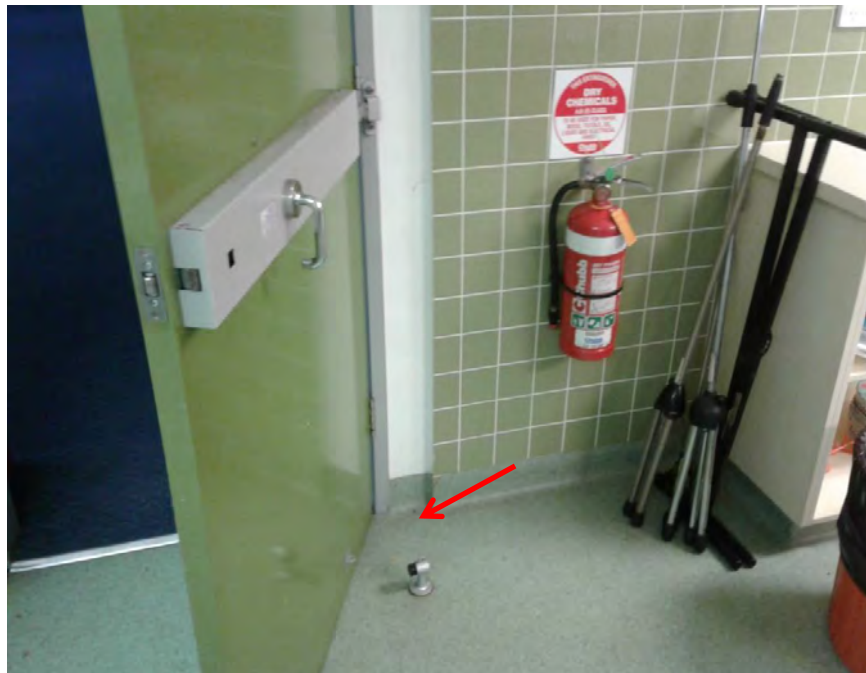
Photograph 12: B00A - R0025, Interior, Flooring material, Vinyl tiles, no asbestos detected by analysis.
