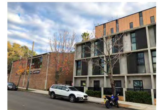
View to Sydney University Student Accommodation - from Abercrombie Street
