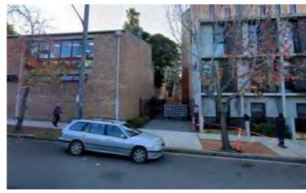
Existing Photo of Abercrombie Student Accommodation in Abercrombie Street
