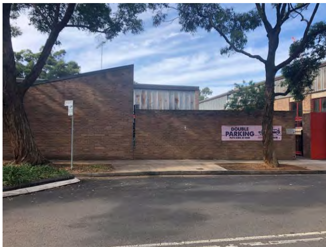
Figure 10 Photo of Existing School (facing east from Golden Grove Street)
