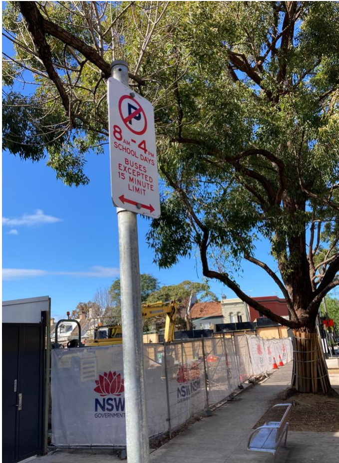
Figure 18 Parking restriction at Golden Grove Street Drop-off and Pick-up Zone
