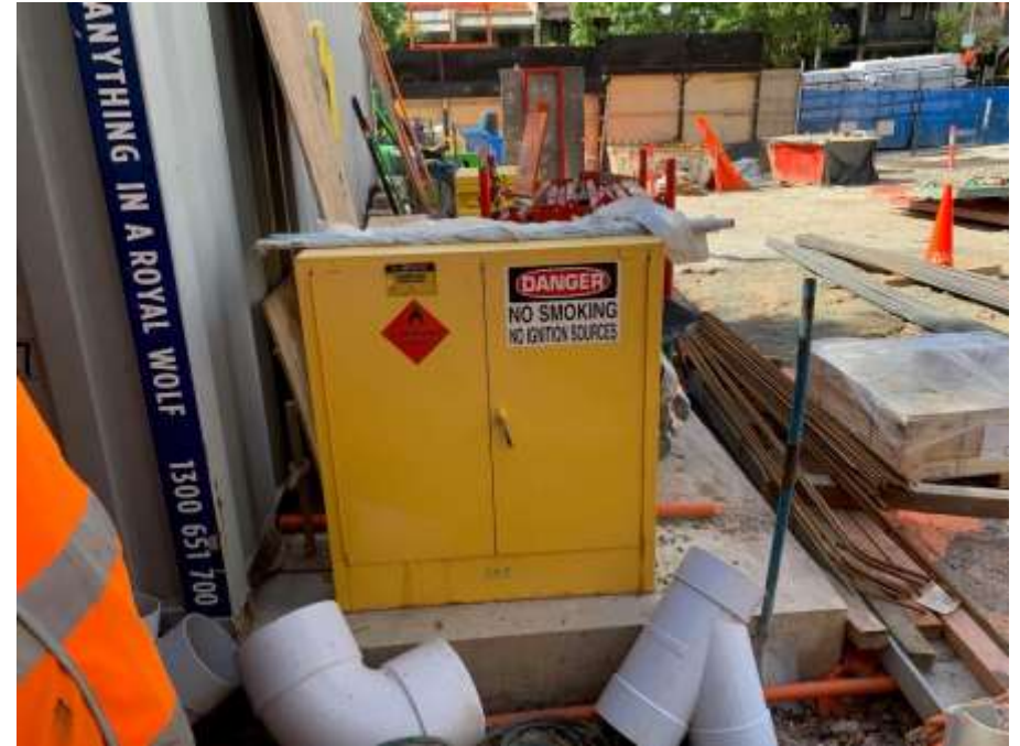
Photo 4: Chemical Storage Container
