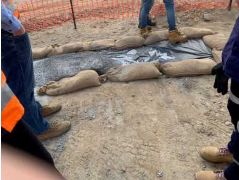
Photo 5: Bunded and sealed concrete washout area
