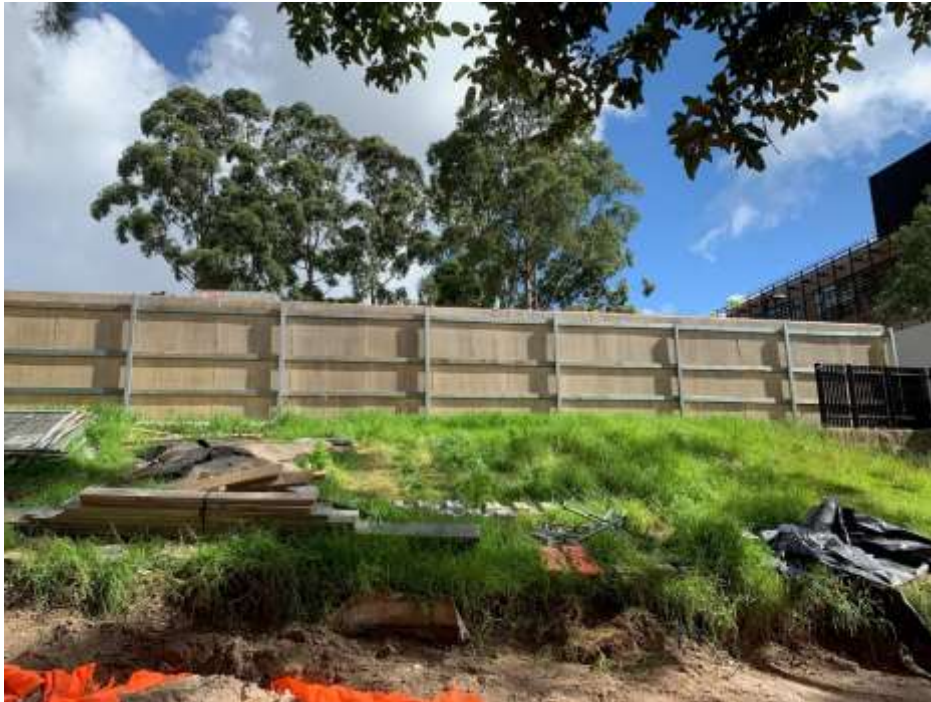
Photo 7: Acoustic hoarding between worksite and school playground
