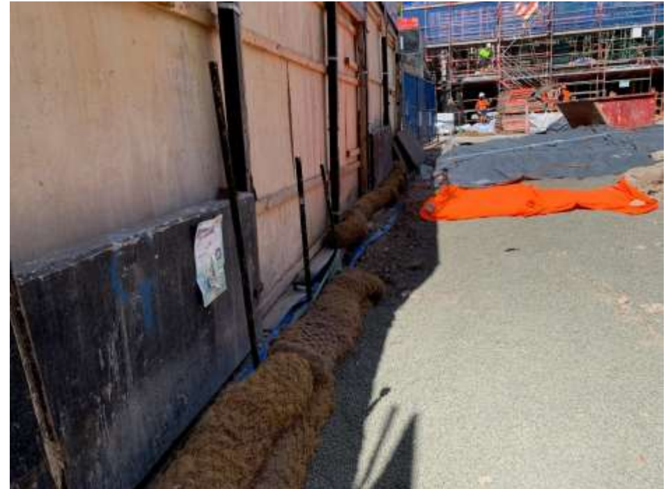
Photo 8: Sediment Controls
