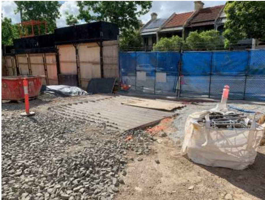
Photo 1: Stabilised Site Access and rumble grid
