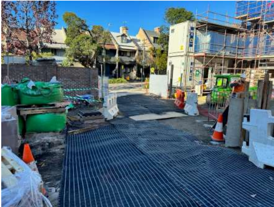
Photo 1: Stabilised Site Access
