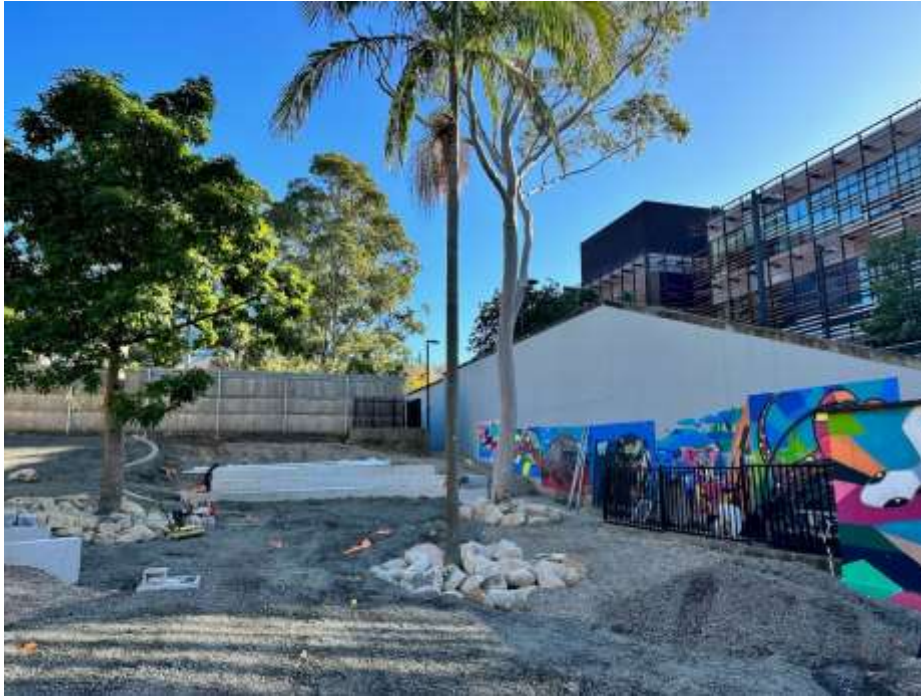
Photo 5: Final landscaping and completion work
