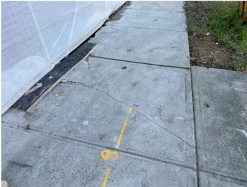
Photo 9: Cracked footpath
