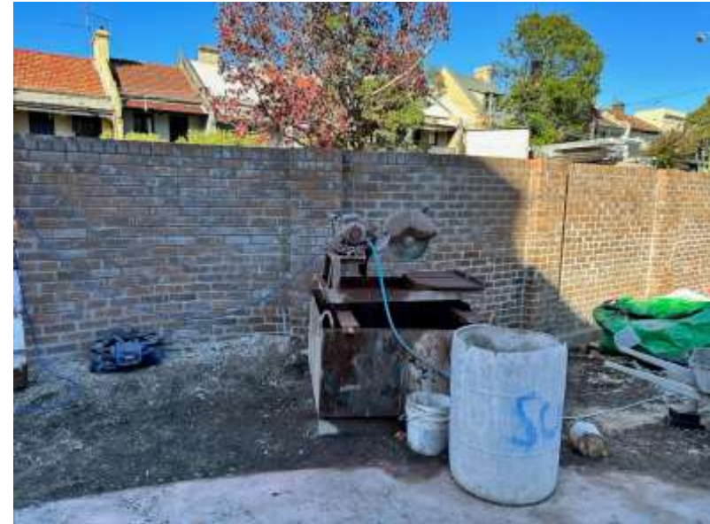
Photo 4: Sawcutter located behind masonry wall for noise attenuation
