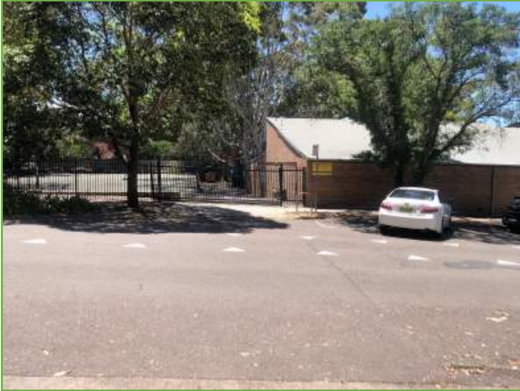
View looking east across Golden Grove Street towards the sites vehicular access driveway
