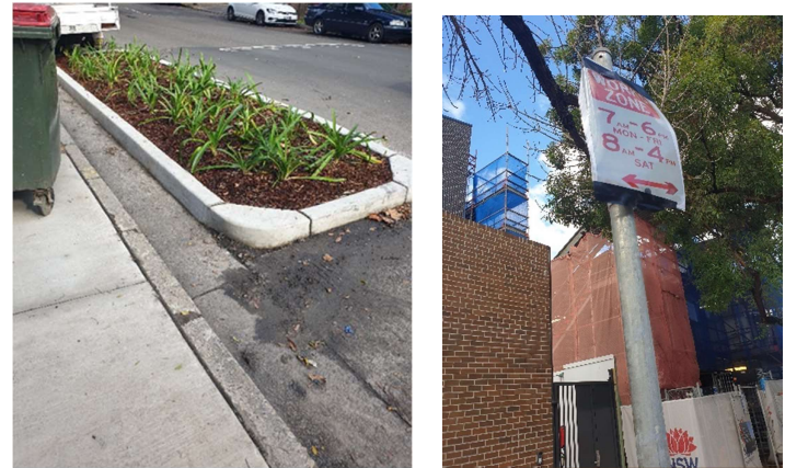
Photo 4: New public domain works island and temporary work zone sign over permanent sign
