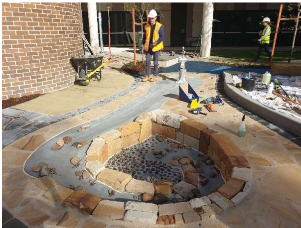
Photo 5: Finishing works within stage 1
