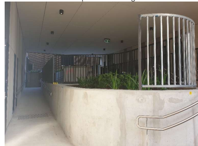
Photo 6: Landscaping within Stage 1
