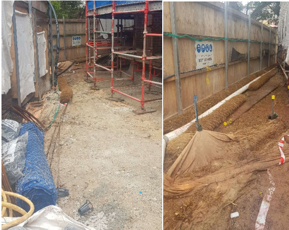
Photo 16: Coir logs observed on perimeter, geofabric shows water level
