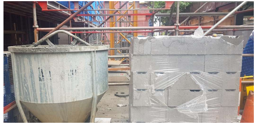
Photo 19: Material laydown area, concrete hopper used for pours
