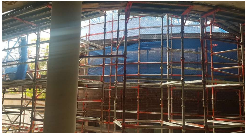
Photo 13: Building works observed, scaffold in place
