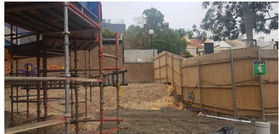
Photo 15: Behind new building, various levels and exposed soil
