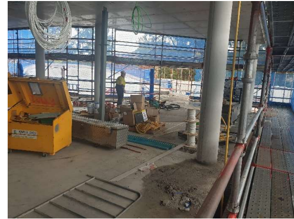
Photo 2: Fitout of buildings, some debris and waste visible
