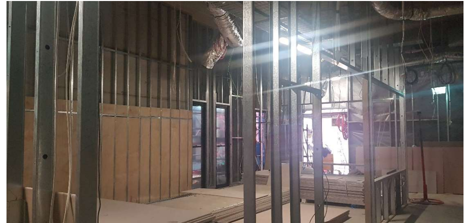
Photo 10: Fitout of buildings underway
