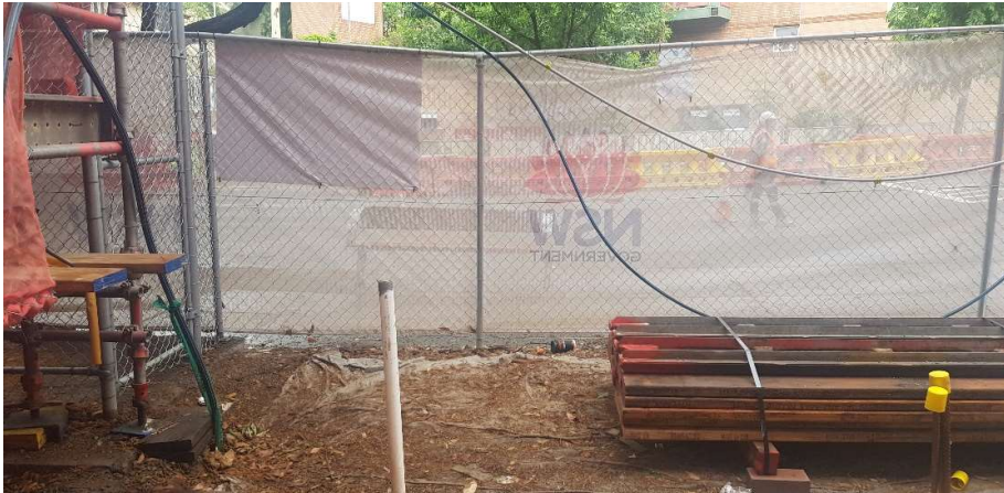
Photo 9: Inside front boundary of site, material layout area
