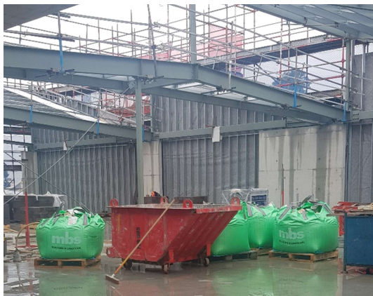
Photo 7: Bins and bulker bags stored in building. Site generally tidy
