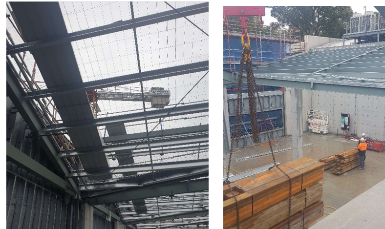
Photo 6: Roof construction in progress. Crane observed in use.
