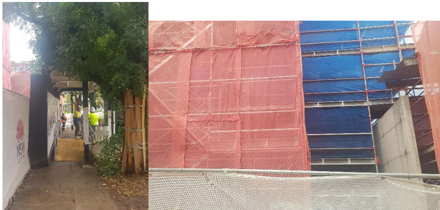
Photo 22: Approved hoarding, street work zone and building scaffold
