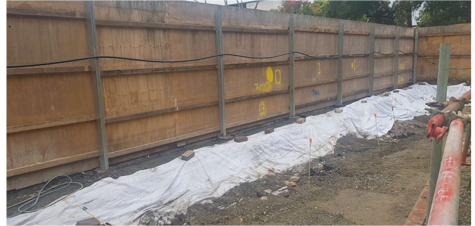
Photo 17: On perimeter to basketball court, geofabric berm in place
