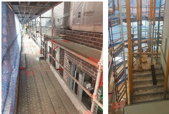
Photo 5: Brickwork and stairwell construction underway
