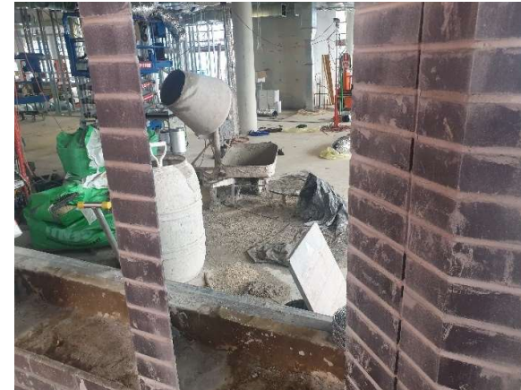
Photo 4: Mortar mixing for brickwork. Tub nearby for tool washout.
