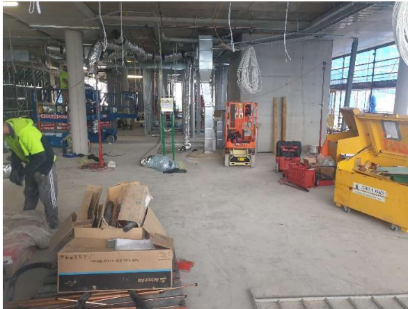
Photo 1: Fitout of buildings, site works area generally tidy
