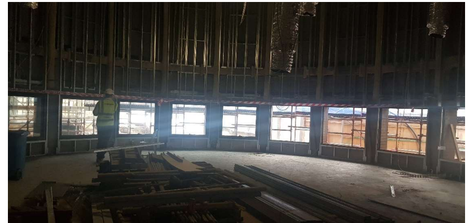
Photo 12: Inside proposed library, fitout underway
