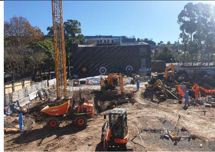
Figure 6 – View of site works, noting covered stockpile and access tracks
