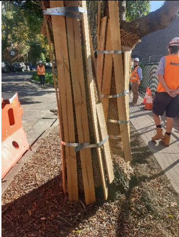
Figure 5 – Tree Protection Zones and controls, including near hoarding
