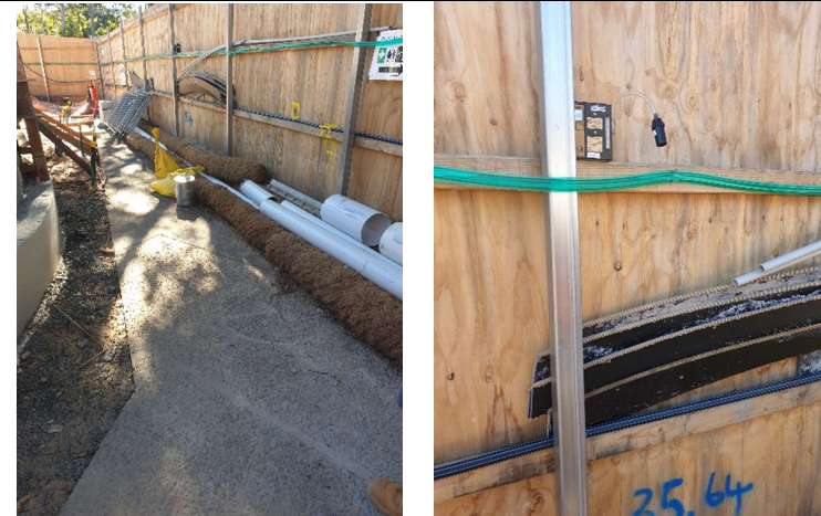
Figure 12 – Internal hoarding, with coir logs, soaker hose and air monitoring
