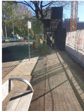
Figure 5 – Tree Protection Zones and controls, including near hoarding
