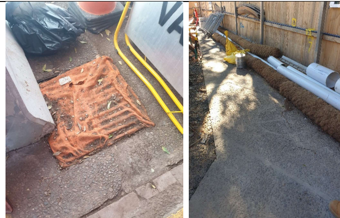
Figure 4 – Geofabric filter over drains and coir logs on perimeter
