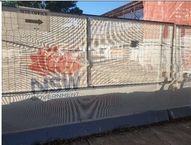
Figure 1 – Banner mesh installed on the perimeter of Project boundary
