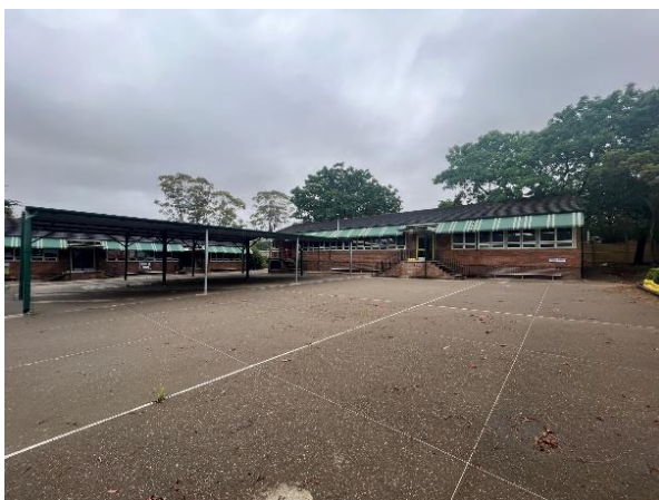
Figure 5 – Existing Building A
