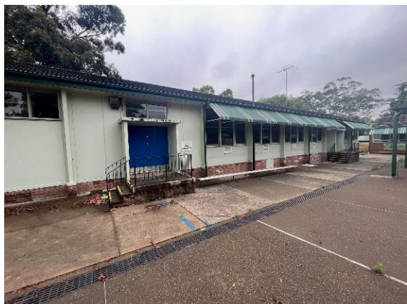
Figure 6 – Existing Building D
