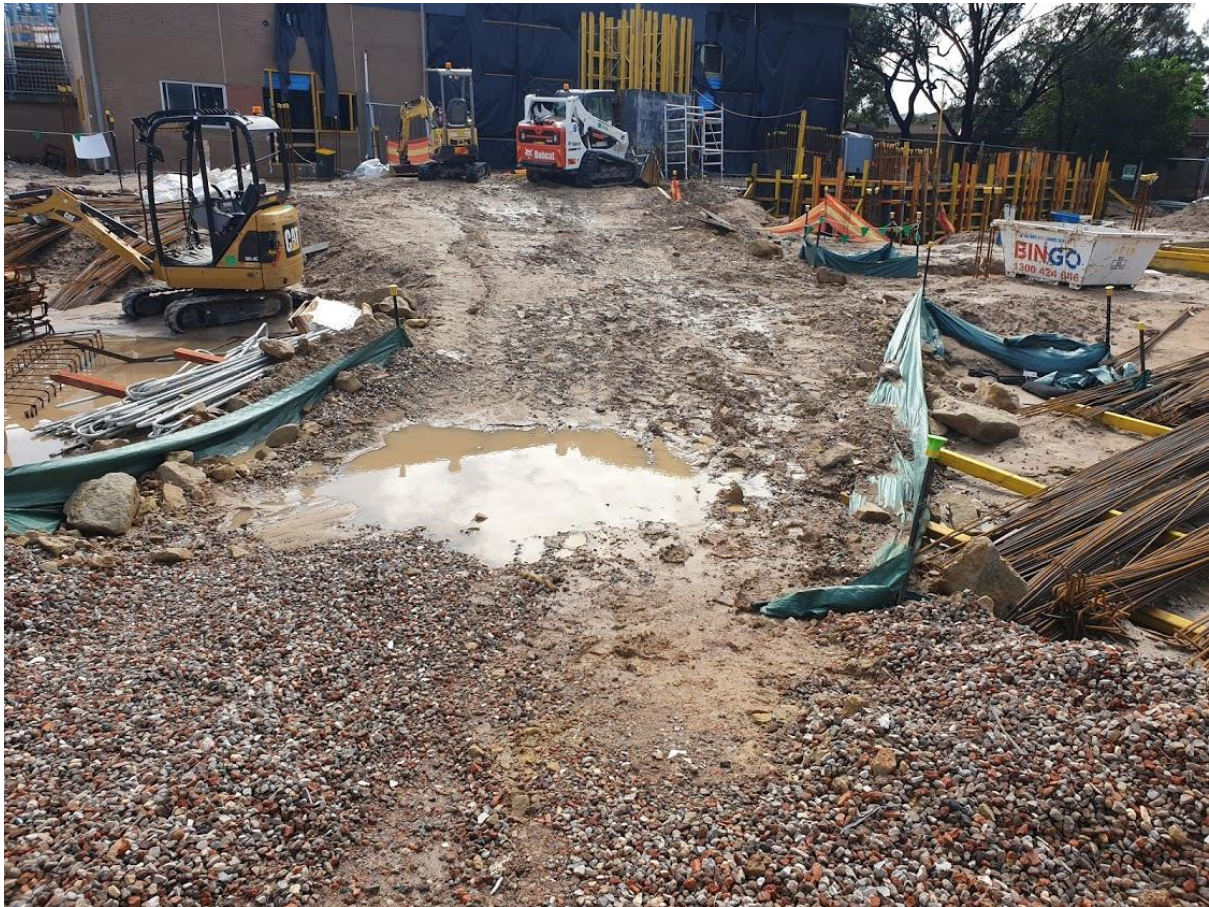
Plate 10 – Silt fence in drainage line following heavy rain event (maintenance planned once site dries out)
