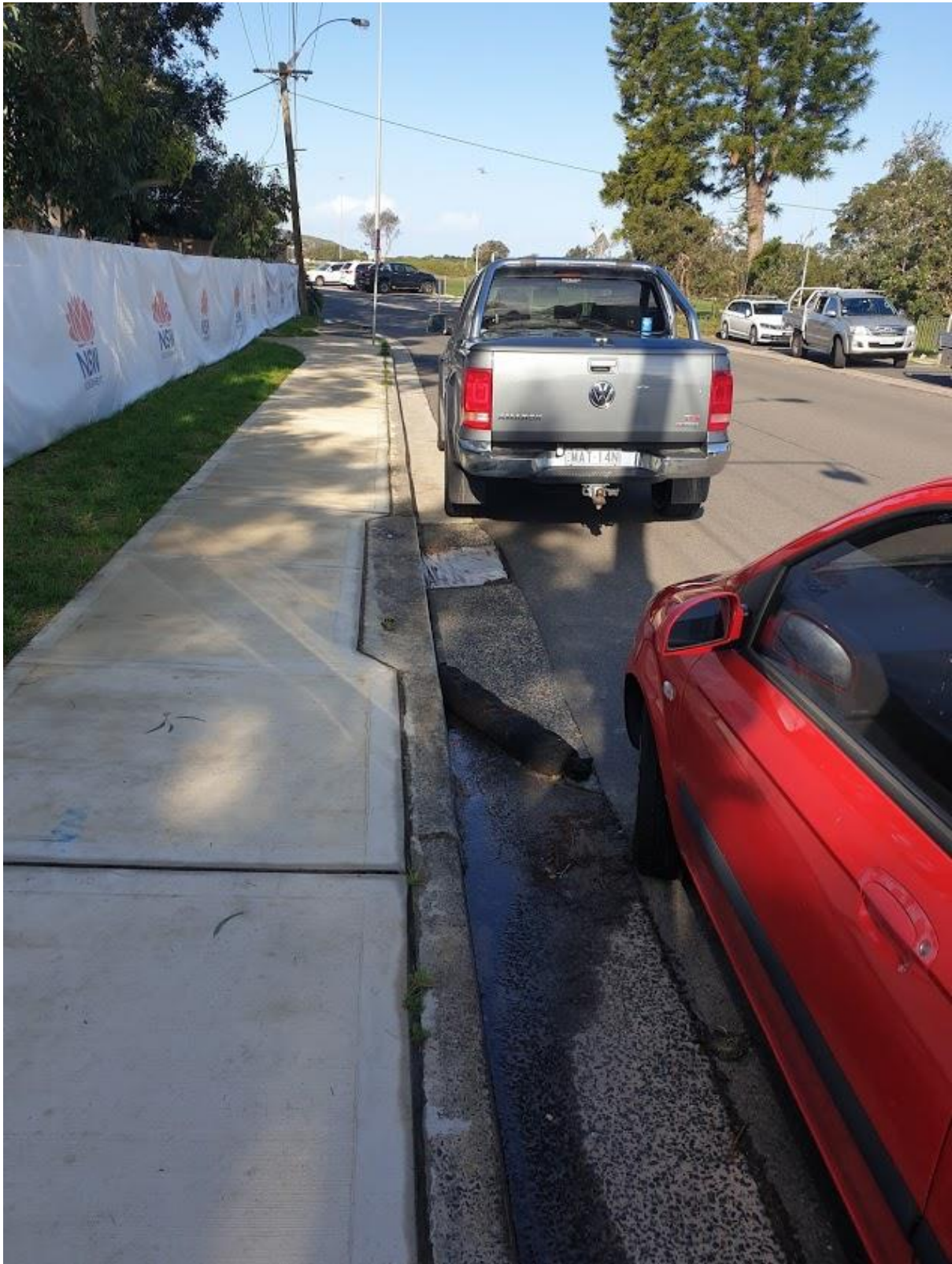
Plate 15 – Sediment socks and geofabric covered inlet in stormwater drainage system outside site
