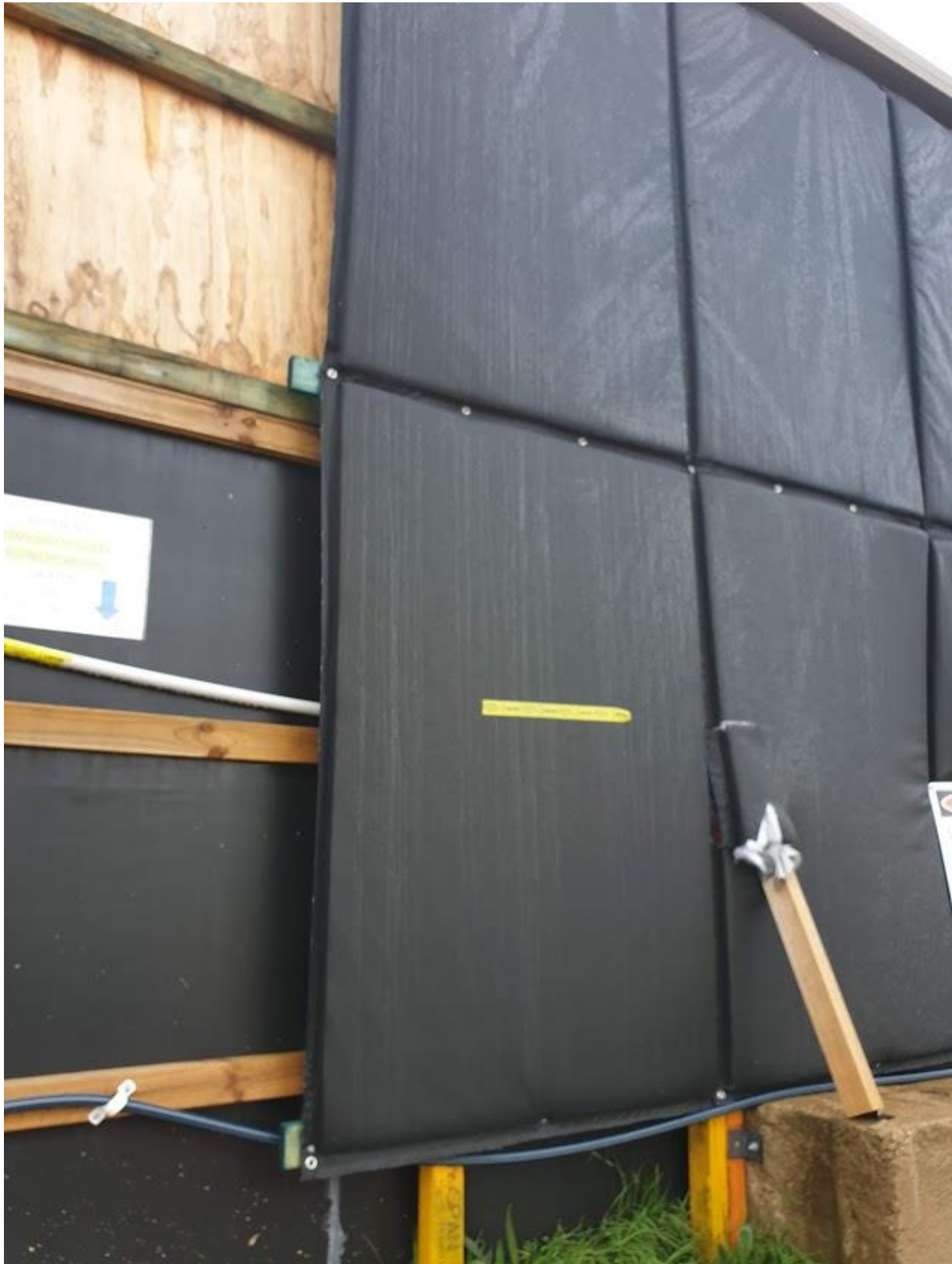
Plate 7 – Acoustic blanket placed over site hoarding
