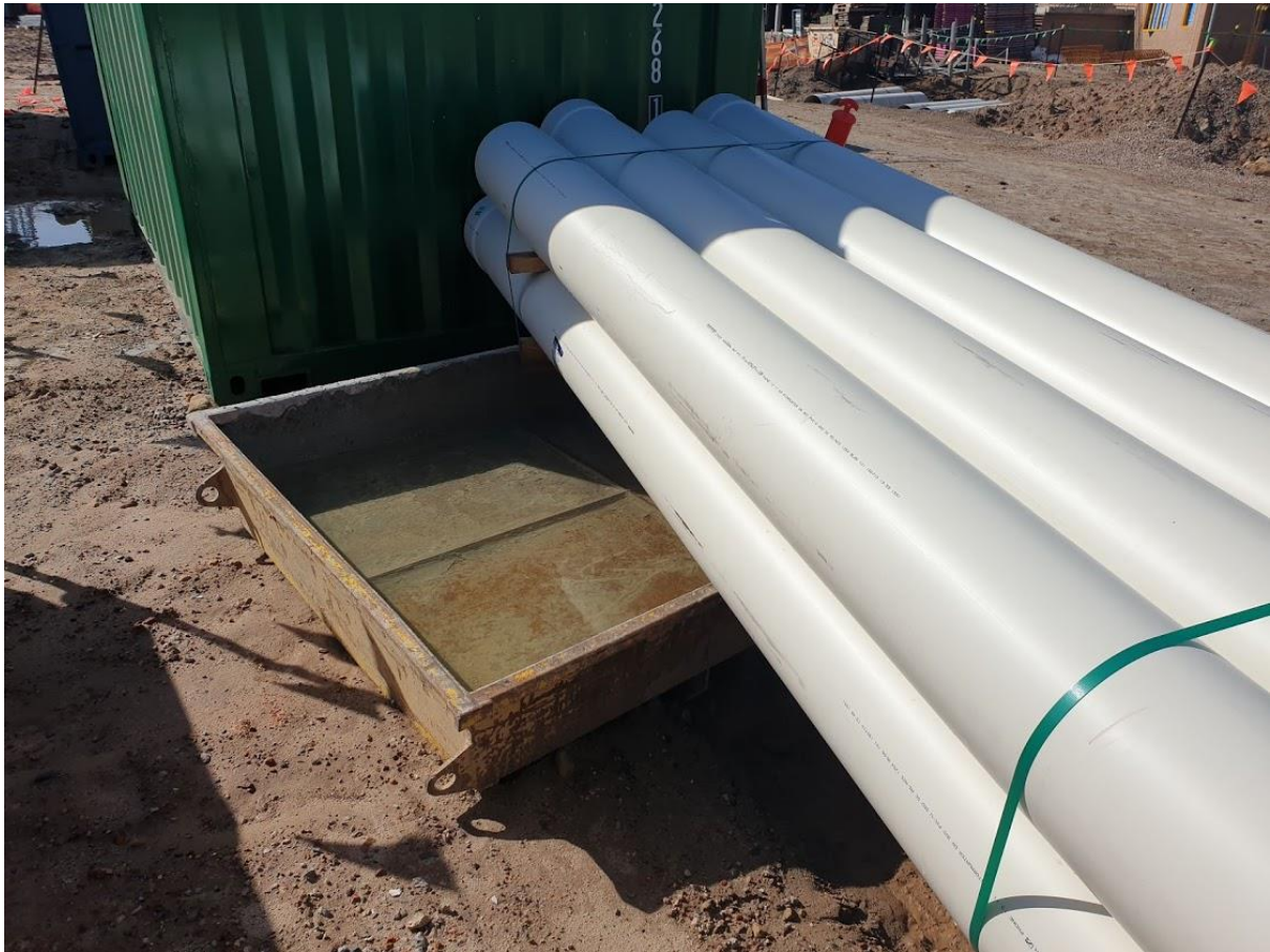
Plate 16 – Concrete washout tray
