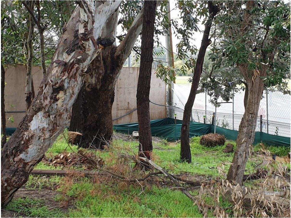
Plate 13 – Silt fence in lowest corner of site
