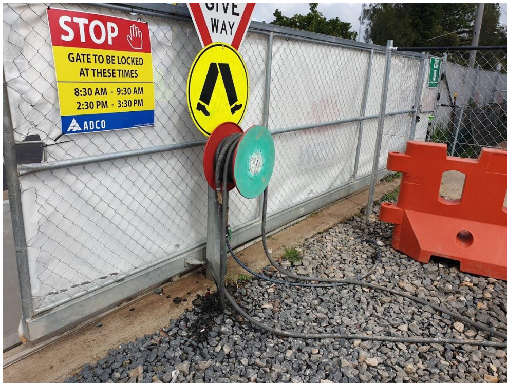
Plate 1A – Site entrance sliding gate with high pressure hose for vehicle wash down
