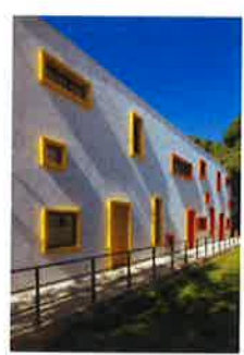
AW2 COLOURED CLADDING OVER FRAME
